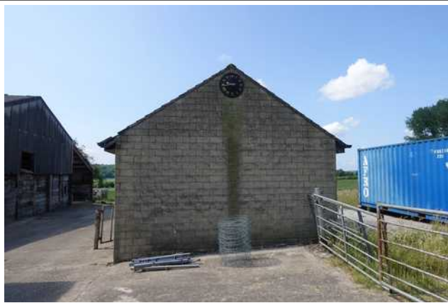
Outbuilding 1 North Gable End
