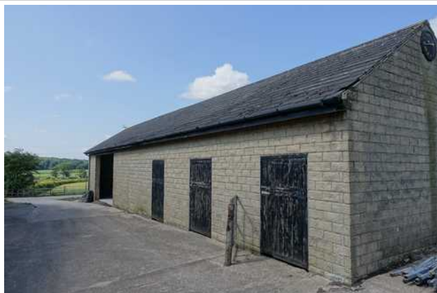
Outbuilding 1 South East Facade
