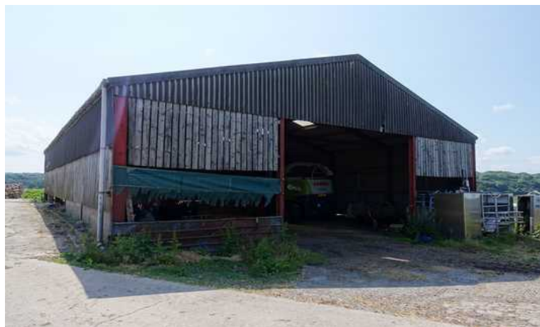
Outbuilding 3 Northern Gable
