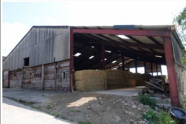
Outbuilding 2 Northern Gable
