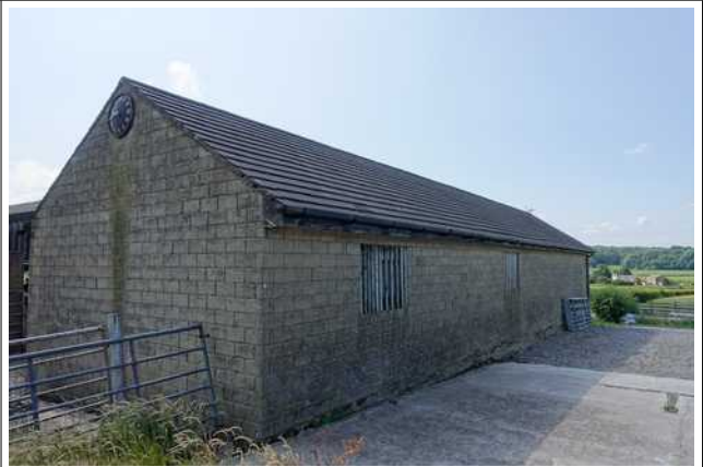
Outbuilding 1 North West Facade
