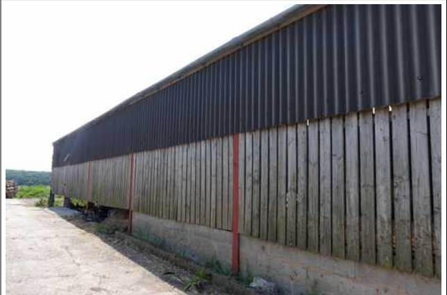
Outbuilding 2 Western Facade
