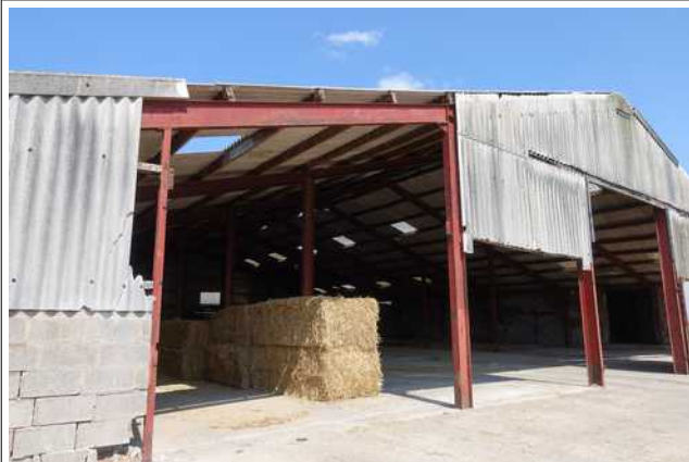
Outbuilding 2 Southern Gable
