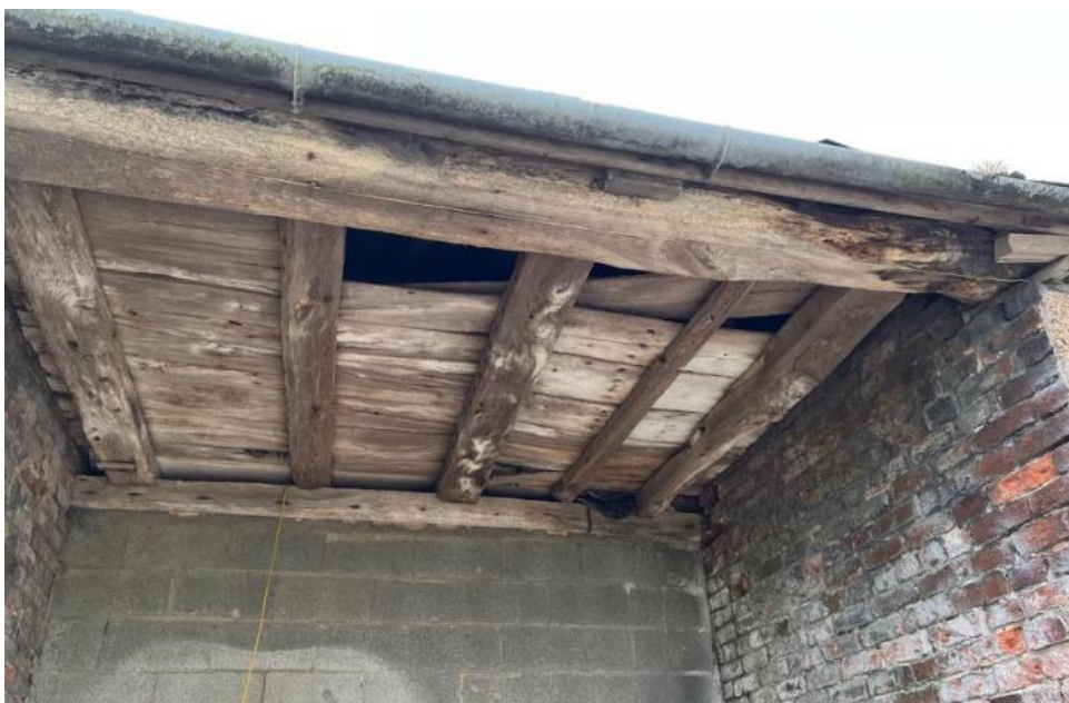
Figure 5) Northern cart entry porch with brick cheeks and wooden loft above
