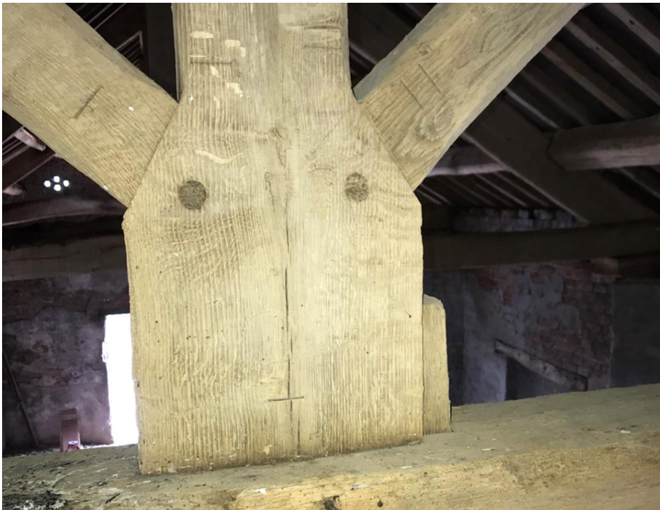
Figure 15) Jowelled king post with pegged joints and carpenter's marks
