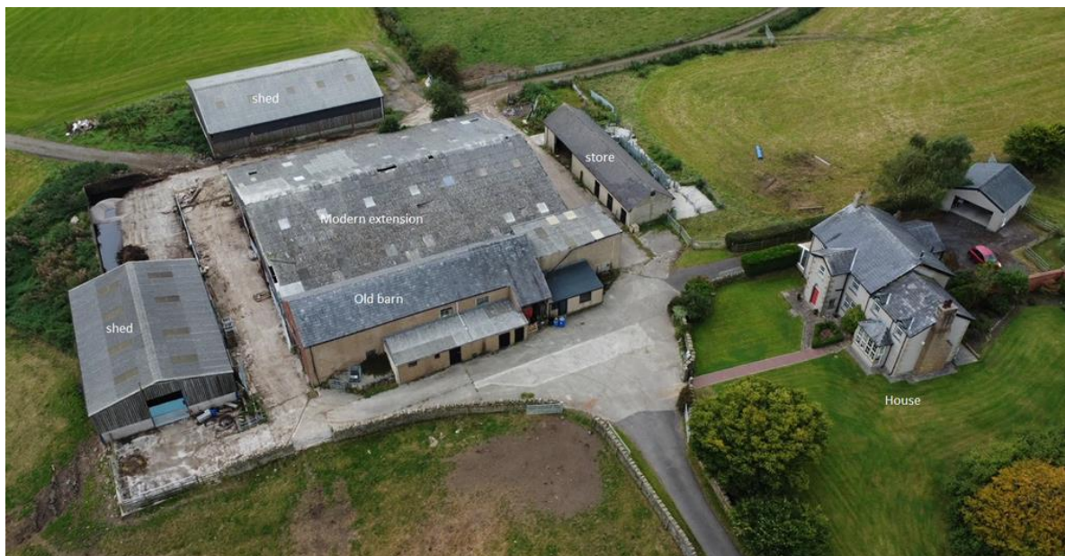
Figure 2) Aerial view of the barn and adjacent buildings (viewed from the north)
