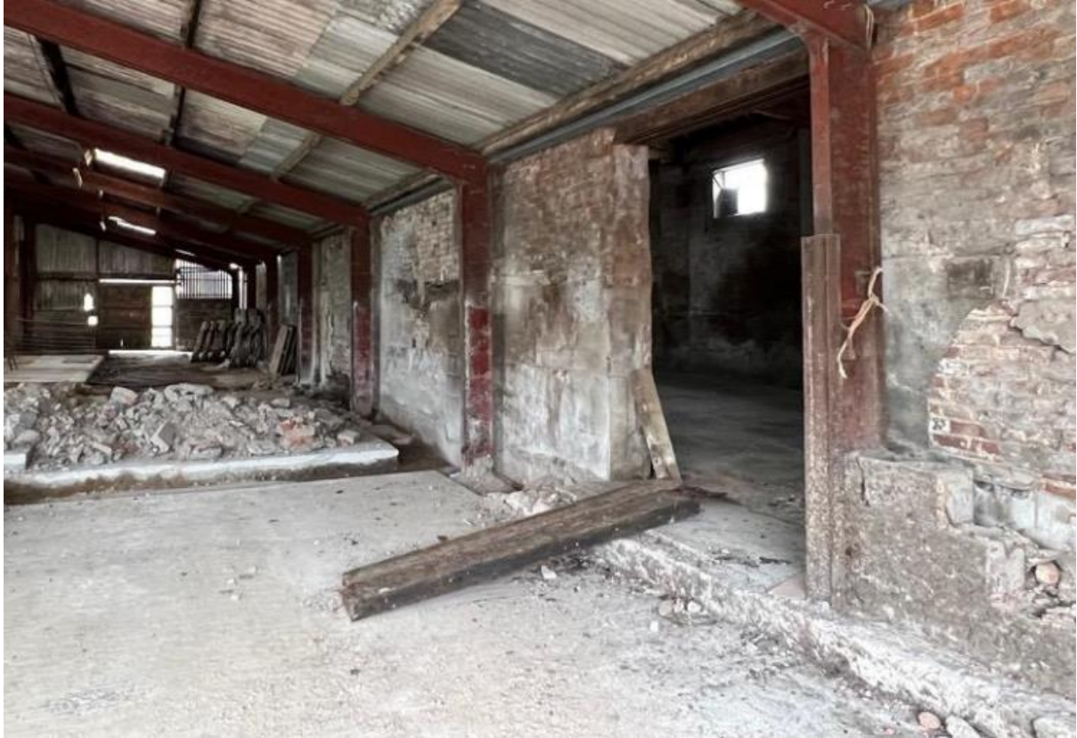
Figure 10) Long southern elevation enclosed within the adjoining portal frame shed extension
