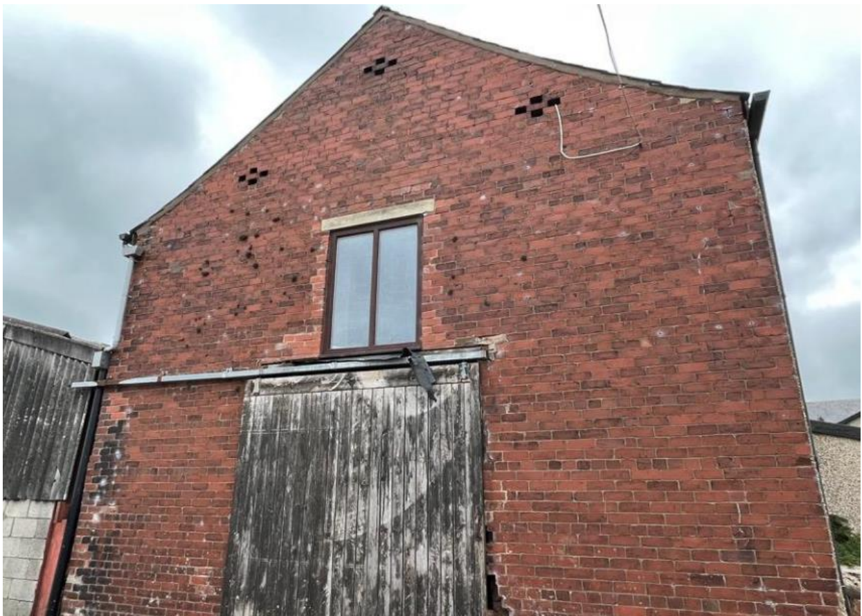
Figure 7) Rebuilt/replacement eastern gable with upper breather vents, inserted loft window and sliding door
