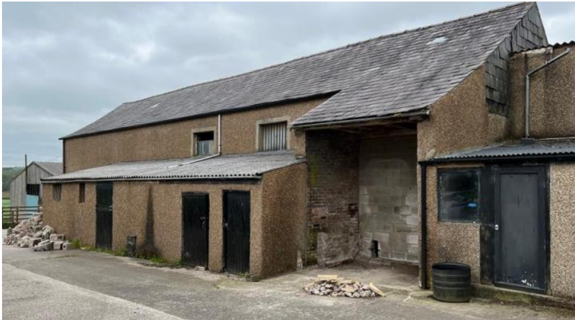
Figure 4) Long northern elevation with cart entry porch, two upper pitching holes above lean-to store additions
