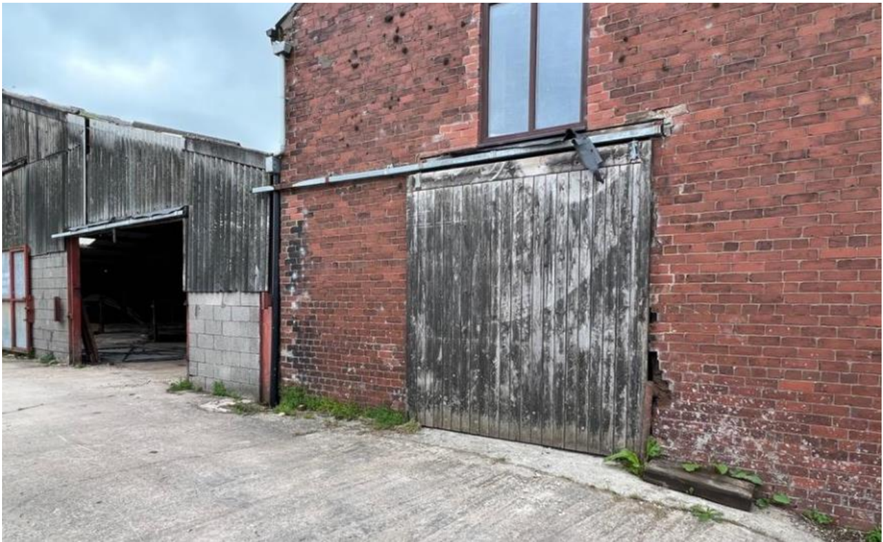
Figure 14) Eastern gable of the barn showing portal frame addition to the left (south)
