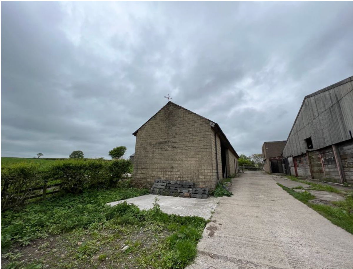
Photo 2 – South West Gable
