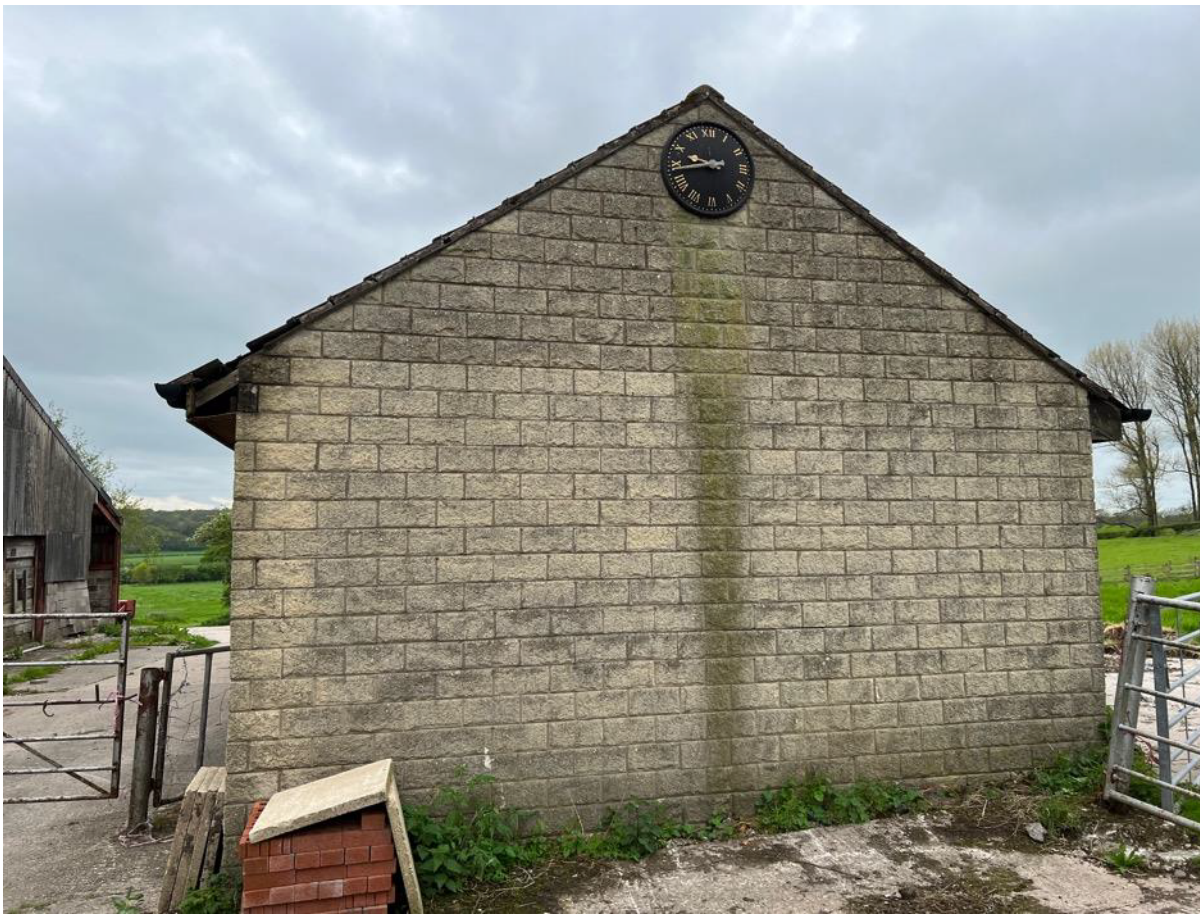
Photo 11 – North East Gable
