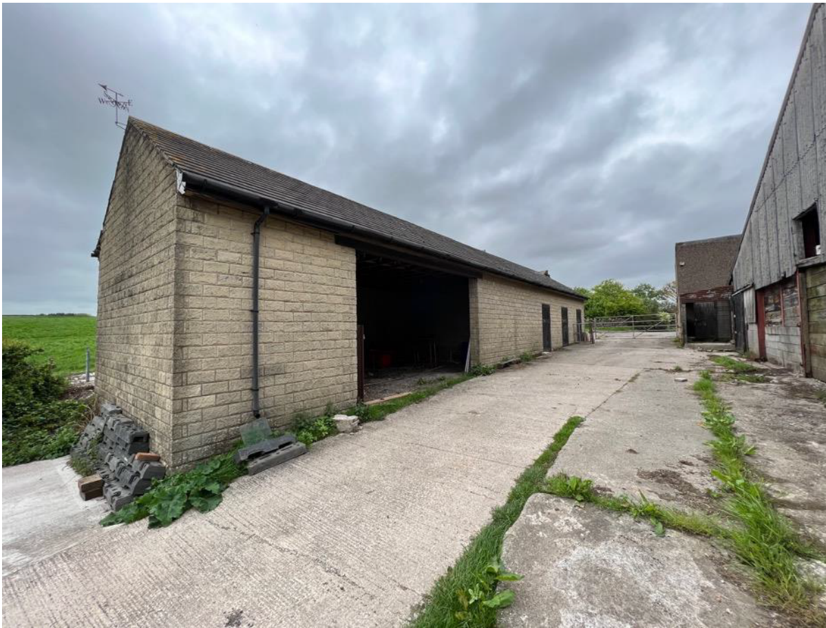
Photo 1 – South East Elevation
