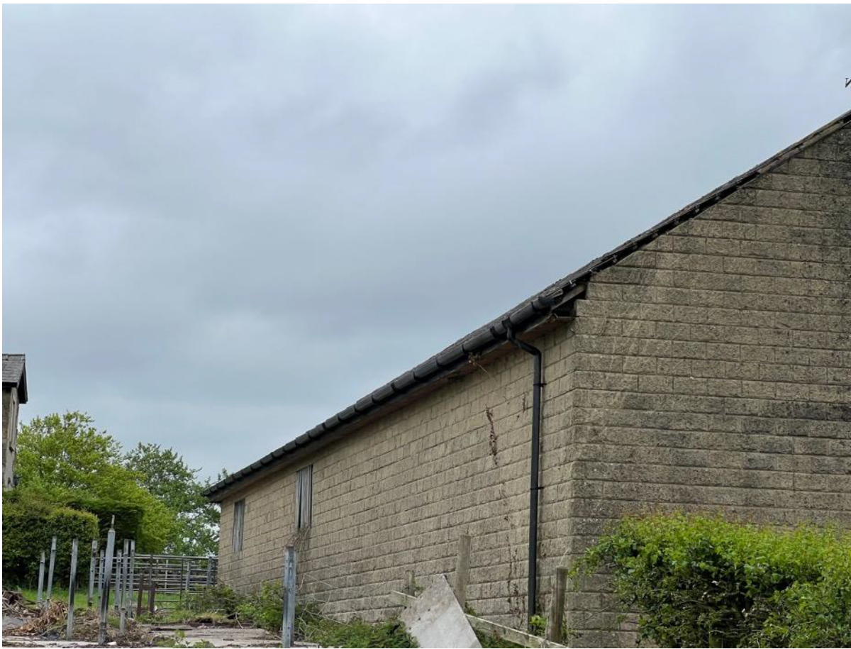
Photo 3- North West Elevation
