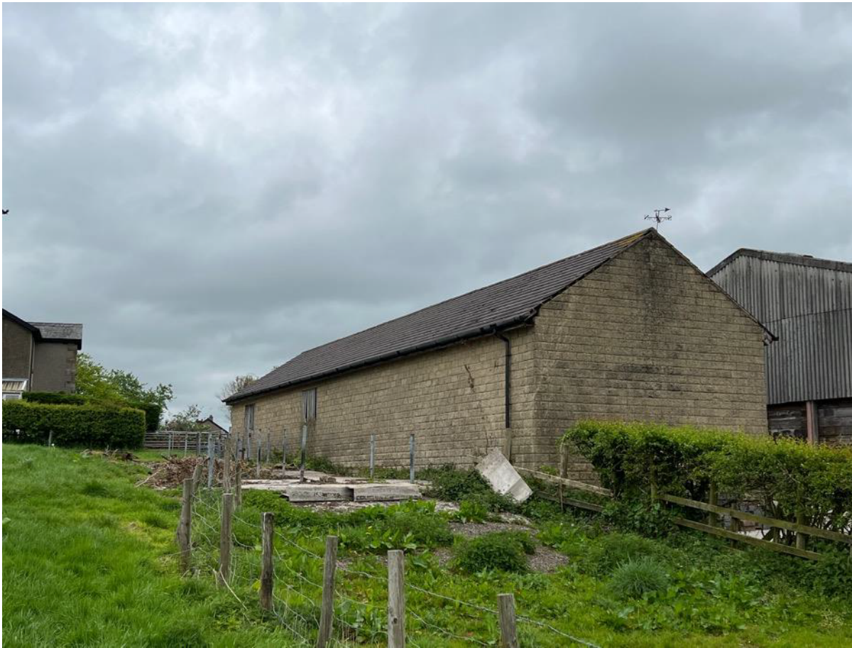
Photo 4 – North West Elevation
