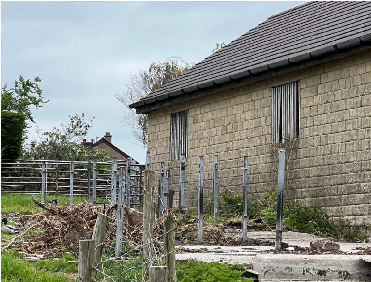
Photo 6 – North West Elevation
