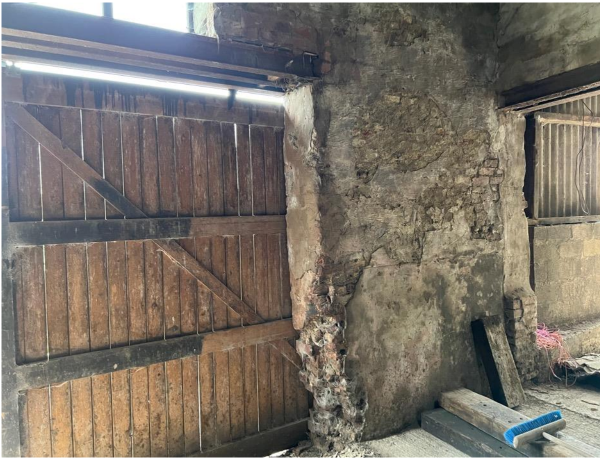
Photo 45 – internal main barn
