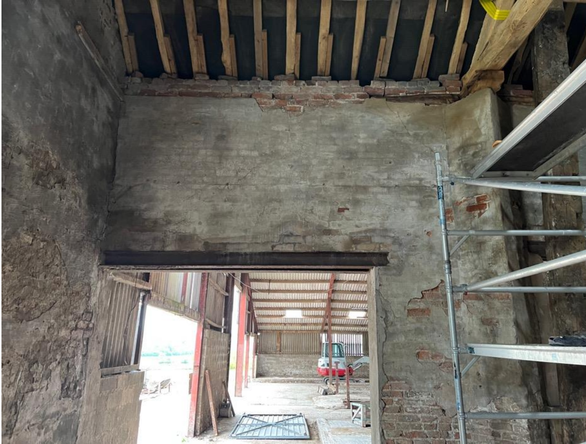
Photo 44 - Internal – main barn
