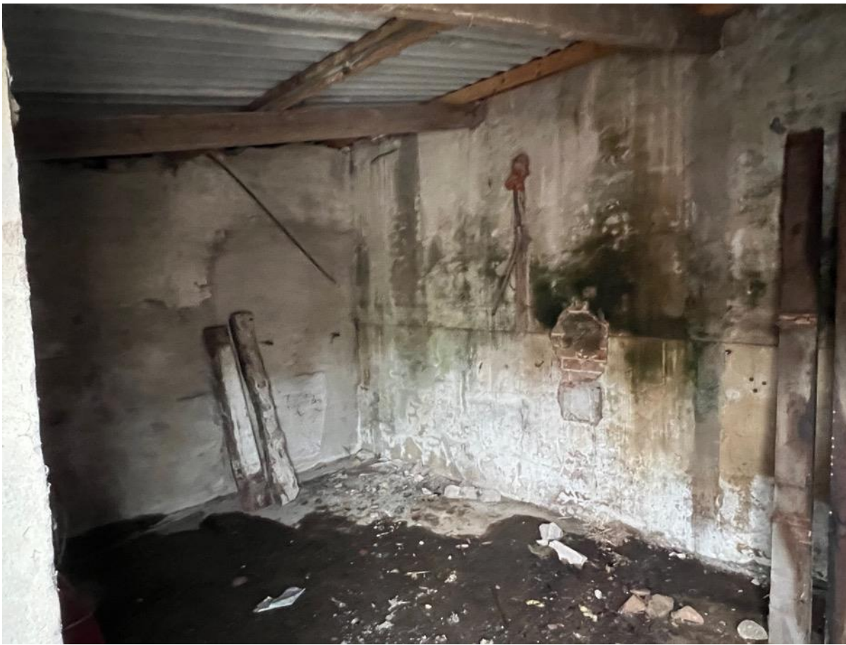
Photo 33 – Internal – extensions to north east elevation
