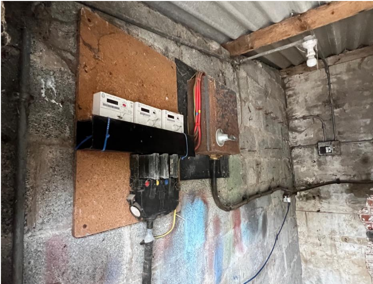
Photo 36 - Internal – extensions to north east elevation
