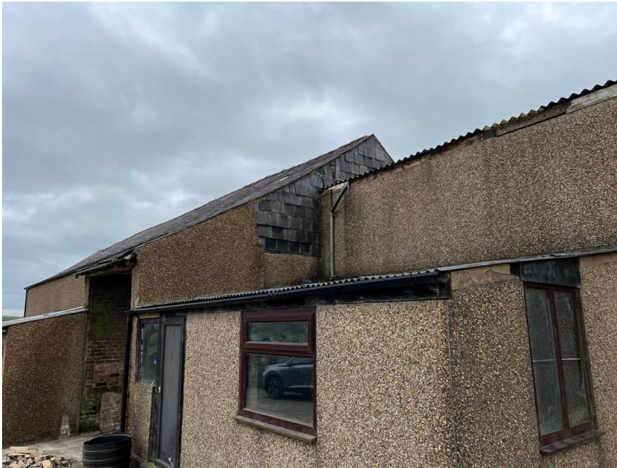
Photo 4 – North East Elevation
