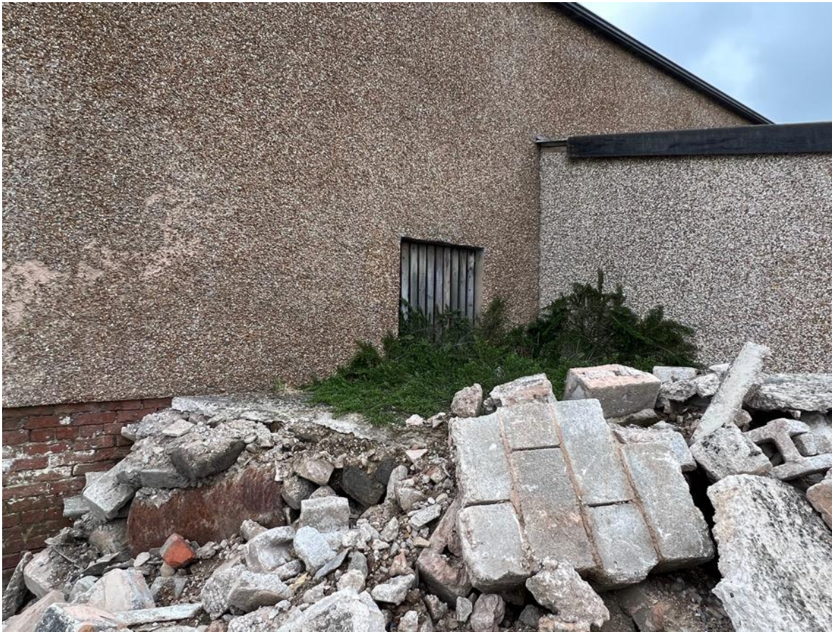
Photo 16 - North East Elevation
