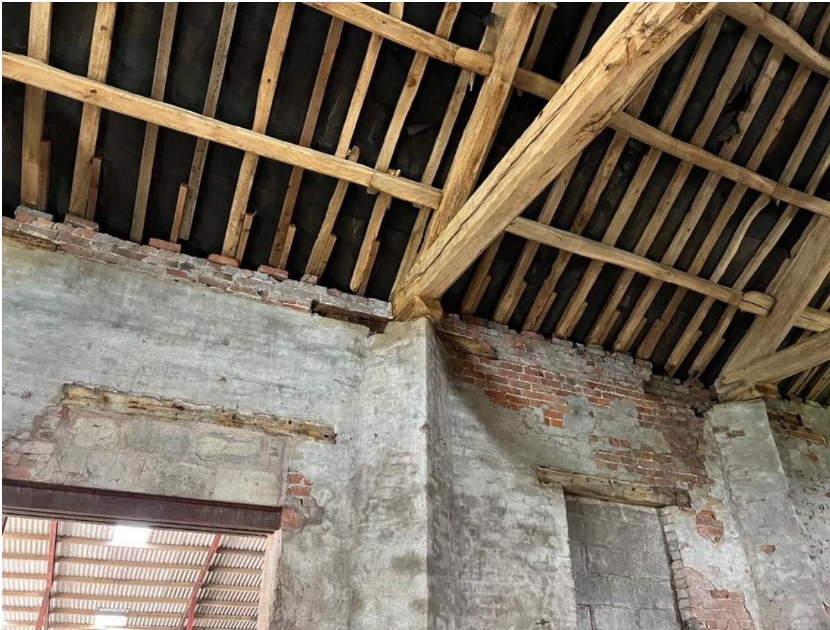
Photo 50 - Internal – main barn
