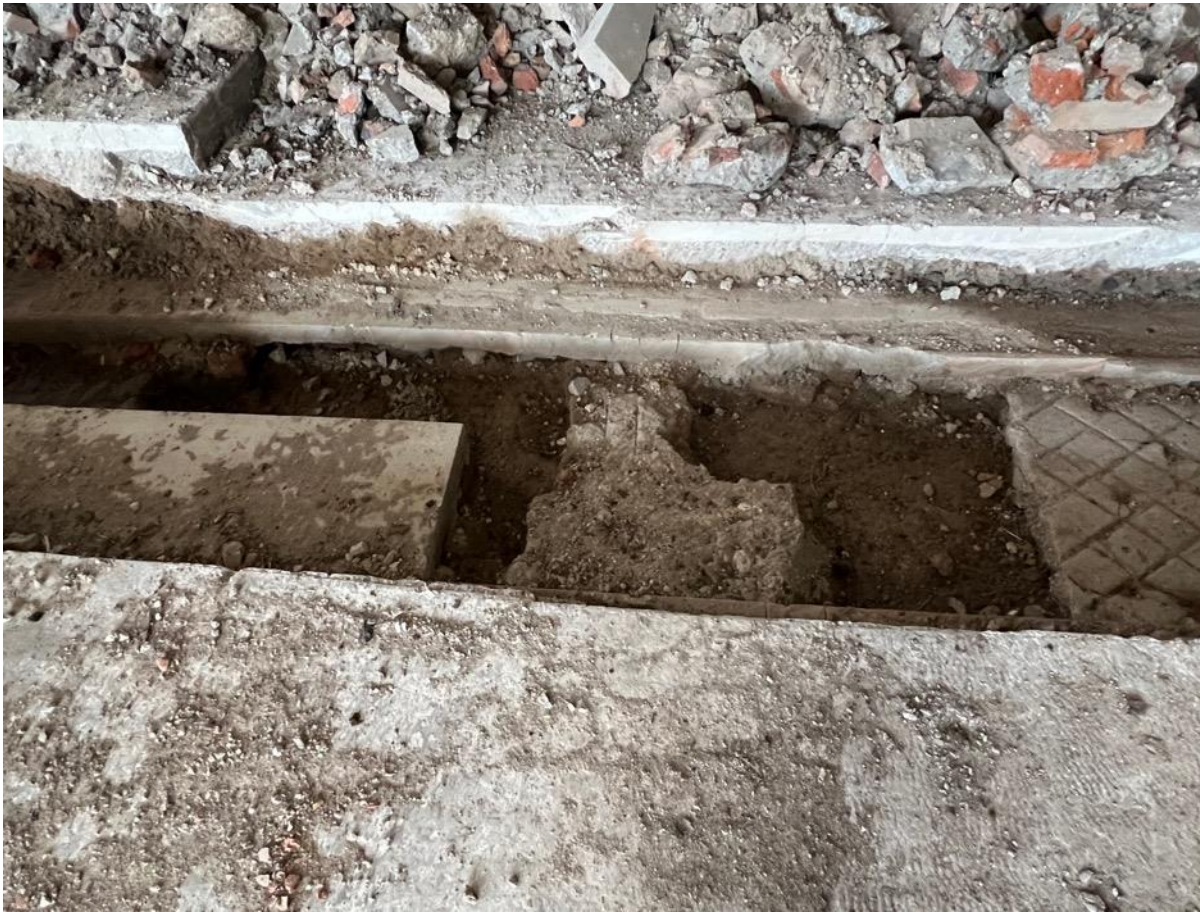
Photo 28 - South West Elevation – excavations to reveal former lean-to section
