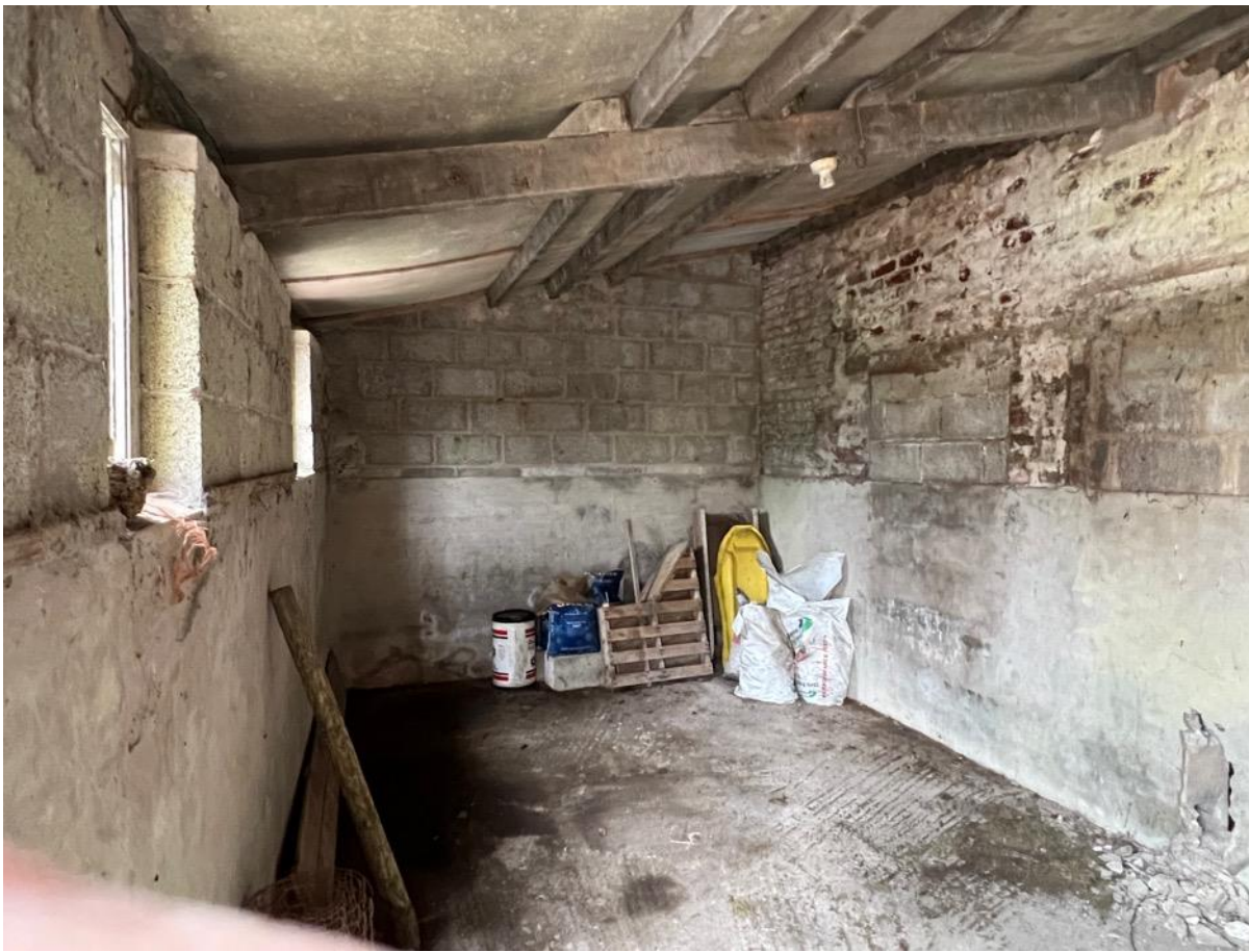
Photo 37 - Internal – extensions to north east elevation
