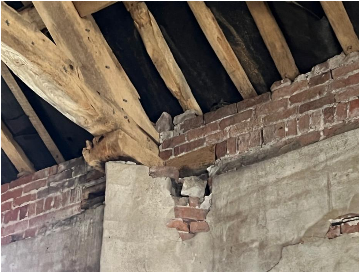
Photo 52 - Internal – main barn
