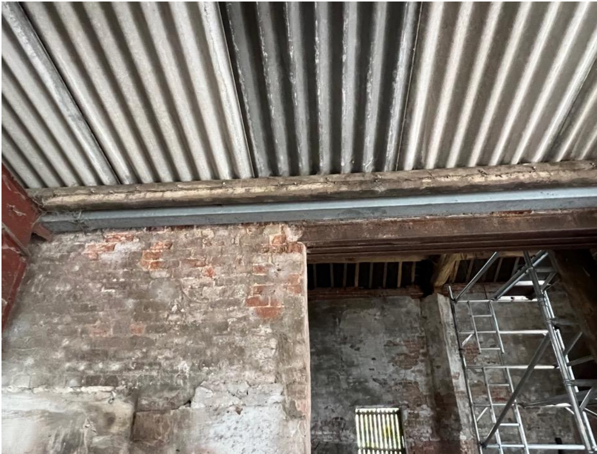
Photo 26 - South West Elevation
