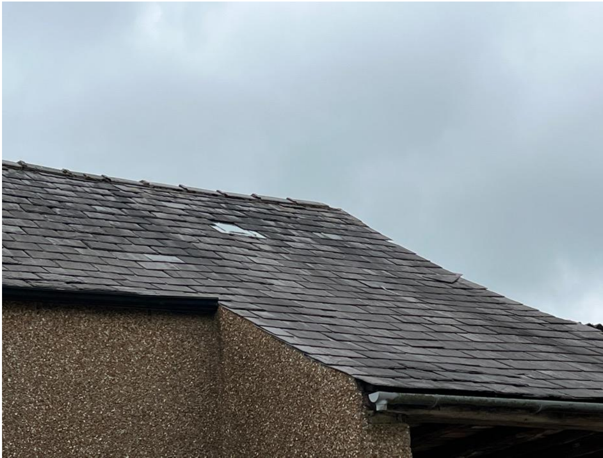
Photo 10 – North East Elevation Roof
