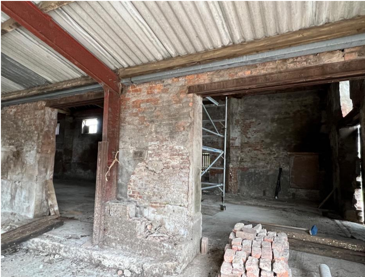
Photo 22 – South West Elevation
