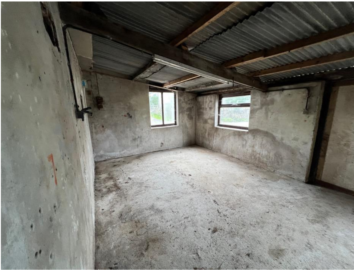
Photo 61 – extension – room to north east elevation
