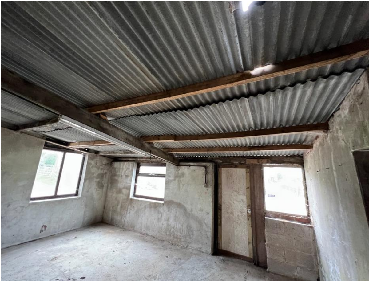
Photo 62 - extension – room to north east elevation
