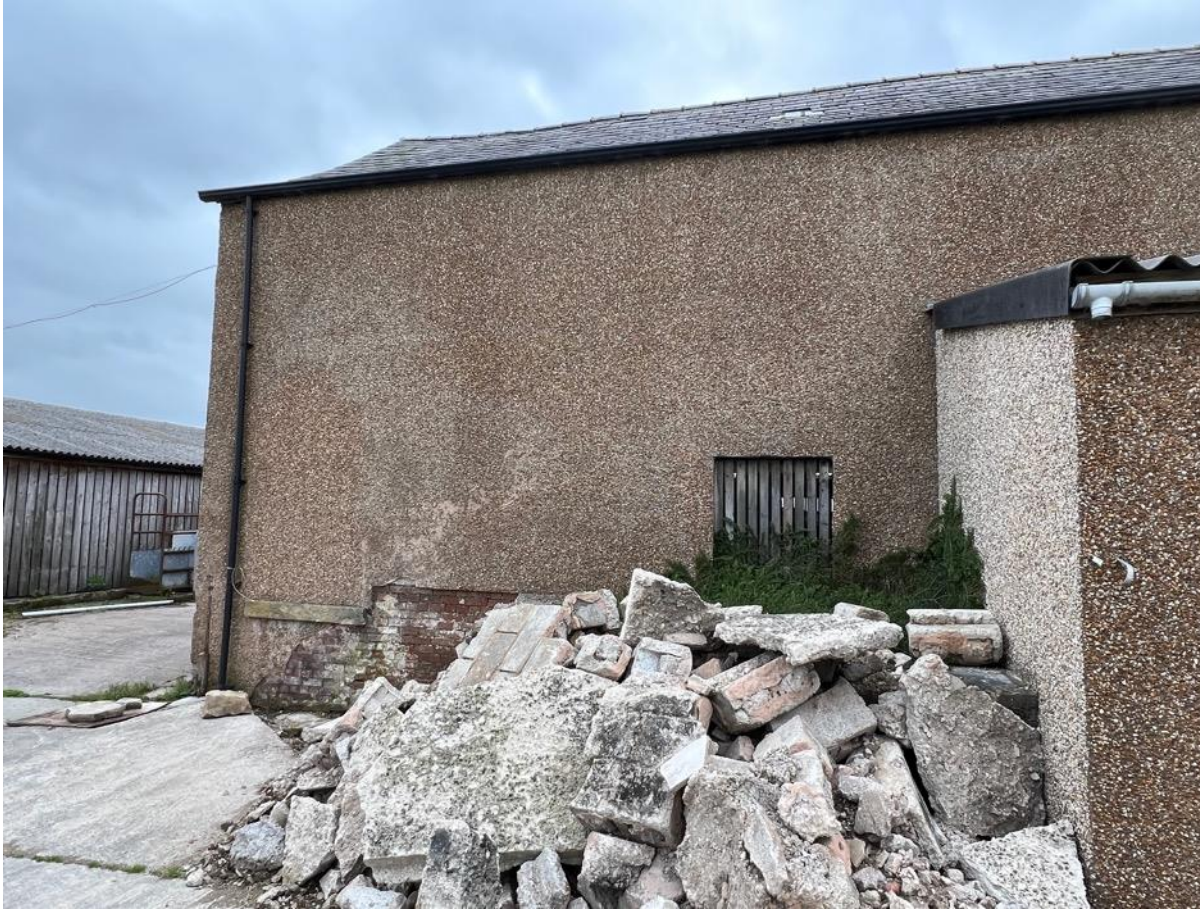
Photo 14 - North East Elevation
