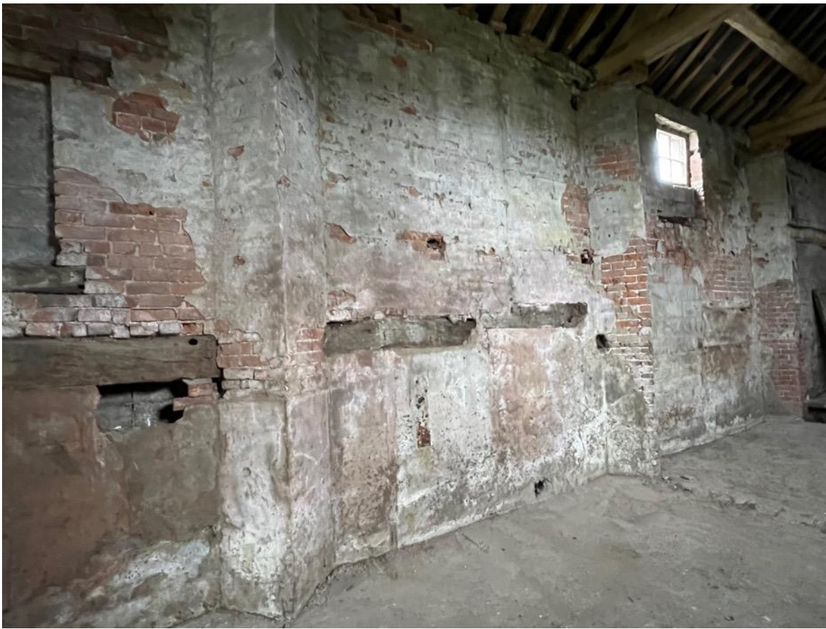
Photo 55 - Internal – main barn
