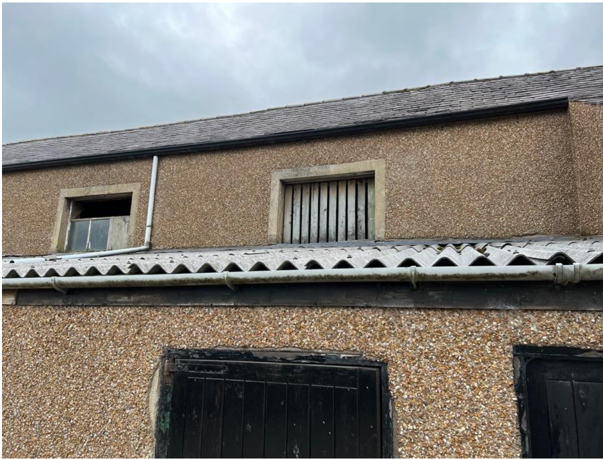
Photo 9 – North East Elevation – Extensions along elevation
