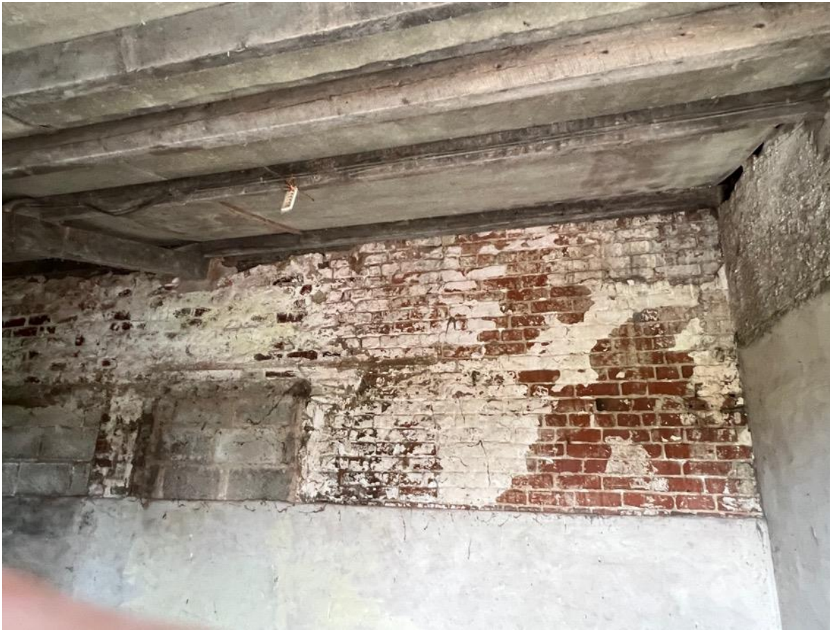
Photo 38 - Internal – extensions to north east elevation
