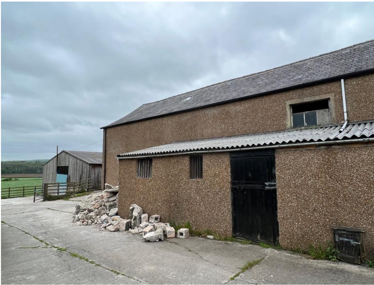
Photo 13 – North East Elevation
