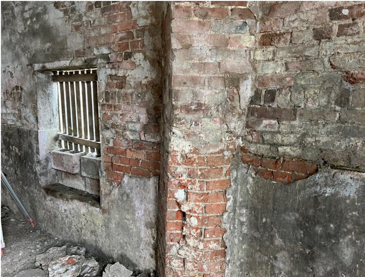
Photo 46 - Internal – main barn
