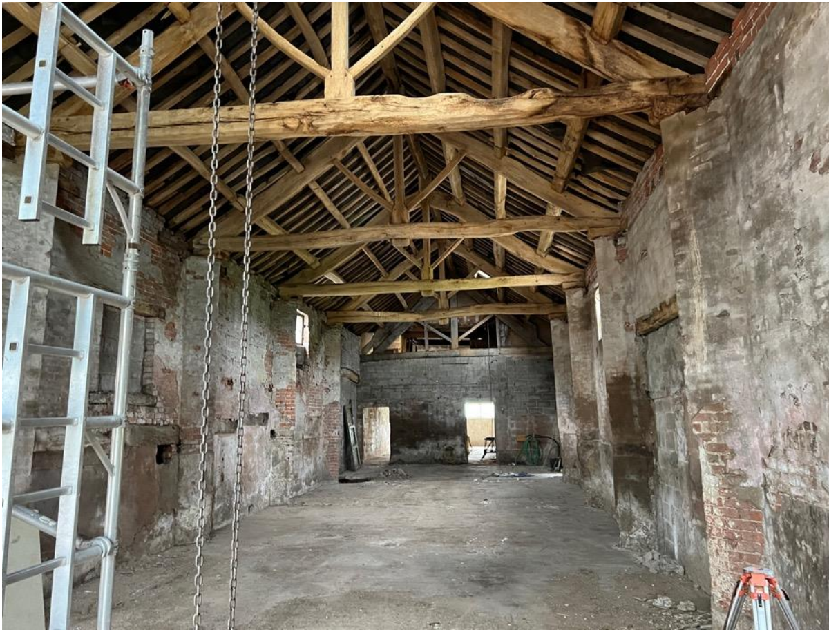
Photo 40 – Internal – main barn
