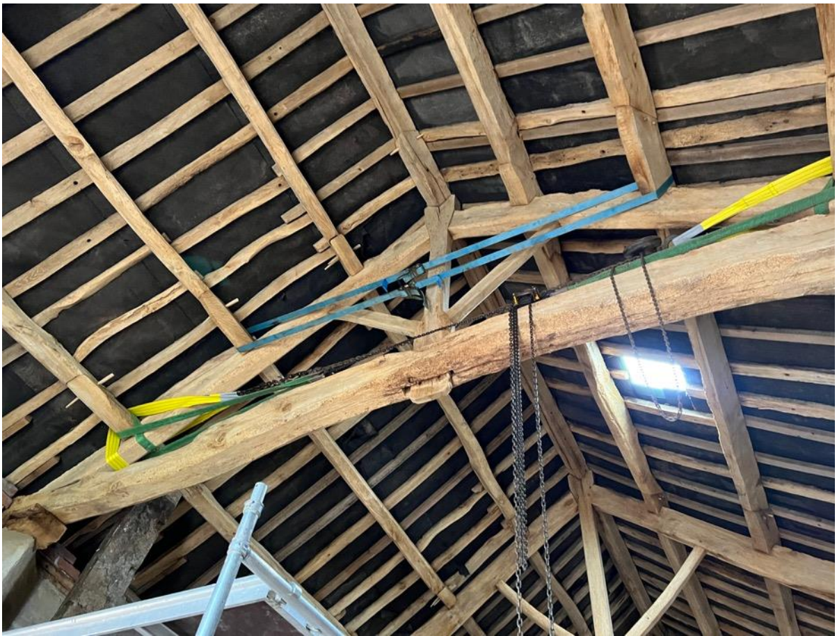
Photo 42 - Internal – main barn
