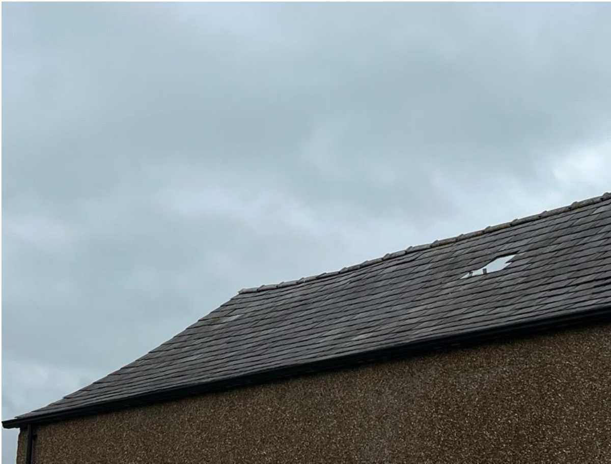
Photo 12 - North East Elevation Roof
