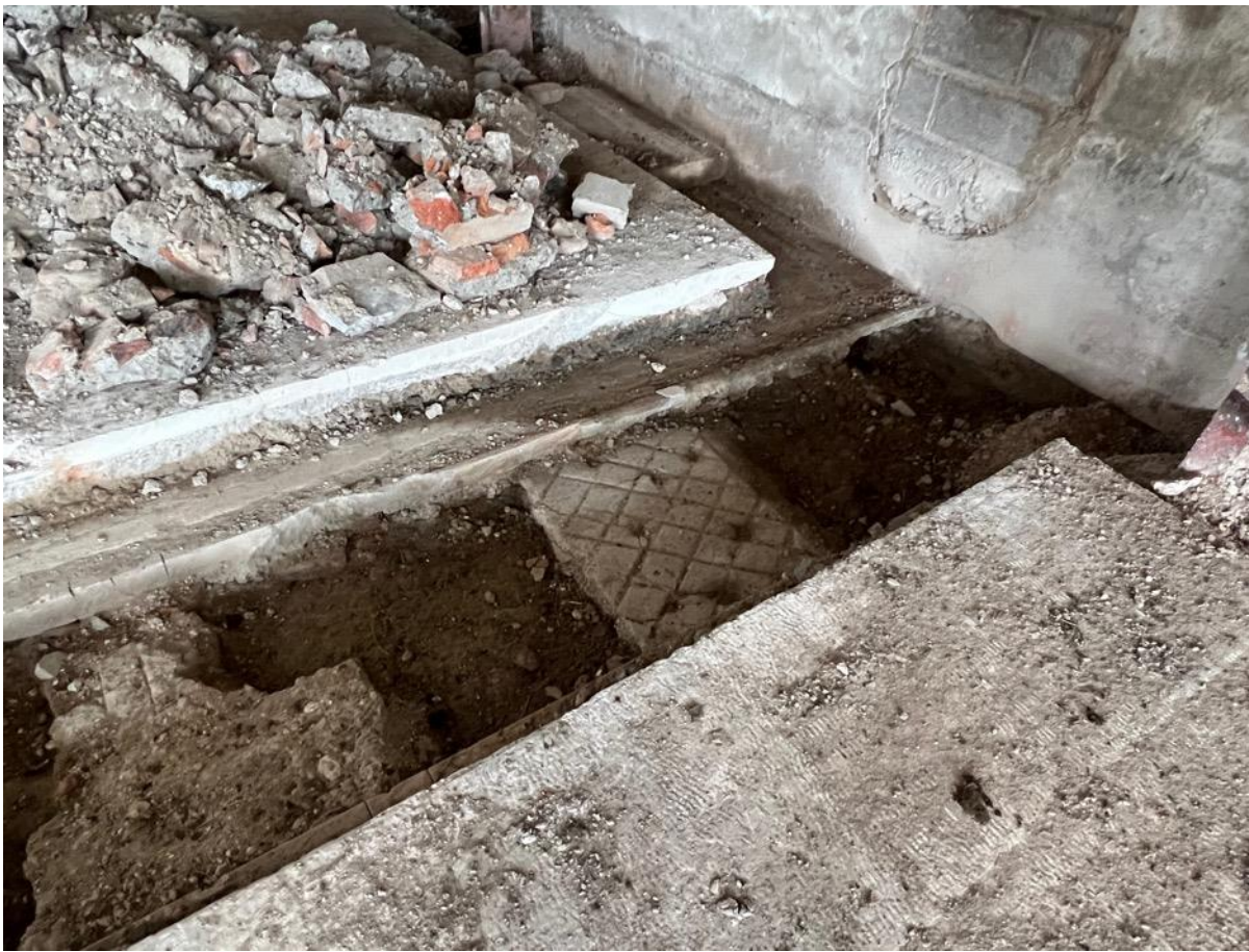
Photo 27 - South West Elevation – excavations to reveal former lean-to section
