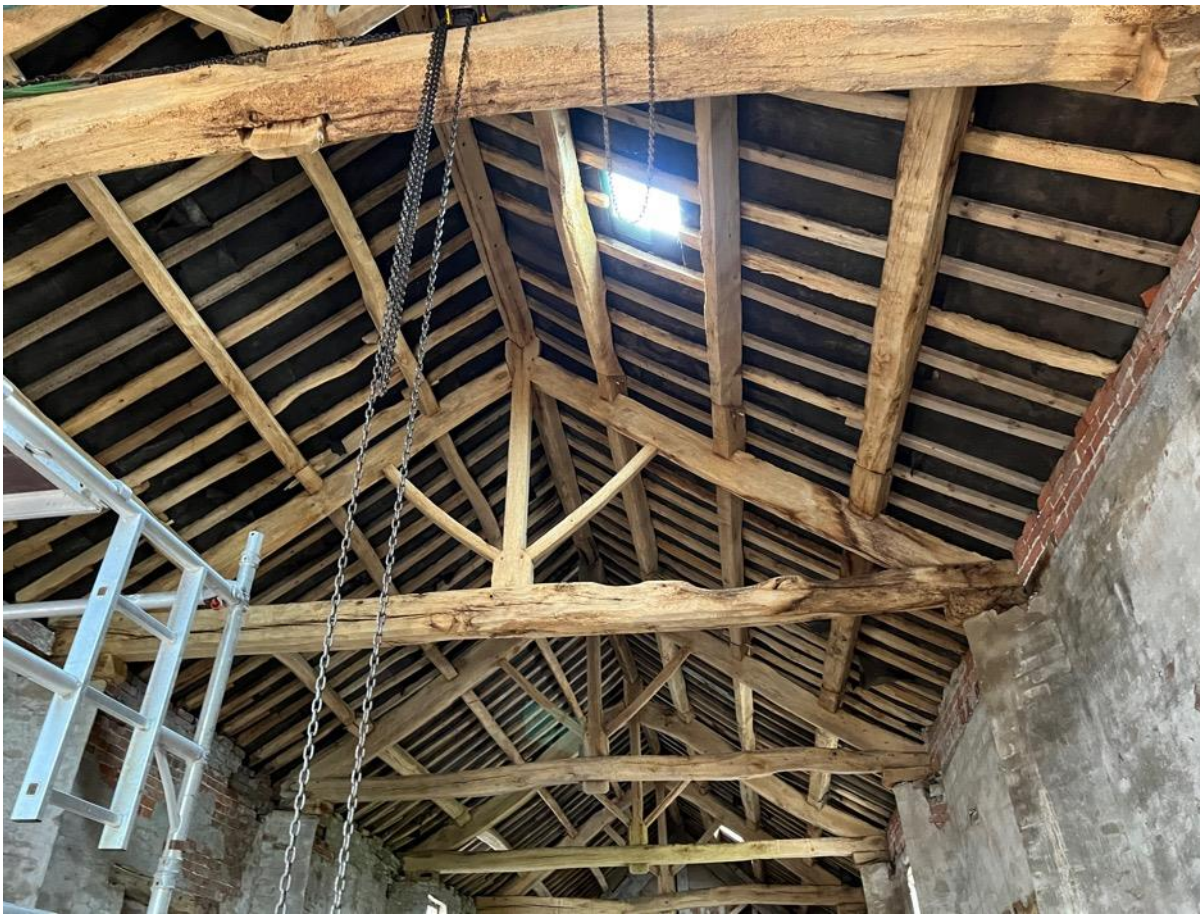
Photo 41 - Internal – main barn
