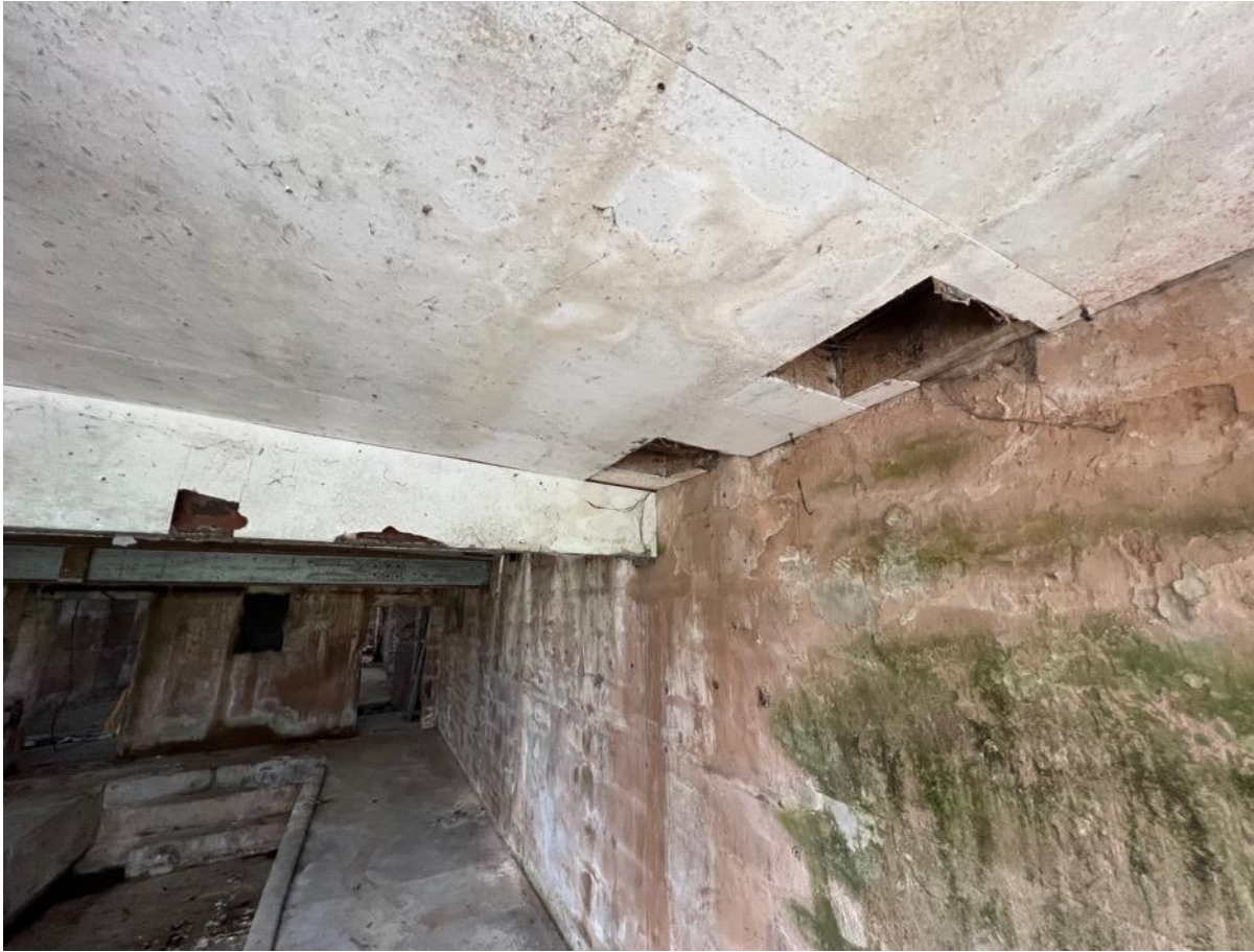
Photo 63 - extension to north west end
