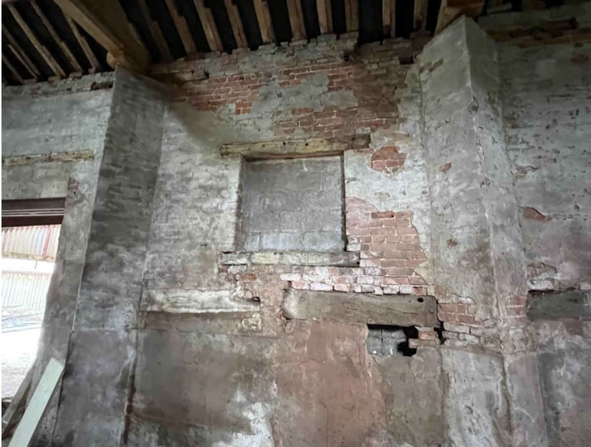
Photo 54 - Internal – main barn
