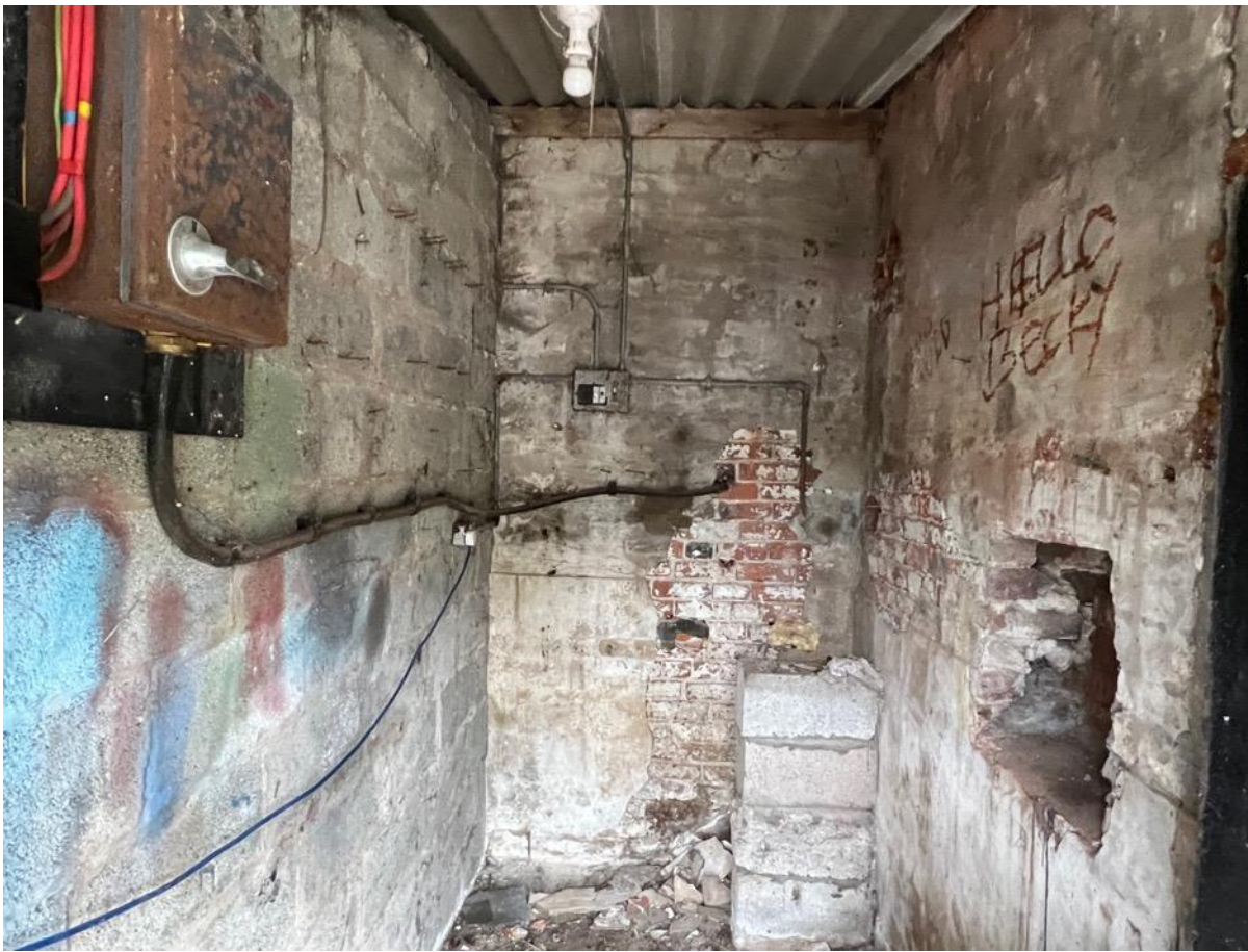
Photo 35 - Internal – extensions to north east elevation
