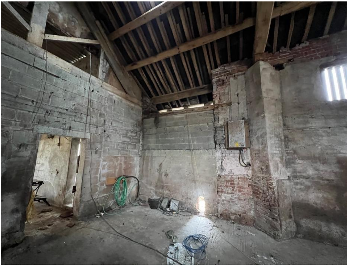
Photo 57 - Internal – main barn
