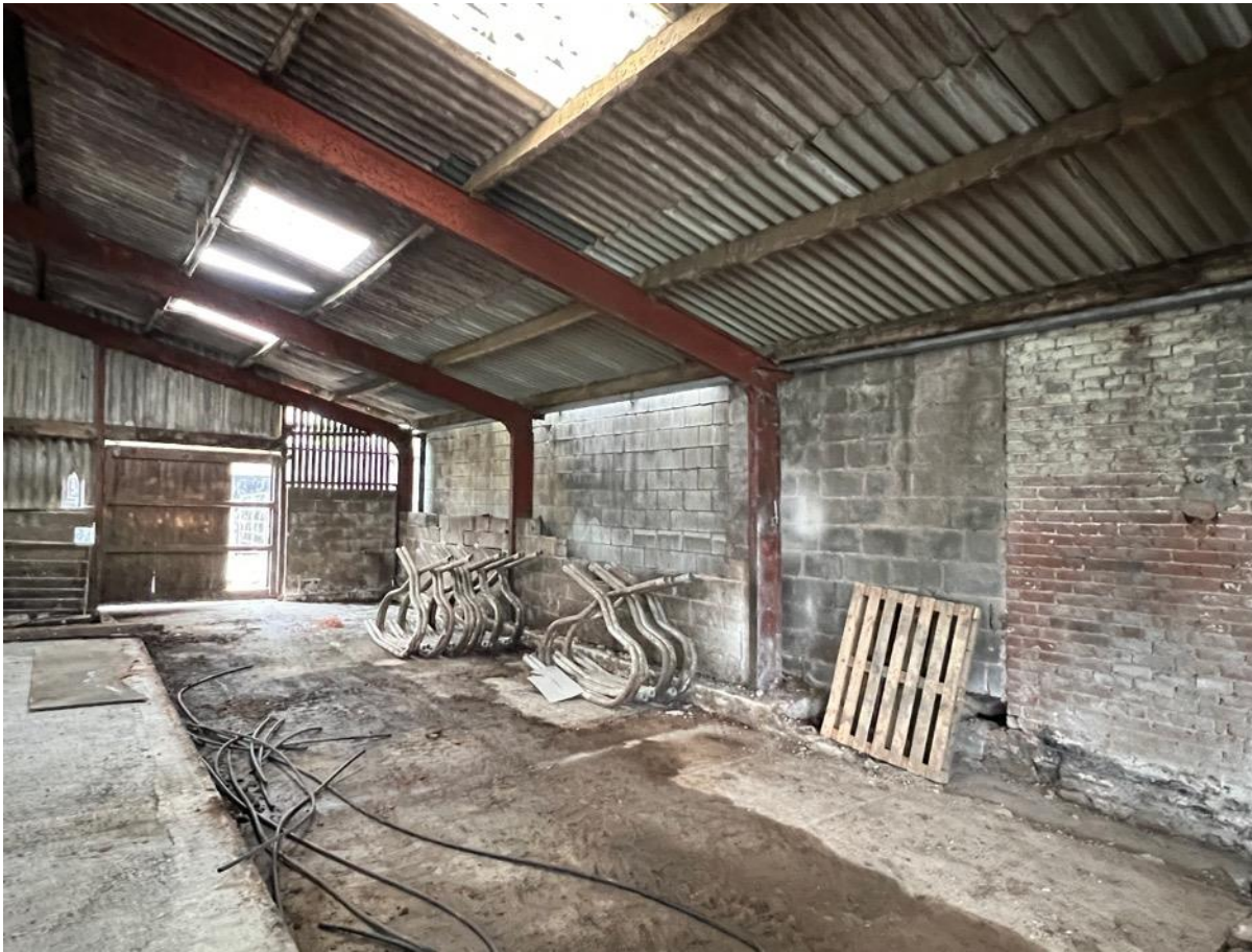
Photo 30 - South West Elevation
