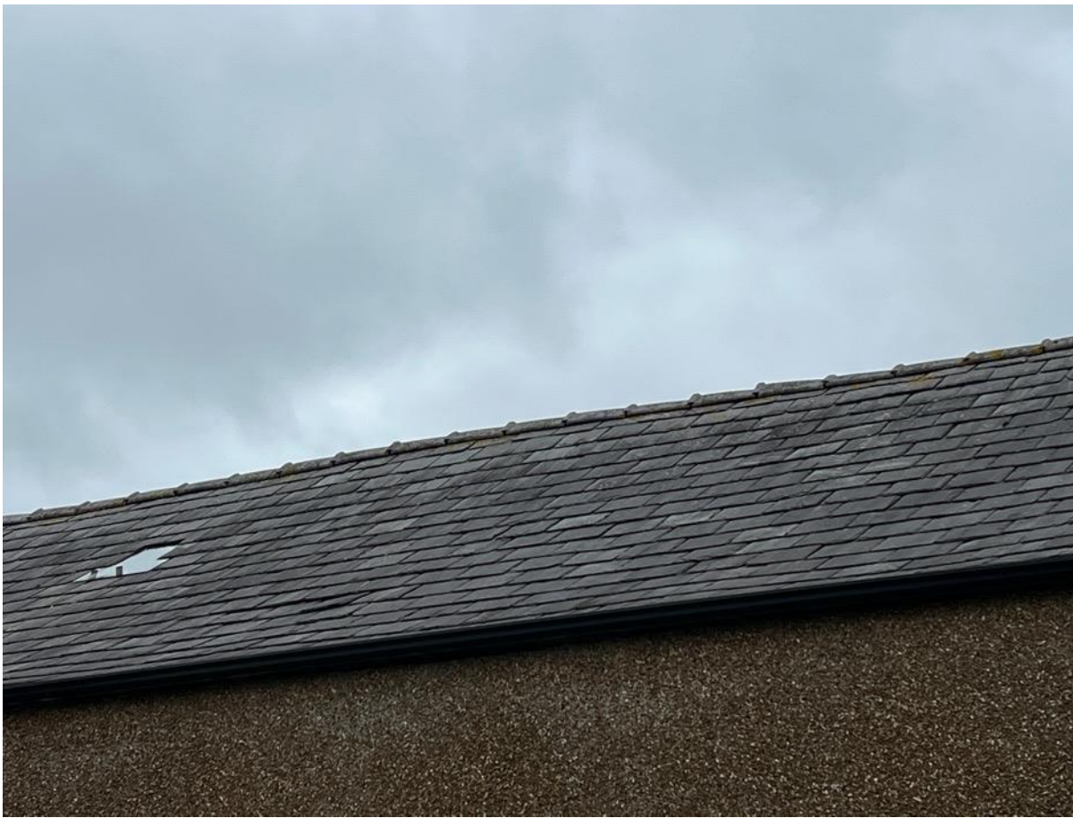
Photo 11 - North East Elevation Roof
