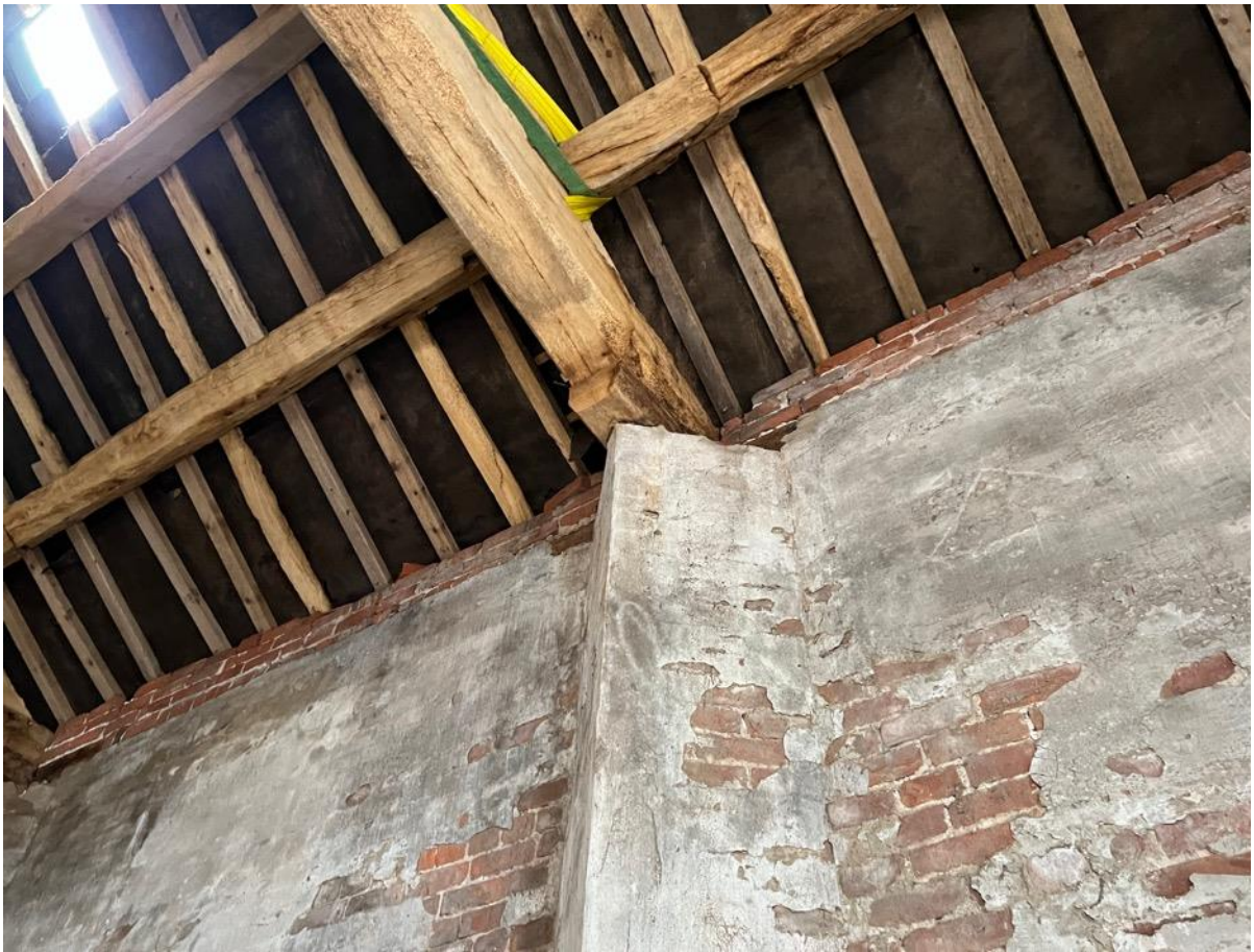
Photo 47 - Internal – main barn
