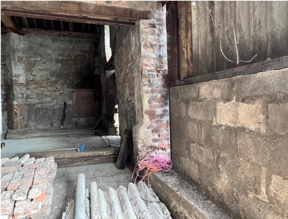
Photo 24 - South West Elevation
