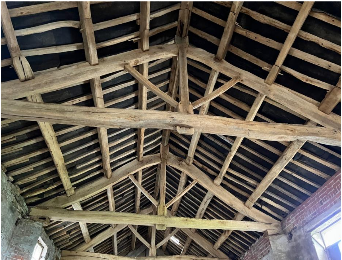
Photo 51 - Internal – main barn
