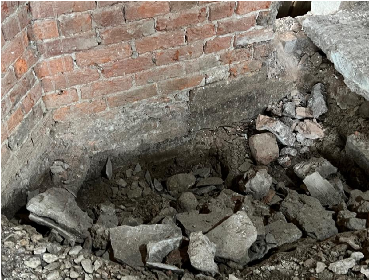
Photo 56 - Internal – main barn – excavation to founding stones
