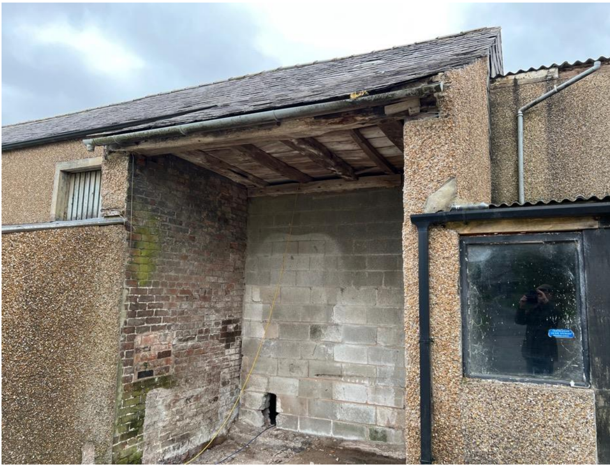
Photo 5 – North East Elevation – Original Barn Entrance
