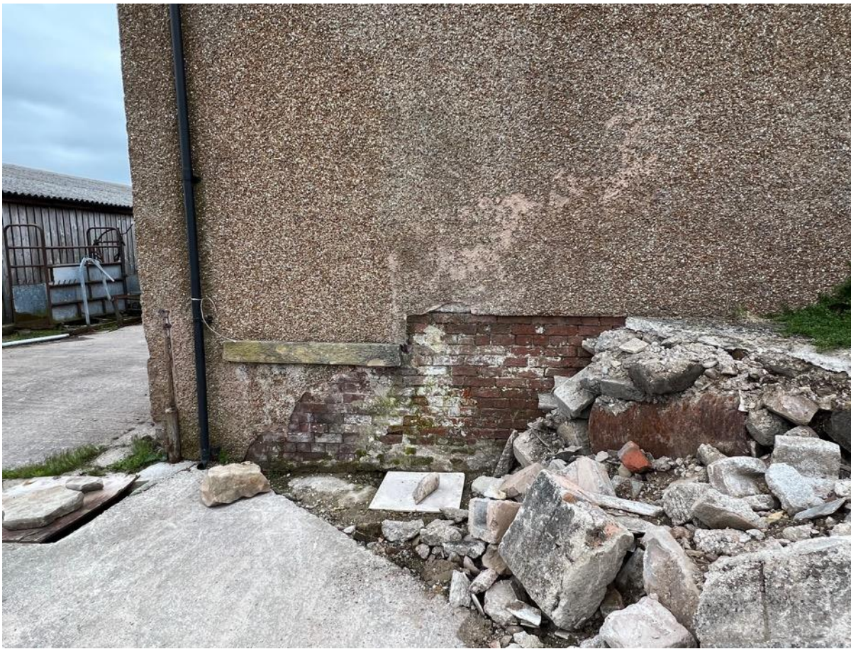
Photo 15 - North East Elevation
