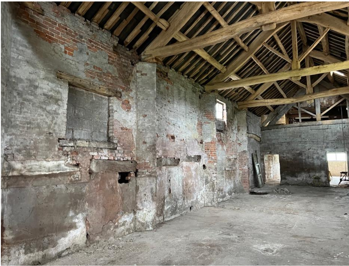
Photo 49 - Internal – main barn
