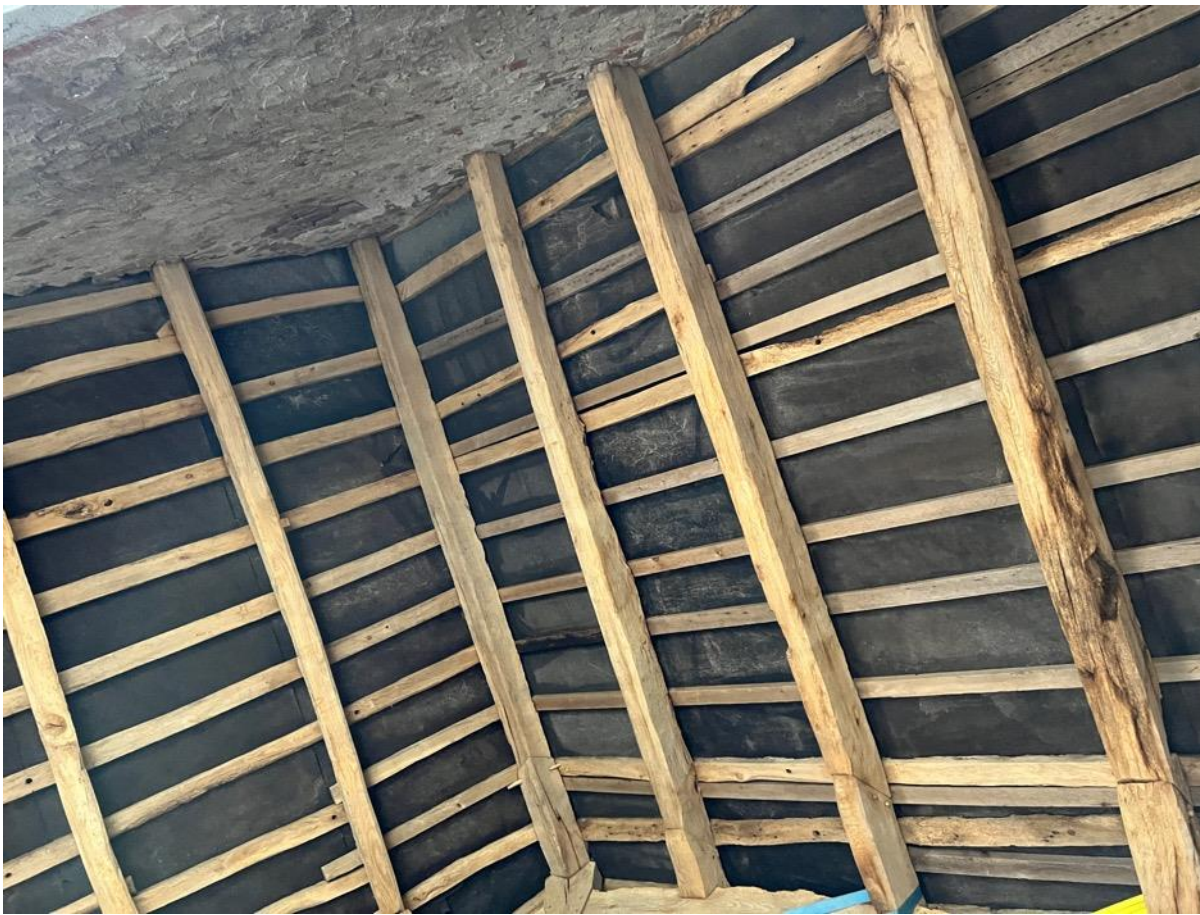
Photo 43 - Internal – main barn
