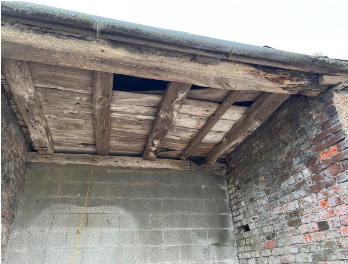
Photo 6 – North East Elevation – Original Barn Entrance
