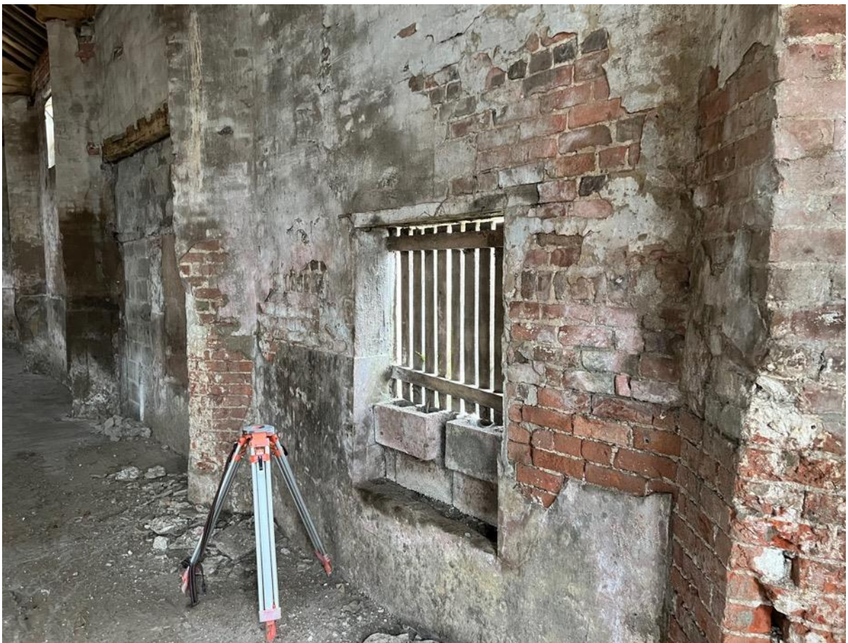
Photo 48 - Internal – main barn
