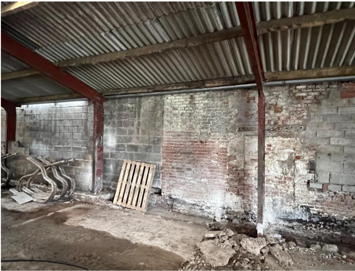
Photo 29 - South West Elevation
