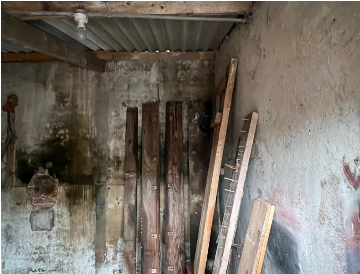
Photo 34 - Internal – extensions to north east elevation
