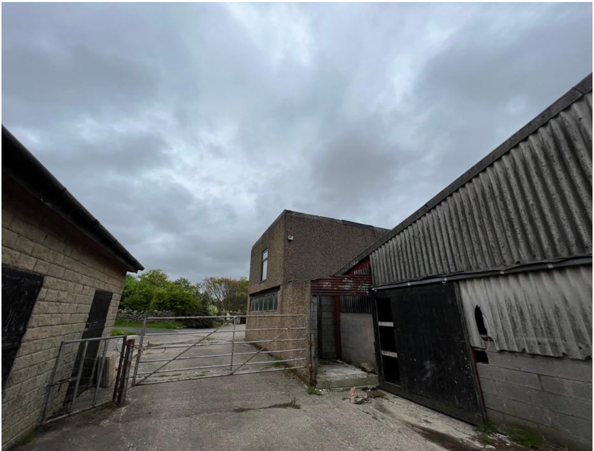
Photo 65 – North West elevation of extension
