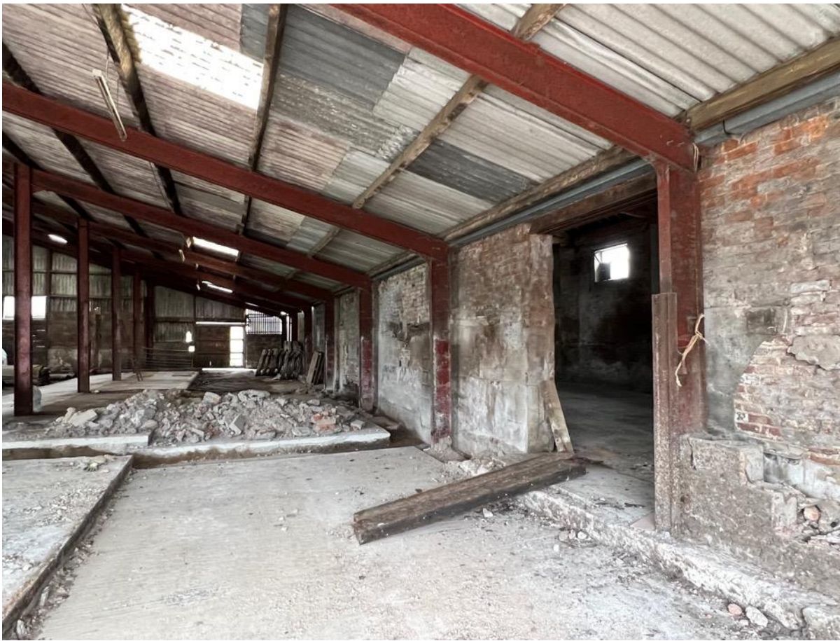
Photo 23 – South West Elevation
