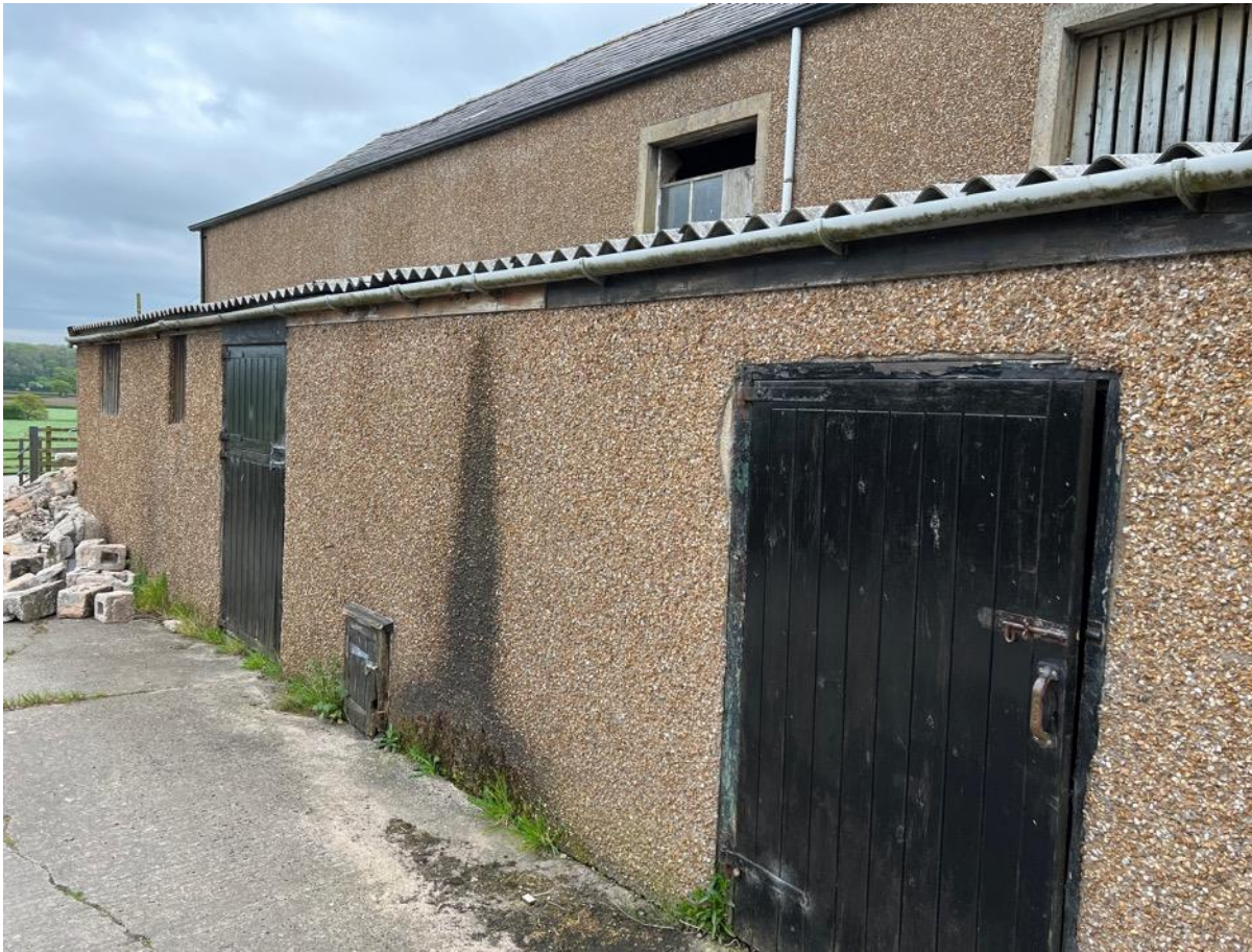
Photo 8 – North East Elevation – Extensions along elevation
