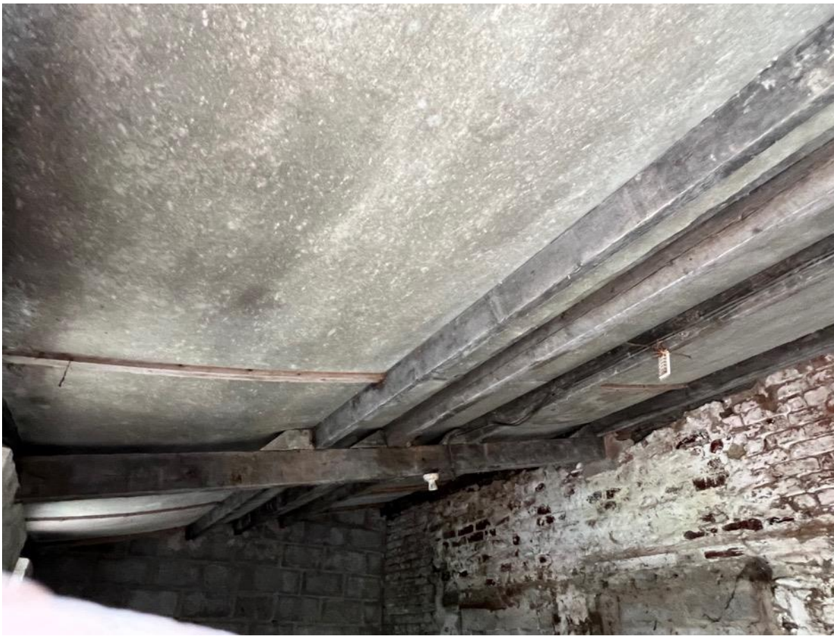
Photo 39 - Internal – extensions to north east elevation
