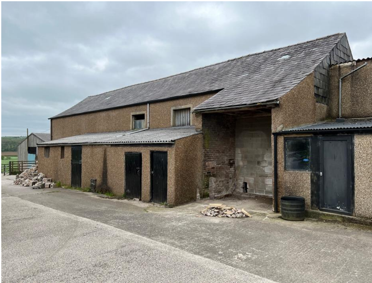
Photo 1 - North East Elevation
