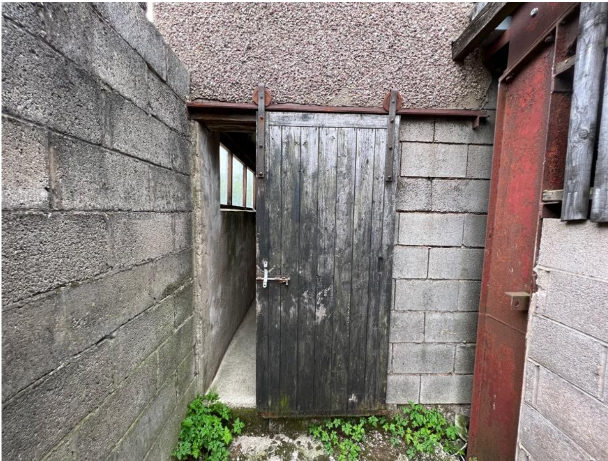
Photo 64 – door on north west elevation to extension
