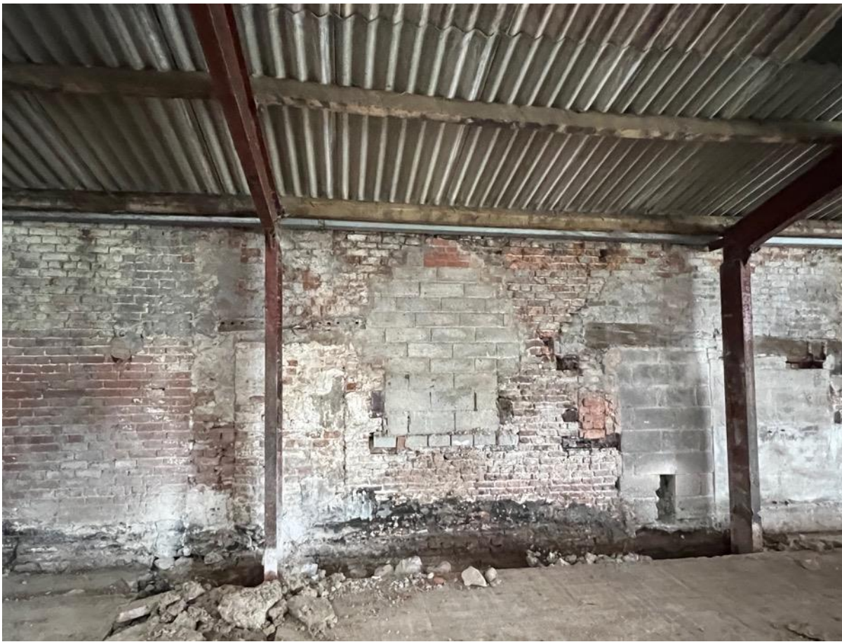
Photo 31 - South West Elevation
