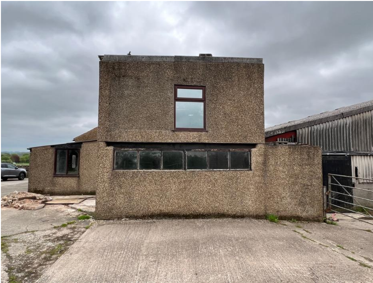
Photo 32 – North West Elevation of extension
