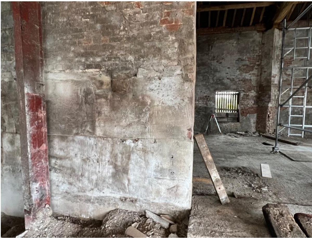
Photo 25 – South West Elevation
