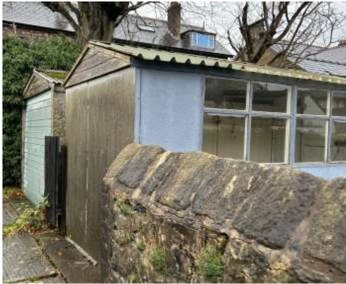
FIGURE 2: PHOTO OF DETACHED GARAGES TO BE REMOVED
