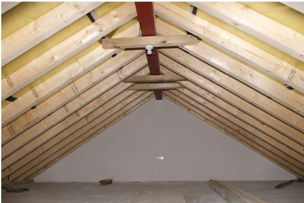
Image showing roof void with intact modern roof liner above detached double garage
