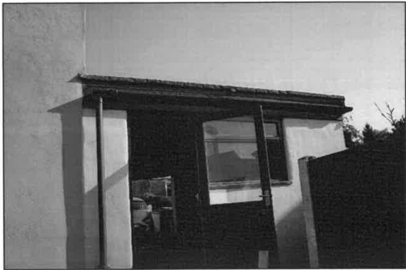
Photo 3: Northwest elevation of the garage.
