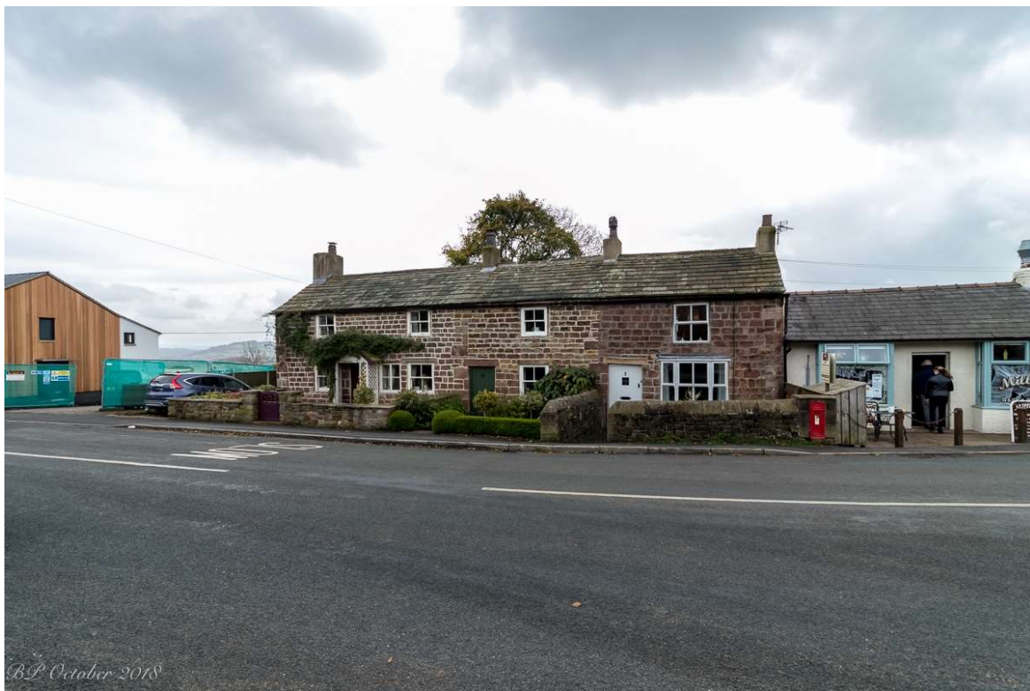
Figure 3 2,4 AND 6 WHALLEY ROAD
