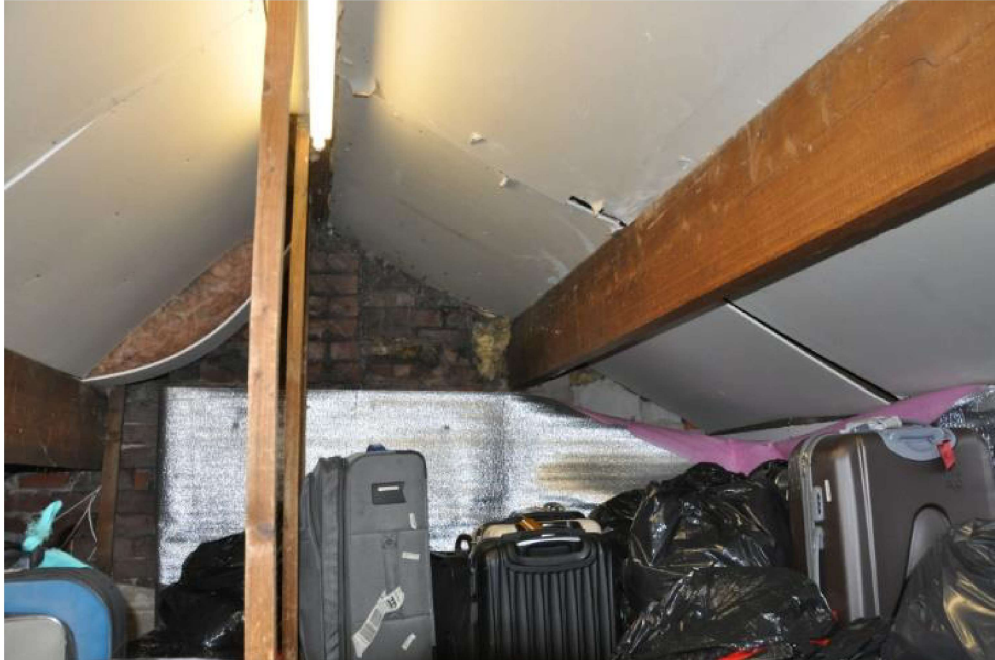
Image showing roof void used for storage
