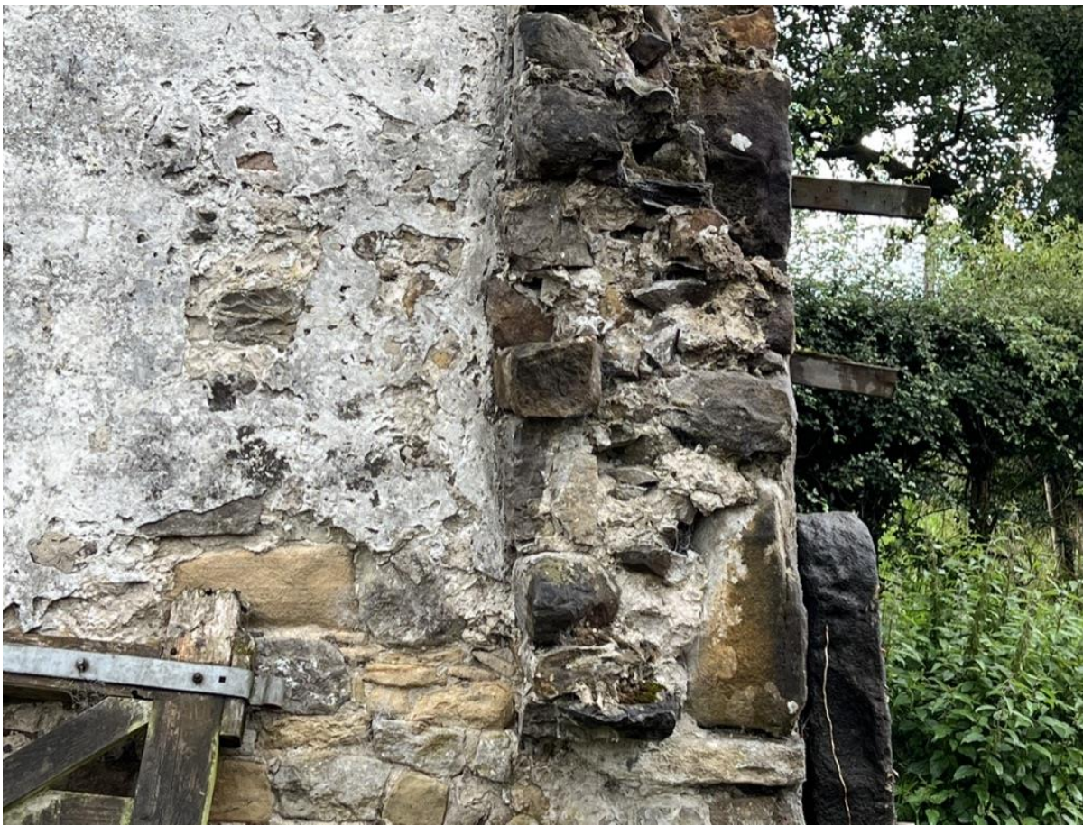
Photo 9 – North East Corner
