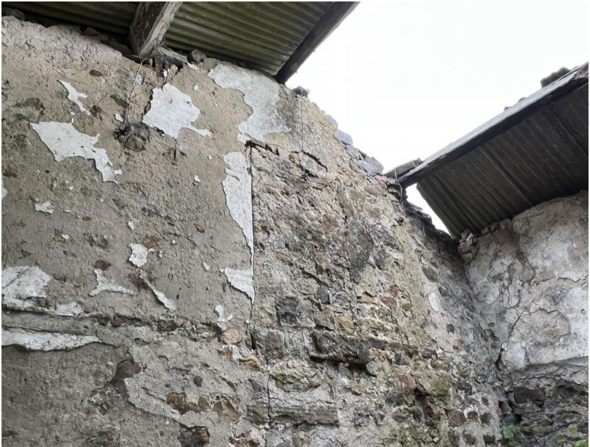
Photo 18 – Internal east elevation
