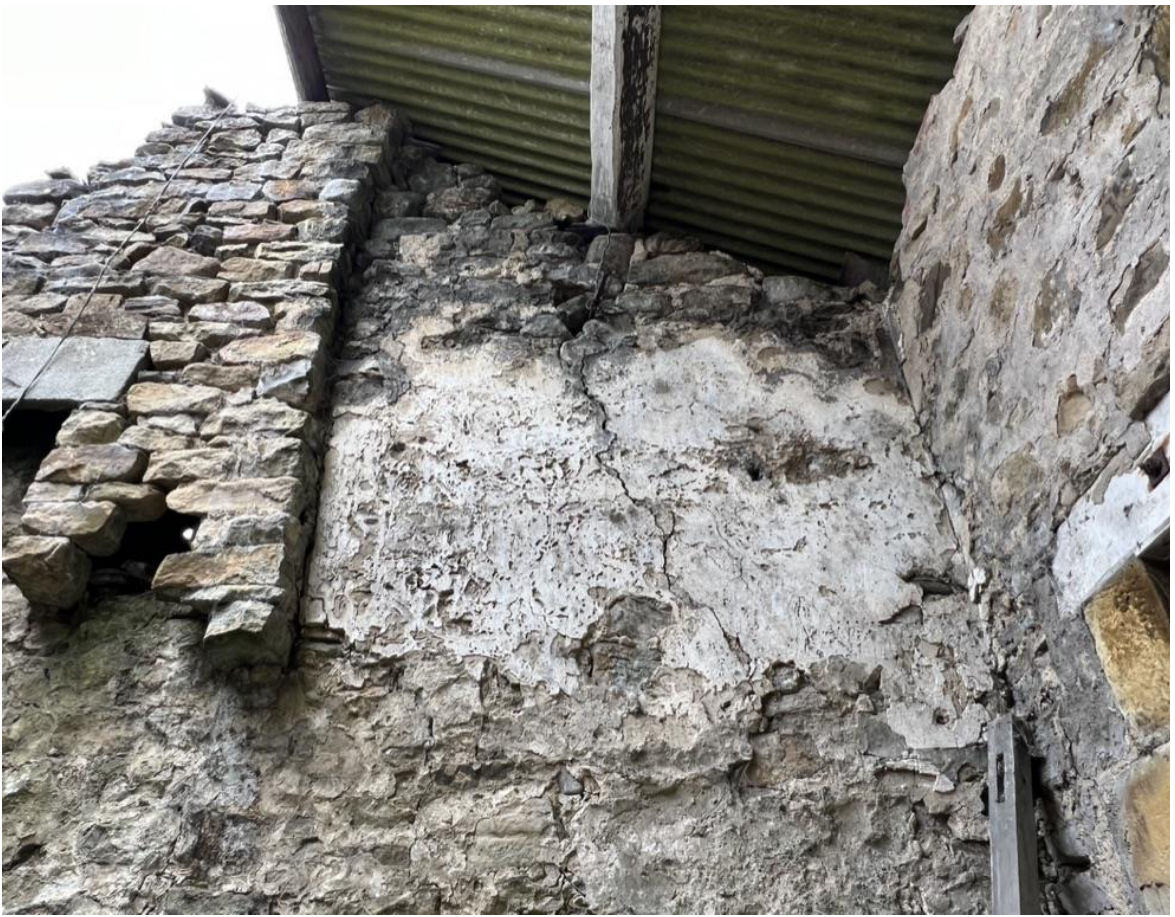
Photo 19 – Internal west elevation
