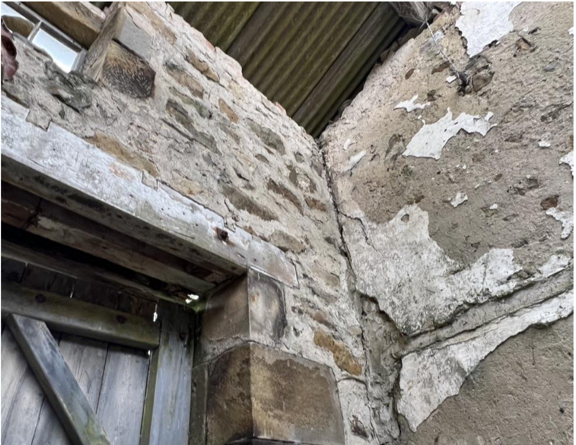
Photo 20 – Internal – north elevation
