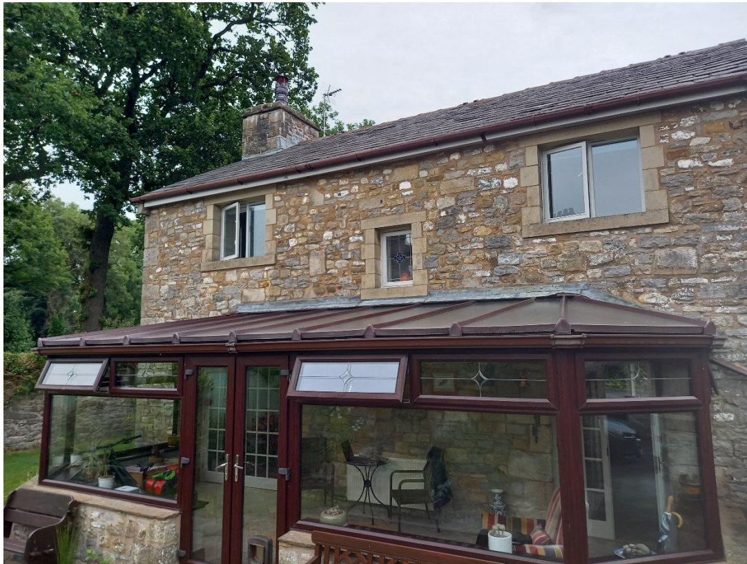
Existing UPVC conservatory extension to be demolished.
