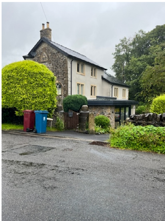
Precedent 2, Extension to Hydro Lodge, located approximately 2miles away visible from Sawley Road.
