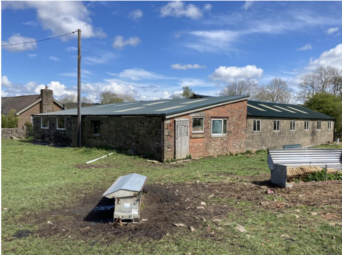
Figure 3: An image of the site from the west
