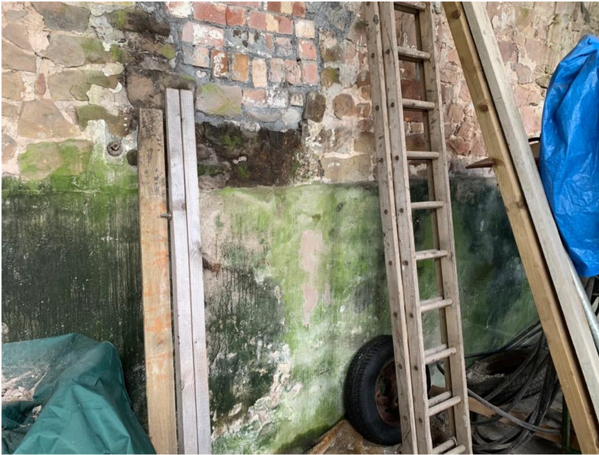
Photo 50 - Internal to newer blockwork building – original building south elevation
