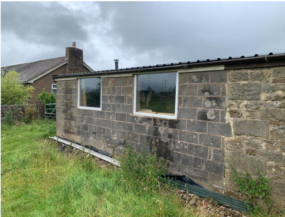
Photo 17 – North Elevation – block section to extension
