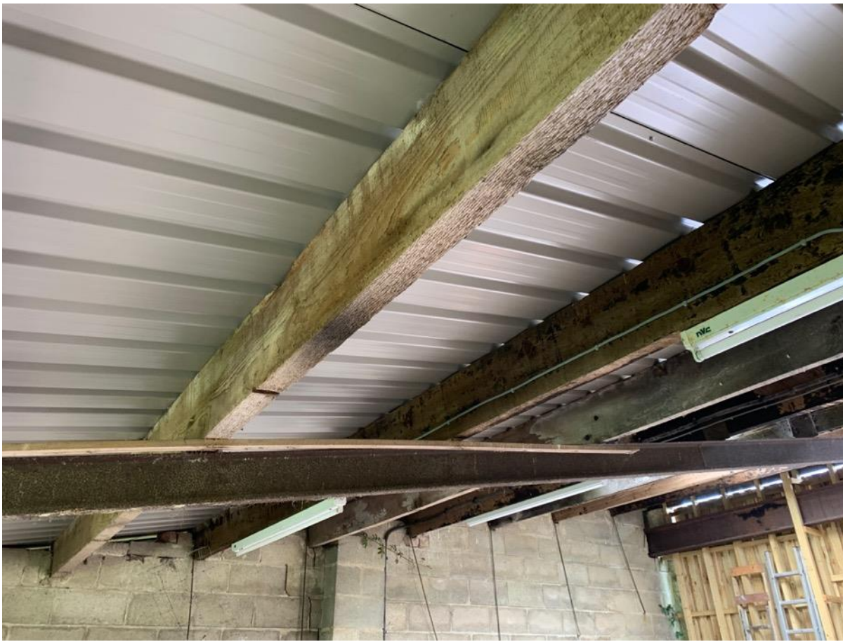
Photo 37 - Internal to extension of original building – timber purlin and block pier
