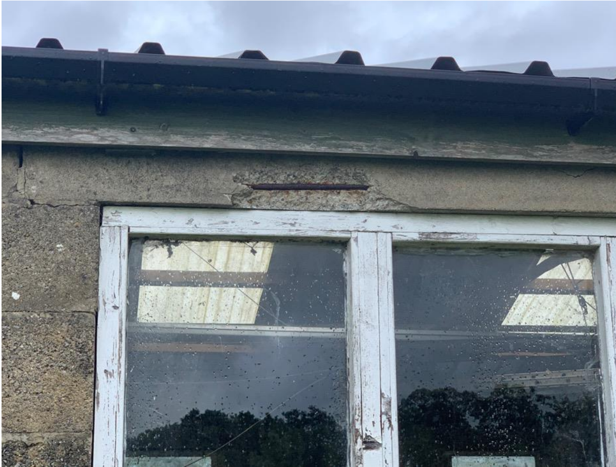
Photo 8 – Lintel on west elevation
