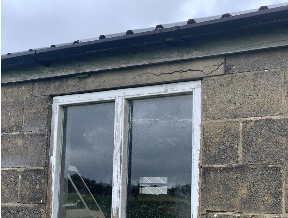
Photo 10 – Lintel to west elevation
