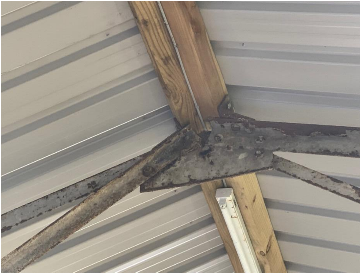
Photo 56 - Internal to newer blockwork building – truss apex
