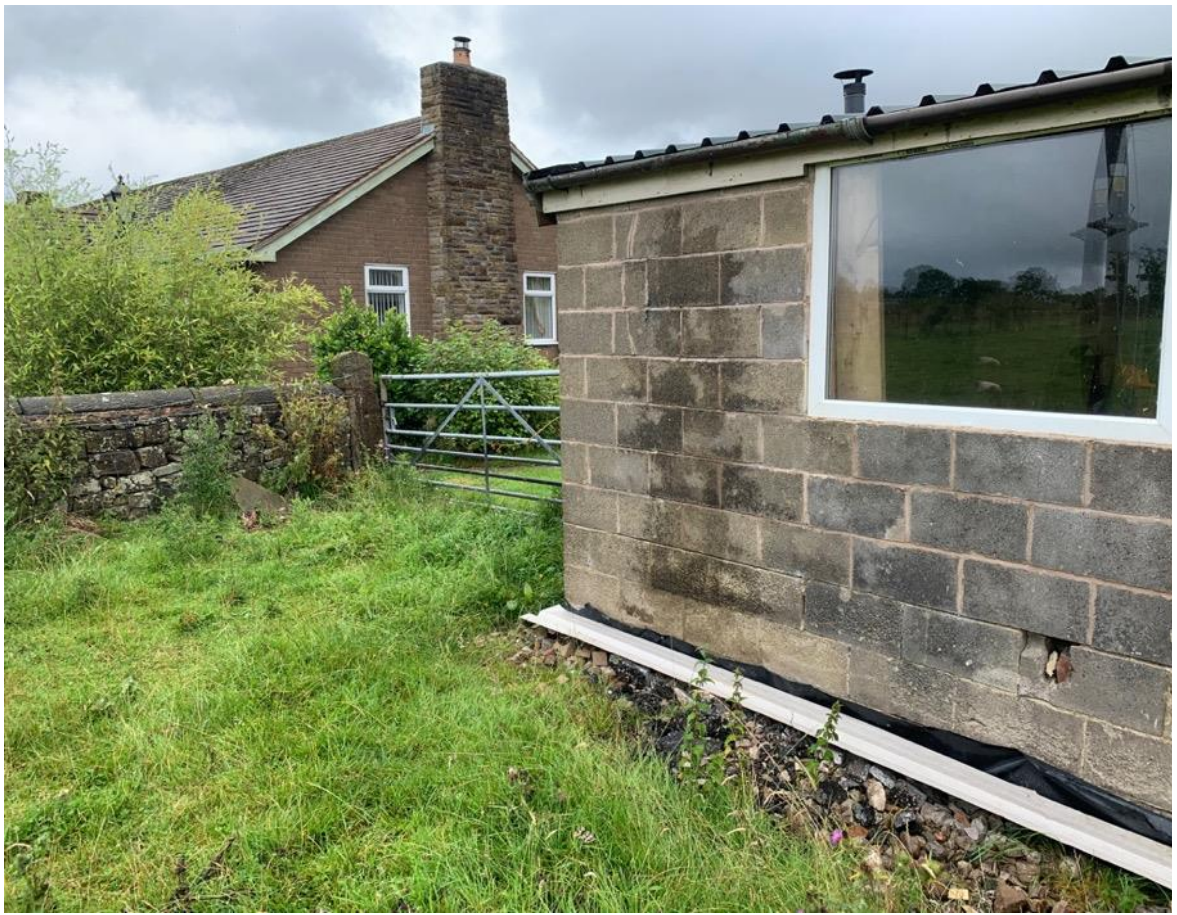
Photo 19 – North Elevation – north east corner
