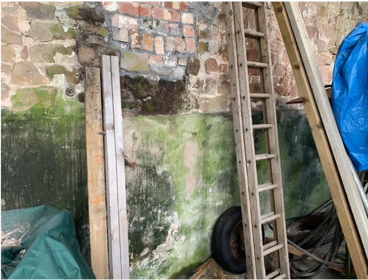
Photo 51 - Internal to newer blockwork building – original building south elevation
