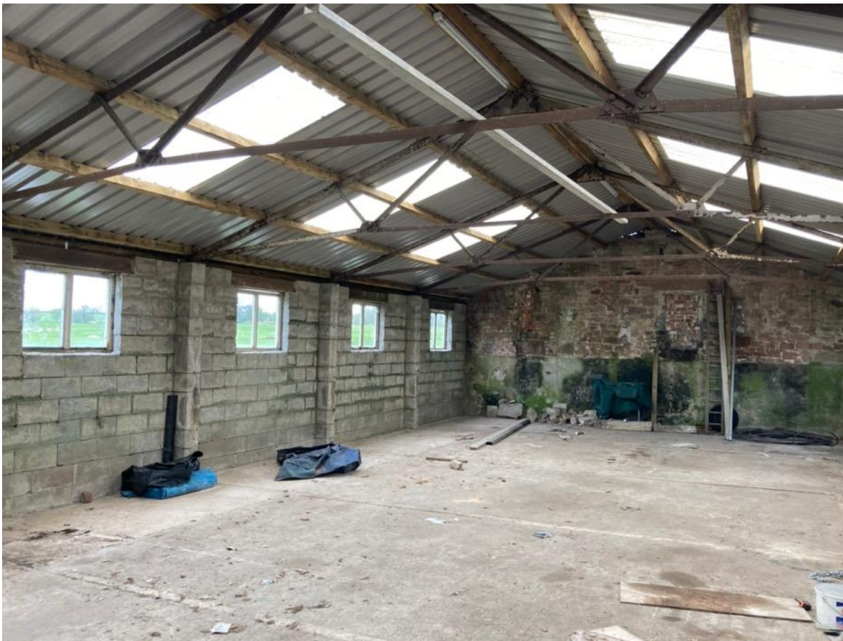
Photo 47 - Internal to newer blockwork building – looking north to original building
