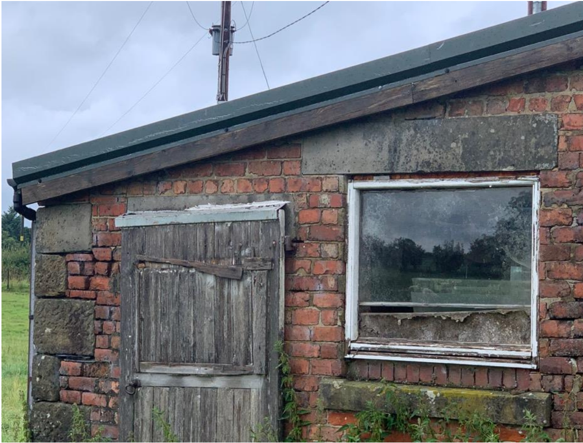
Photo 12 – West elevation north end
