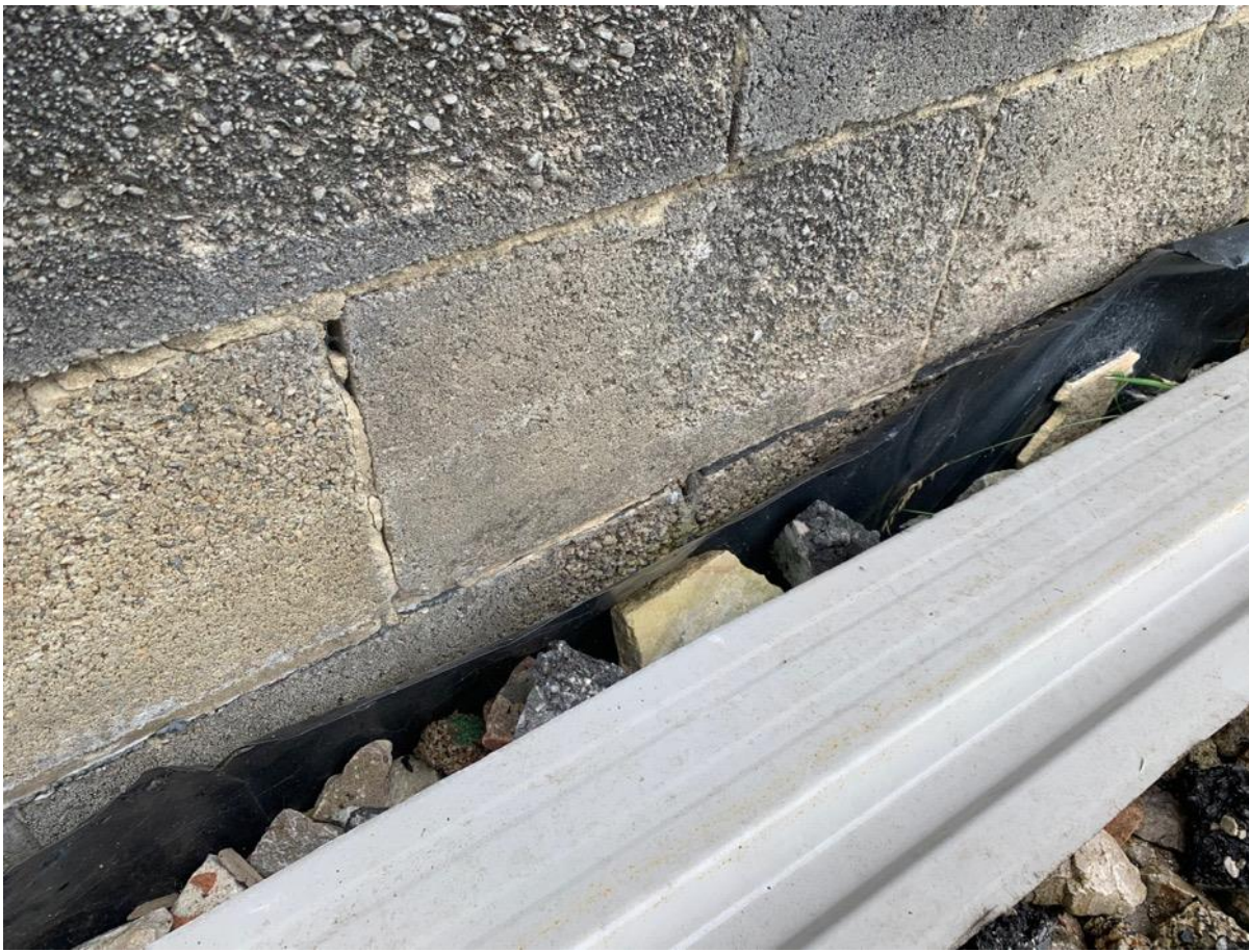
Photo 23 - North Elevation blockwork – DPC membrane
