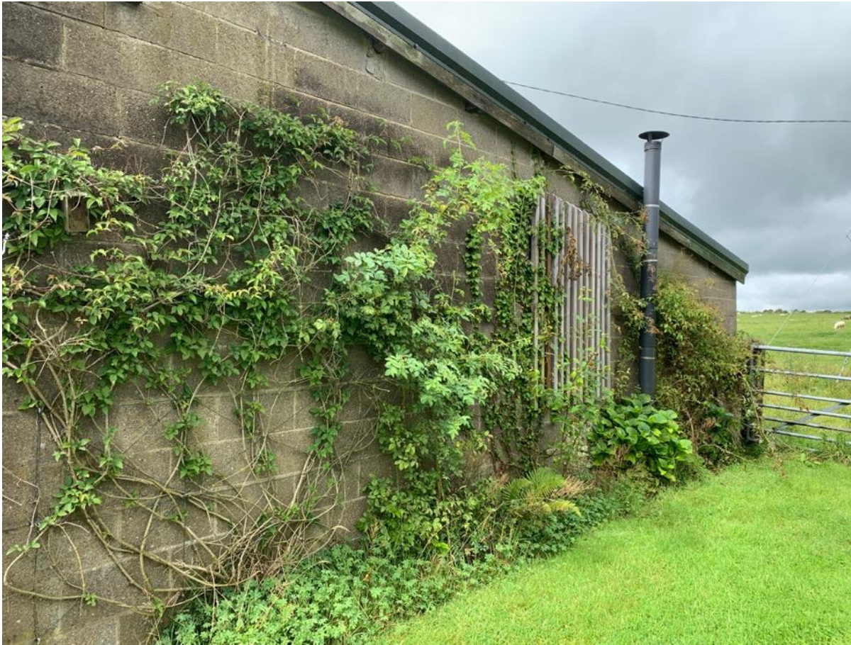
Photo 30 - Blockwork to east elevation of mono-pitch extension to original building
