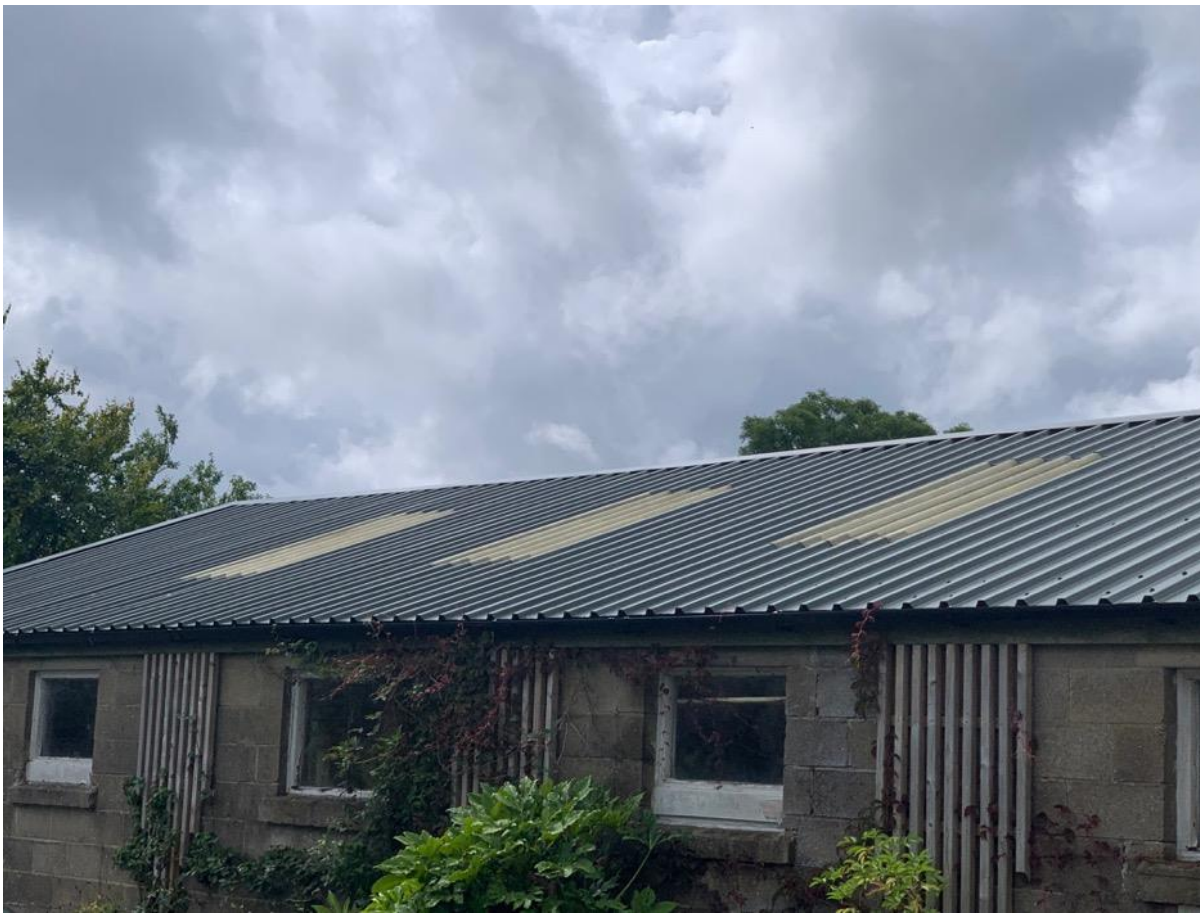
Photo 29 – Roof sheeting to blockwork building
