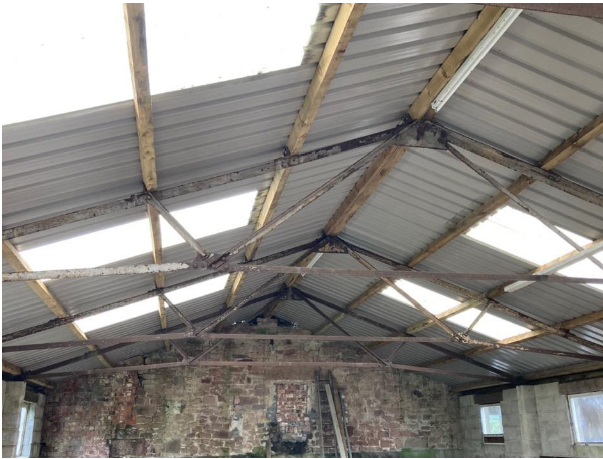
Photo 53 - Internal to newer blockwork building – original building south elevation
