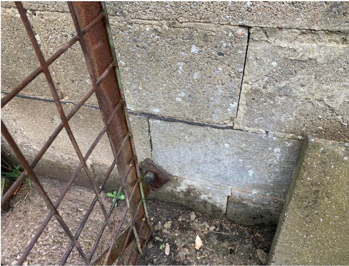
Photo 2 - South Elevation DPC
