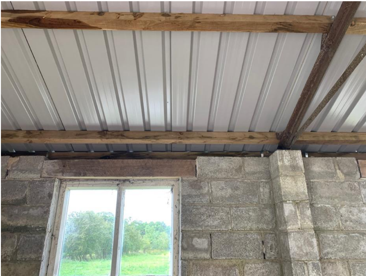
Photo 44 - Internal to newer blockwork building
