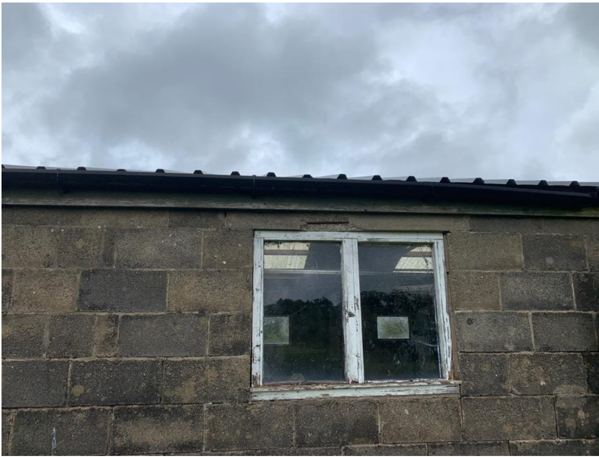
Photo 11 - Lintel to west elevation
