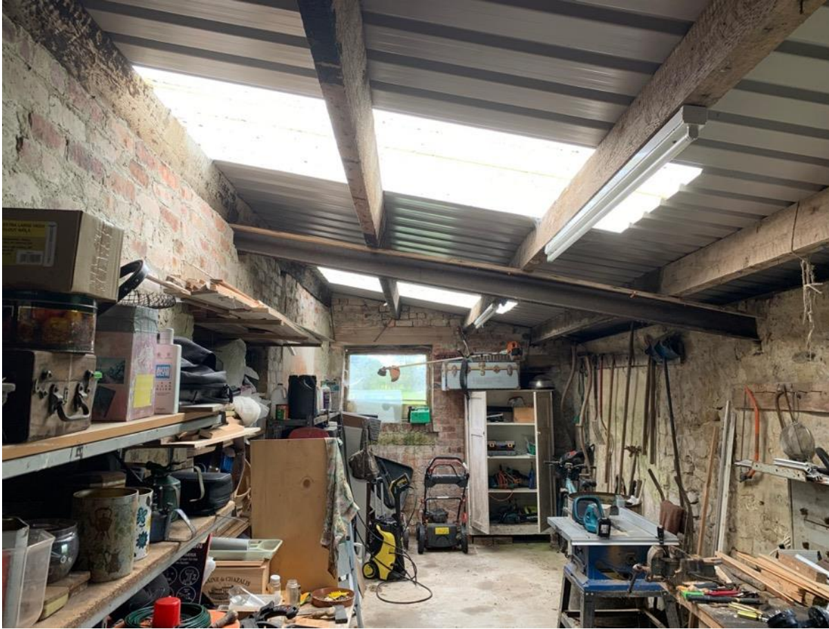
Photo 38 - Internal to original stone building
