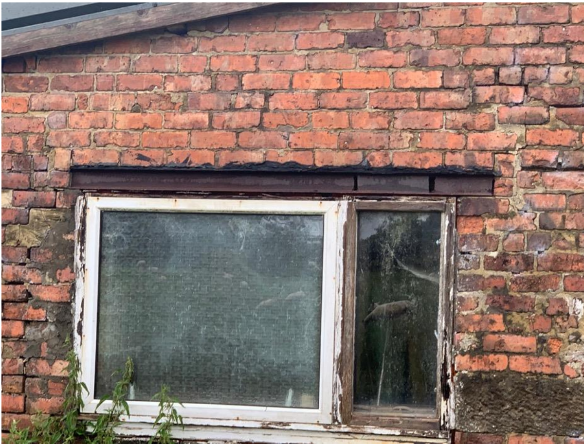
Photo 13 - West elevation north end – steel lintel
