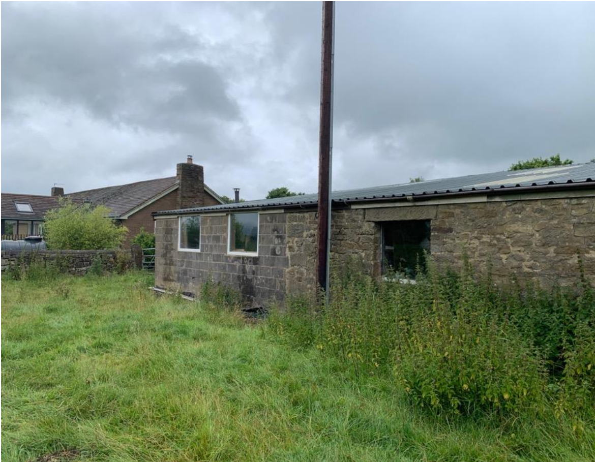
Photo 18 – North Elevation – indicating original stone building and blockwork extension
