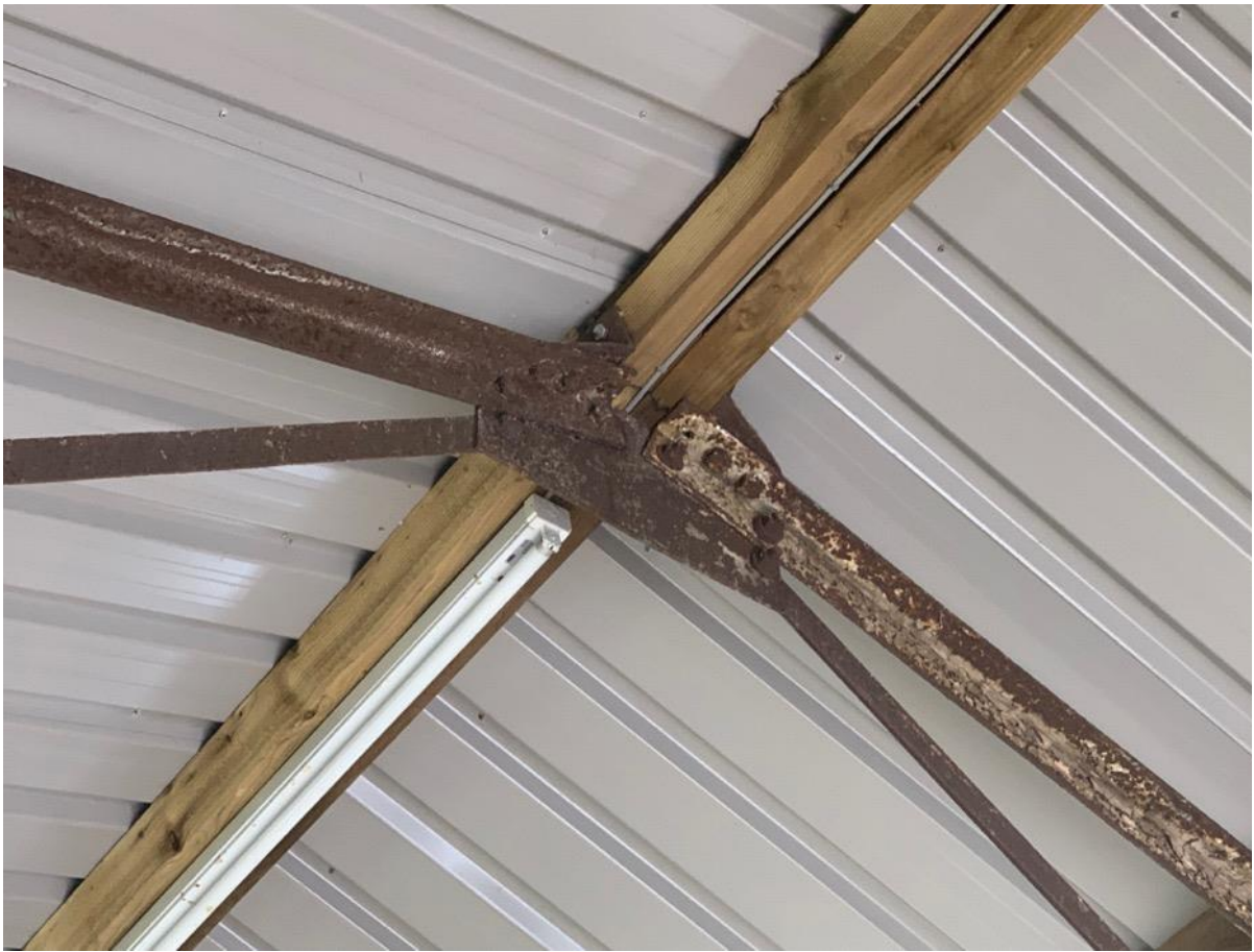
Photo 45 - Internal to newer blockwork building – apex of roof truss
