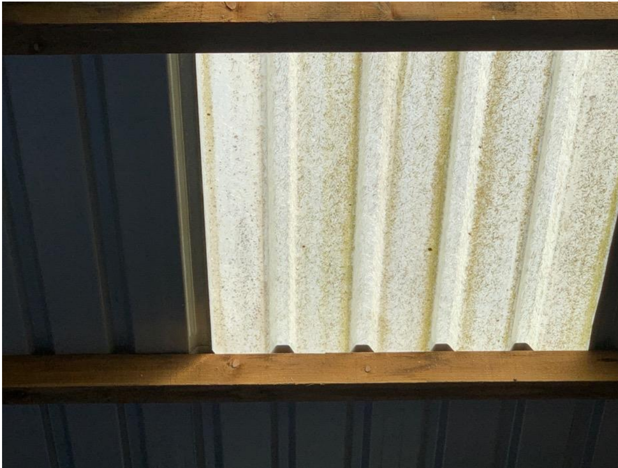
Photo 54 - Internal to newer blockwork building – roof sheeting
