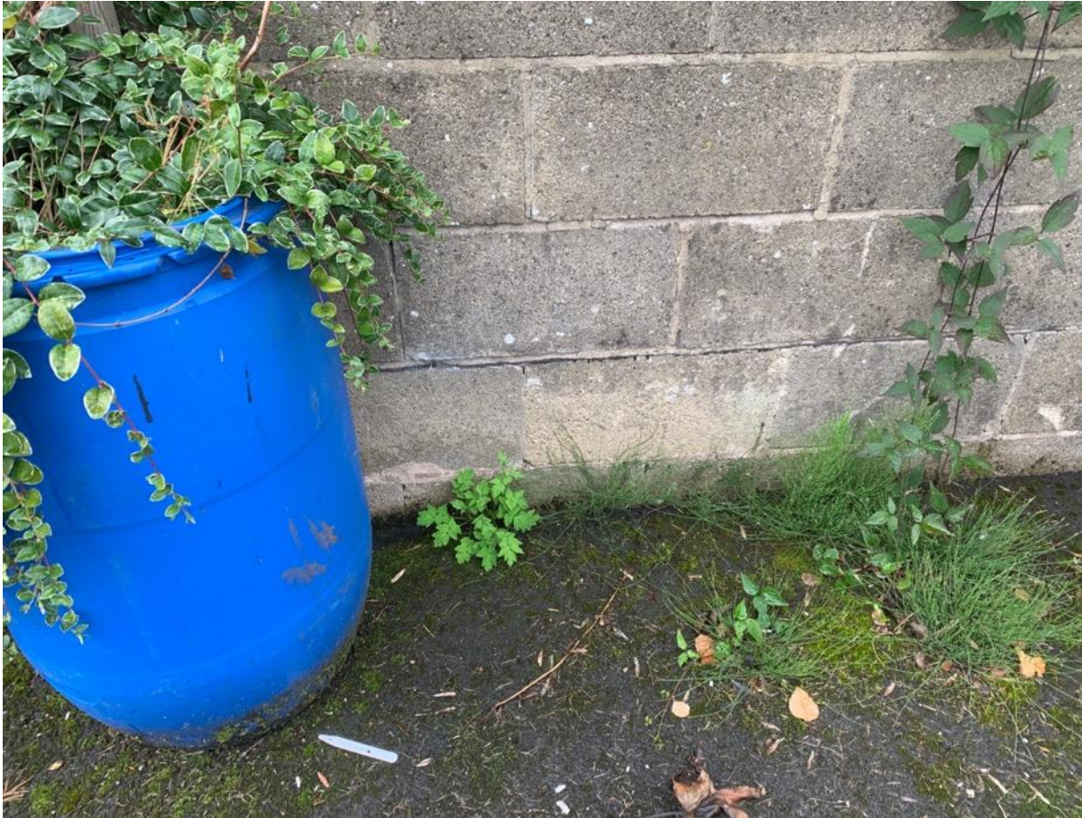
Photo 26 – East Elevation DPC
