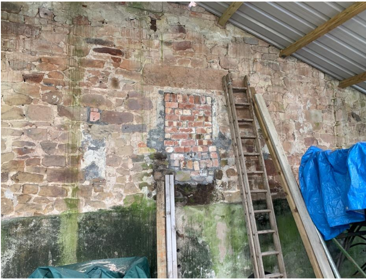
Photo 49 - Internal to newer blockwork building – original building south elevation
