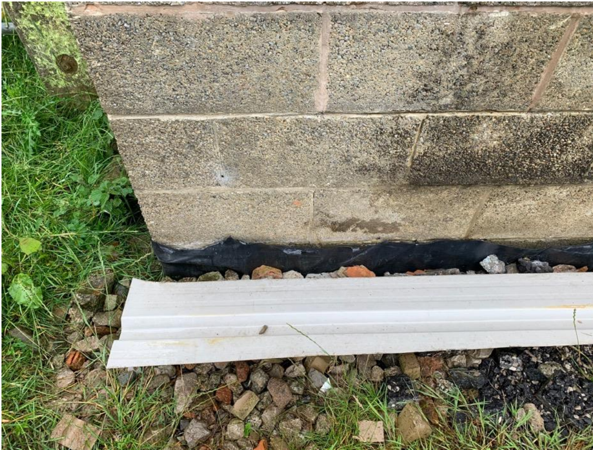
Photo 22 – North Elevation blockwork – DPC membrane
