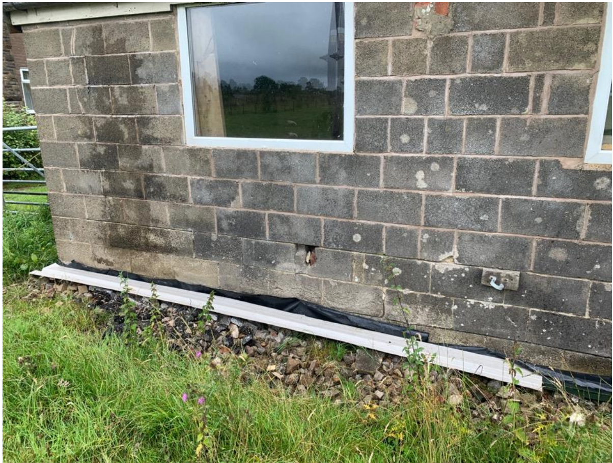
Photo 20 – North Elevation block section showing DPC
