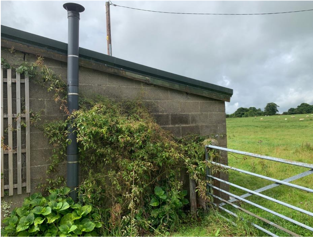
Photo 28 – Blockwork to east elevation of mono-pitch extension to original building
