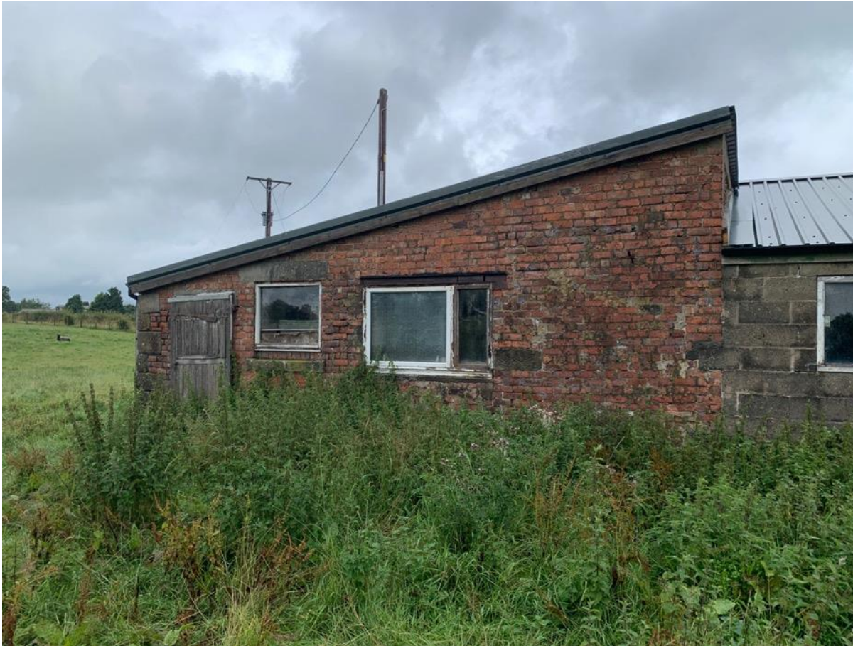
Photo 16 – West Elevation – indicating mono-pitch roof
