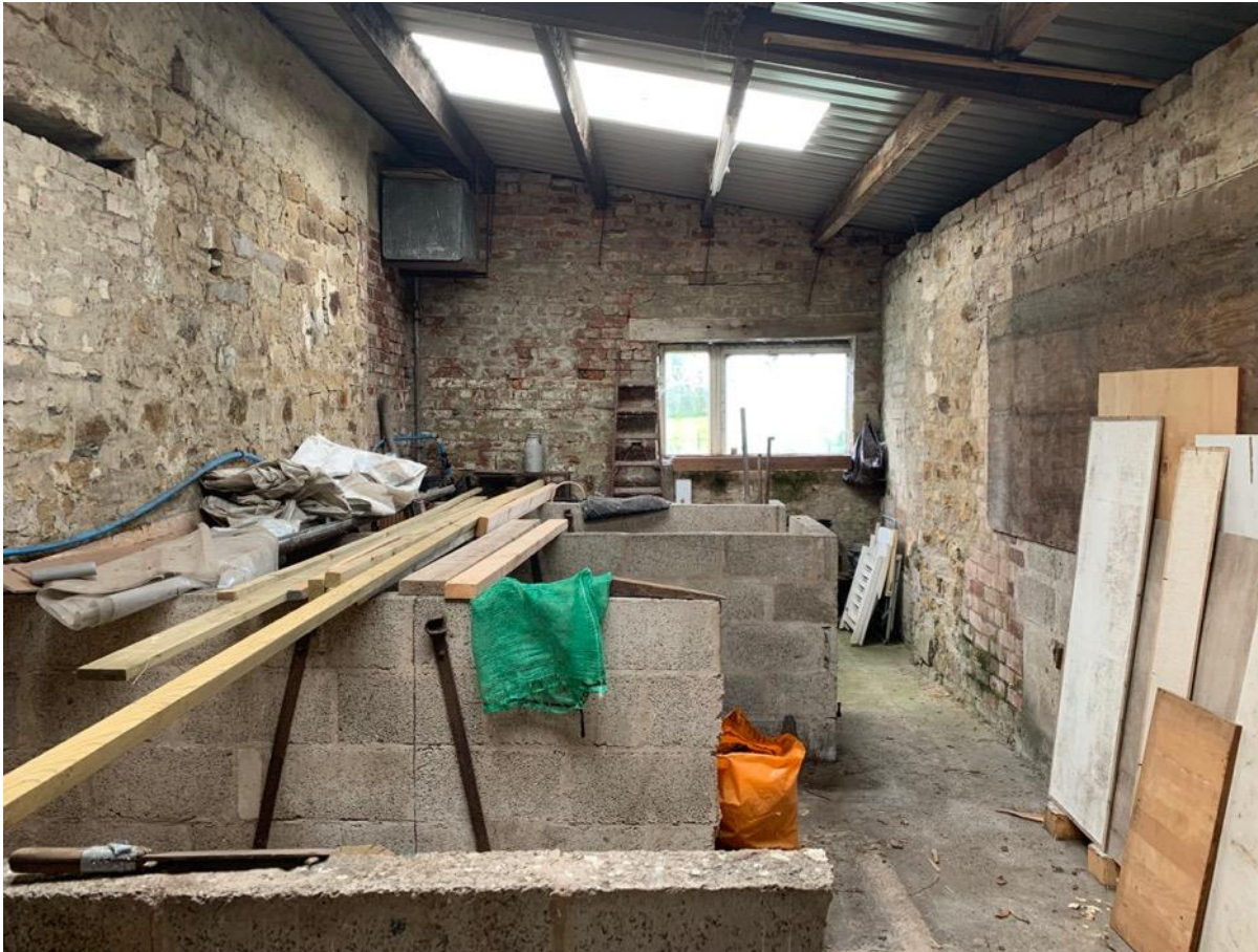
Photo 40 - Internal to original building
