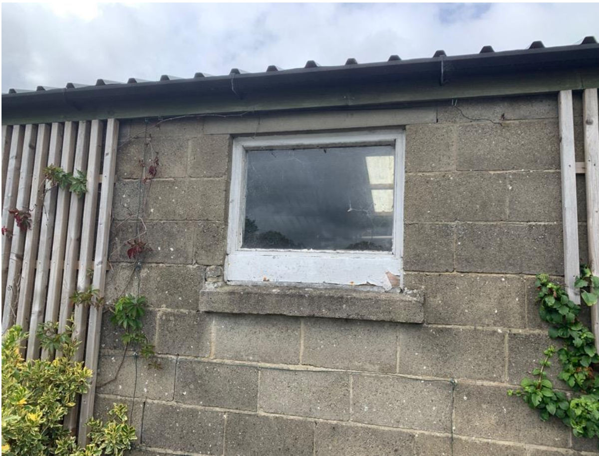
Photo 25 – East Elevation – Window detail
