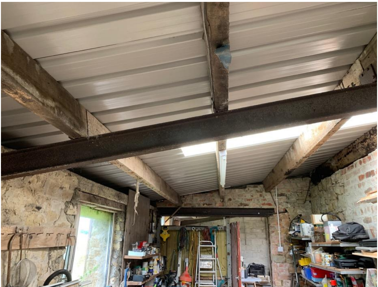
Photo 42 - Internal to original building
