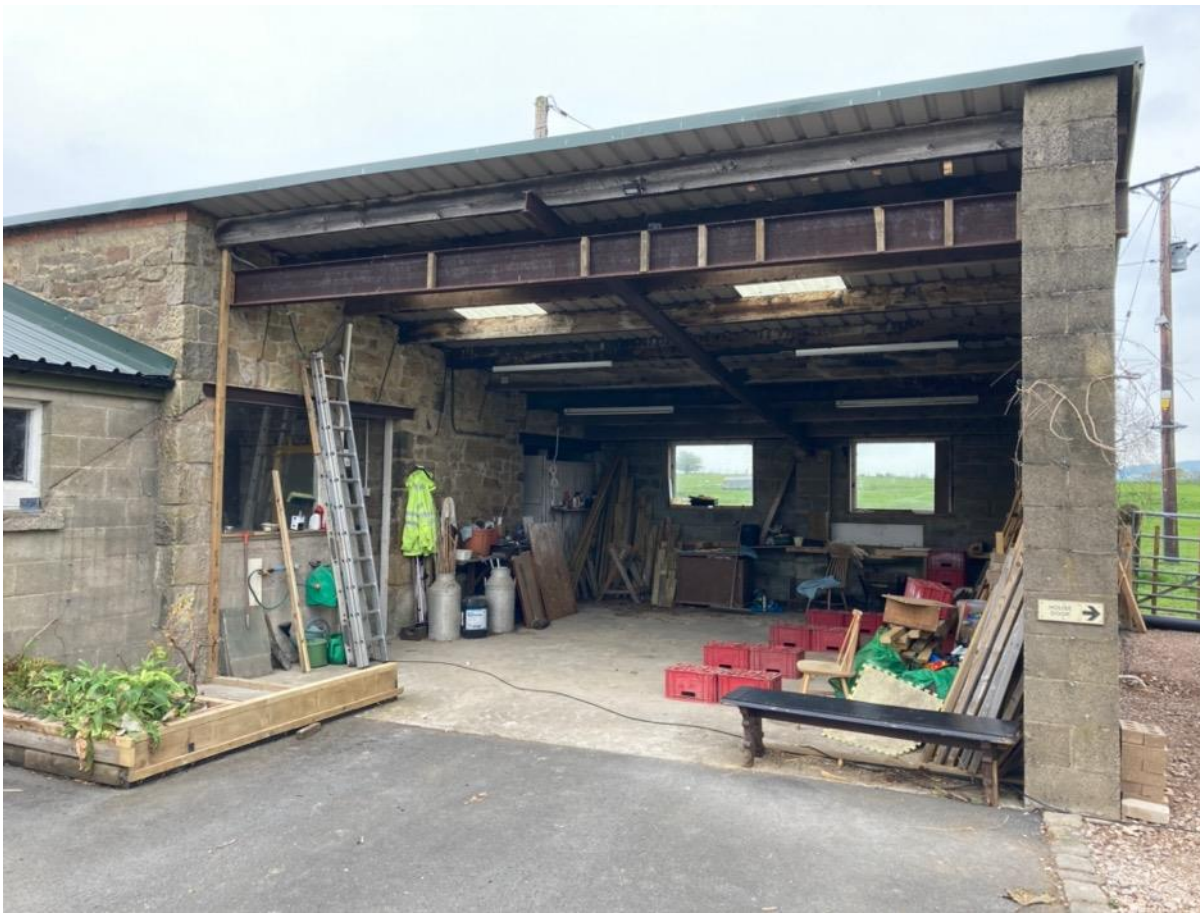
Photo 27 – Large Opening to original building and extension - south elevation
