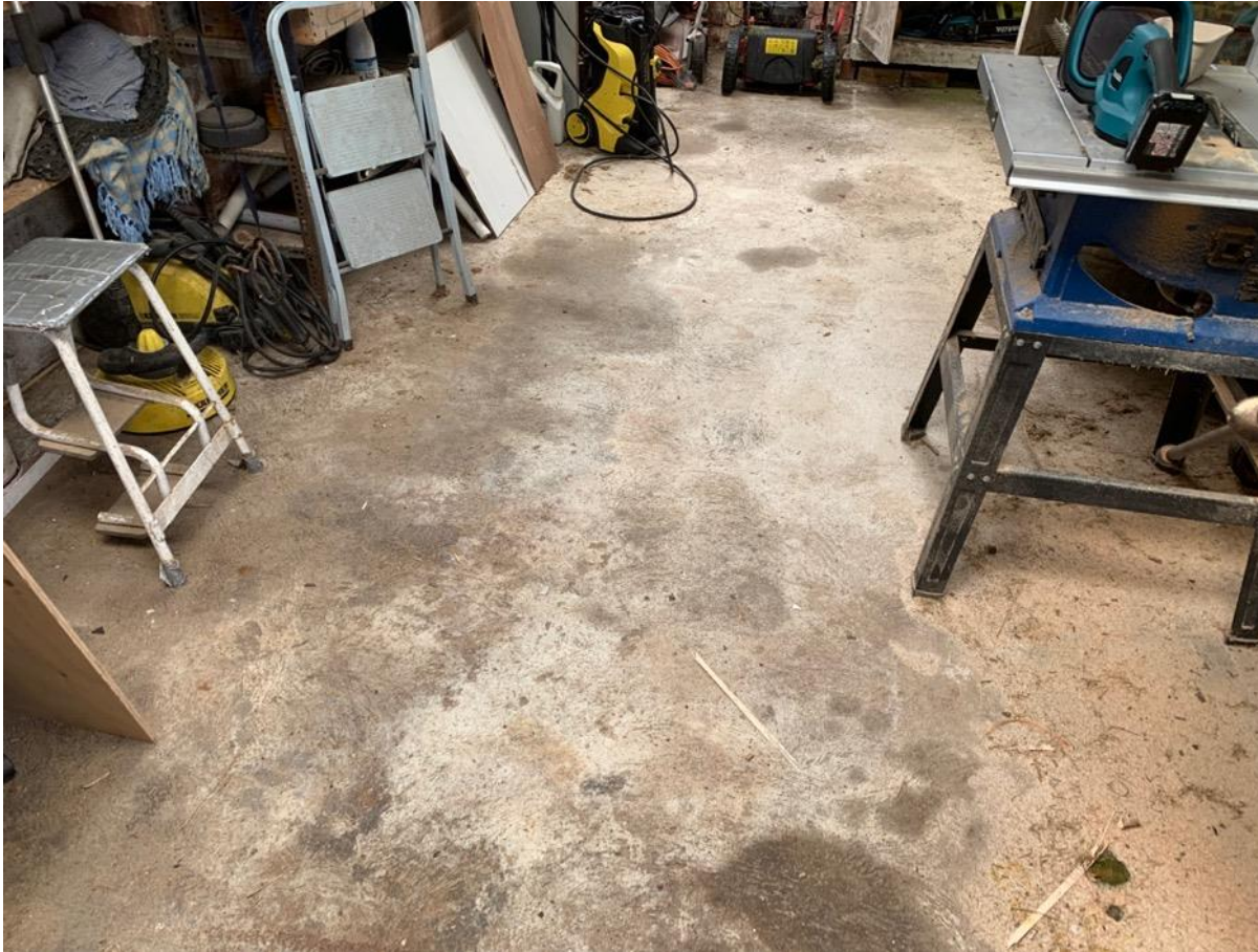
Photo 43 - Internal to original building – concrete floor
