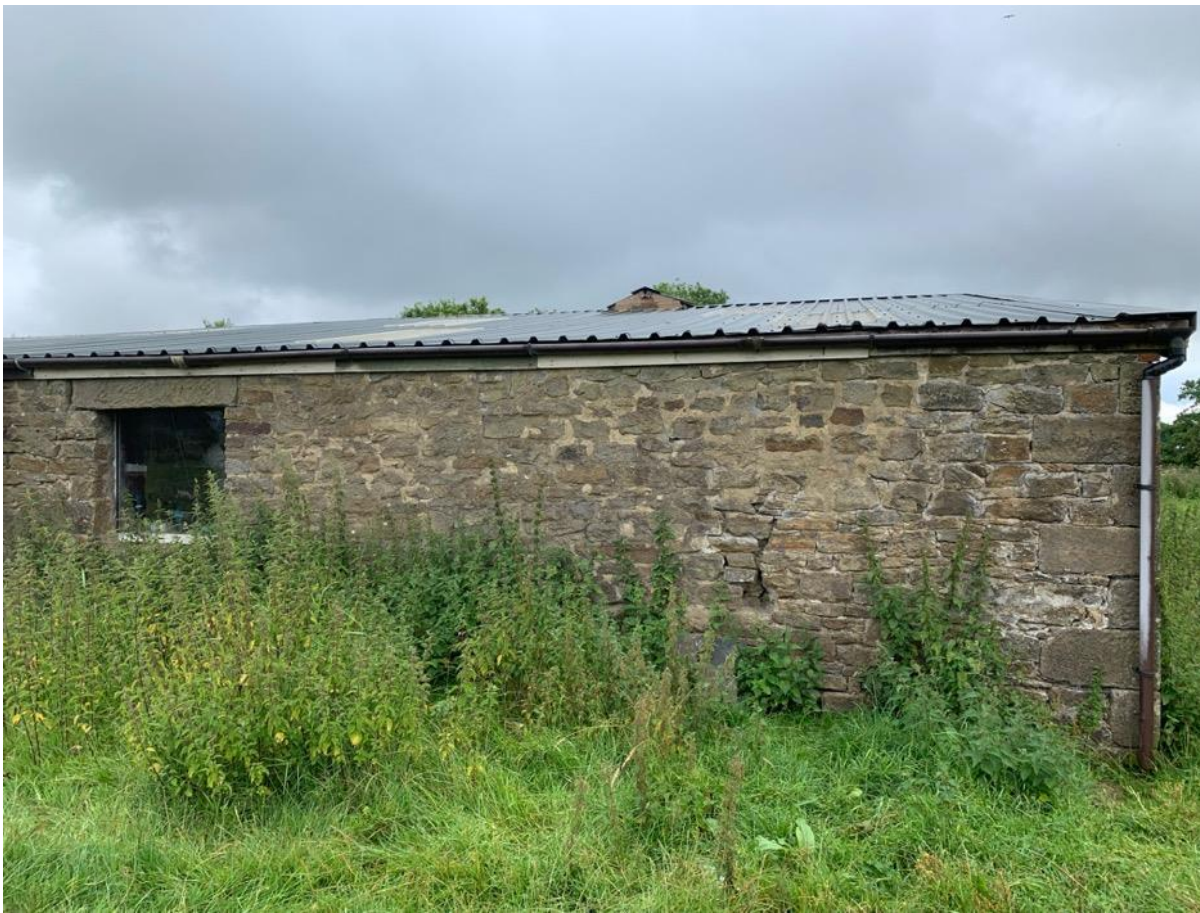
Photo 15 – North Elevation – Stone Section
