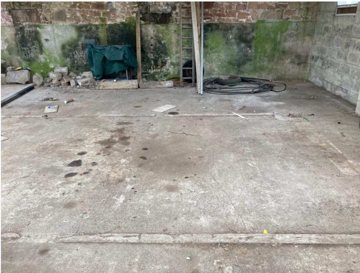
Photo 57 - Internal to newer blockwork building – looking north
