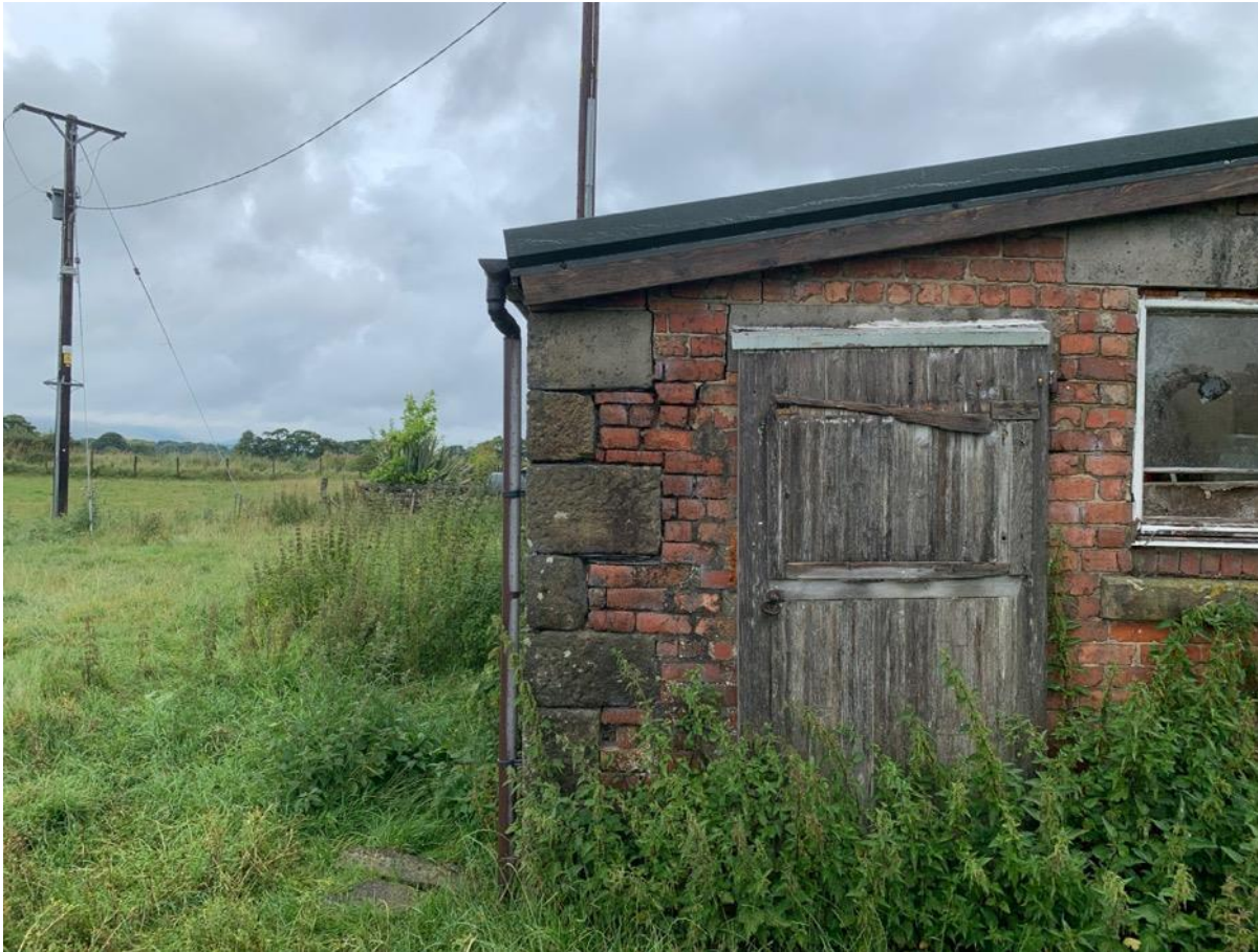
Photo 14 - West elevation north end at north west corner
