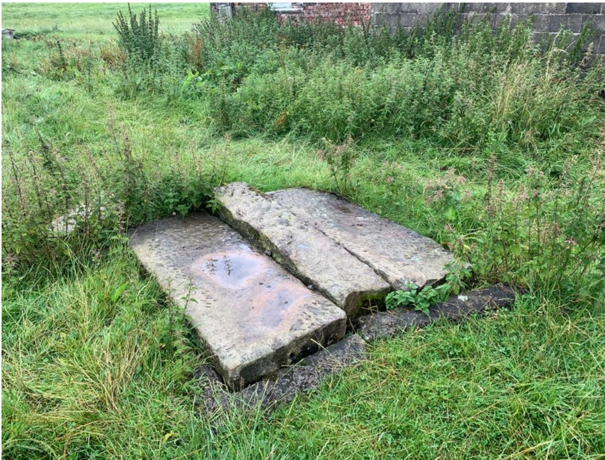
Photo 9 – Tank or manhole adjacent to west elevation
