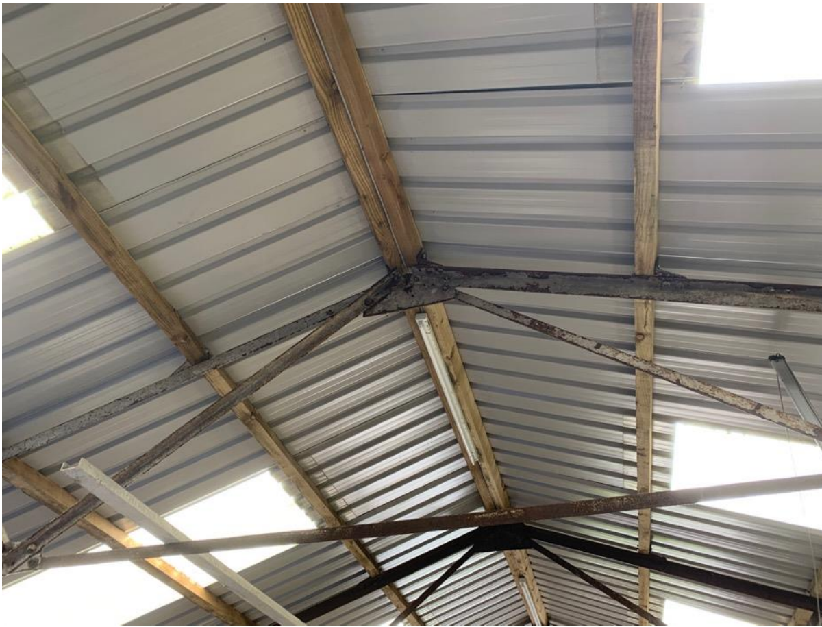
Photo 55 - Internal to newer blockwork building – roof
