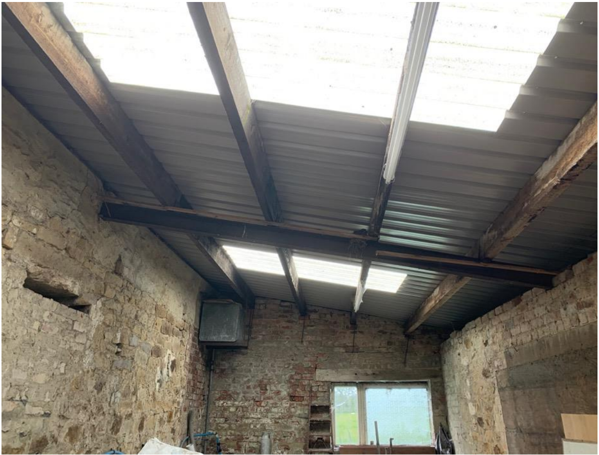
Photo 41 - Internal to original building
