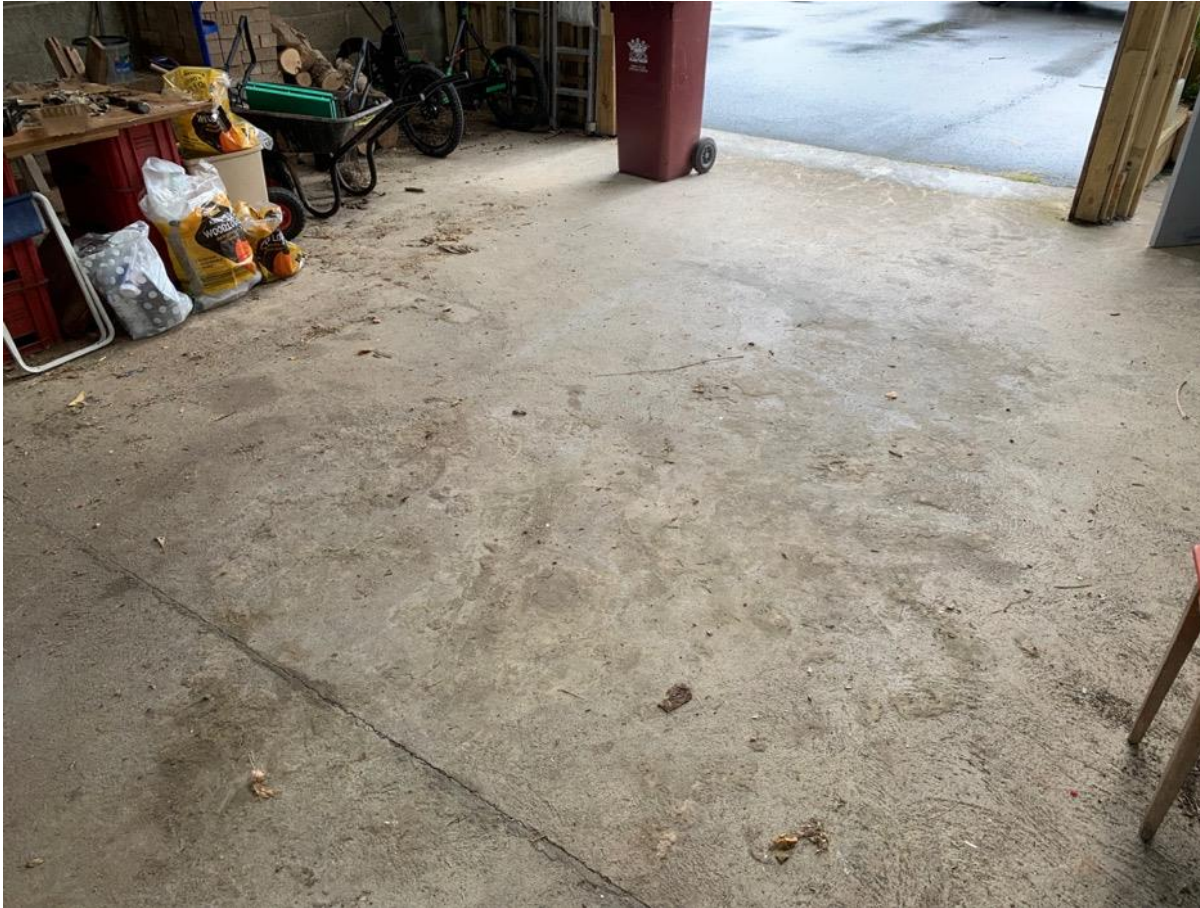
Photo 39 - Internal to extension of original building – concrete floor
