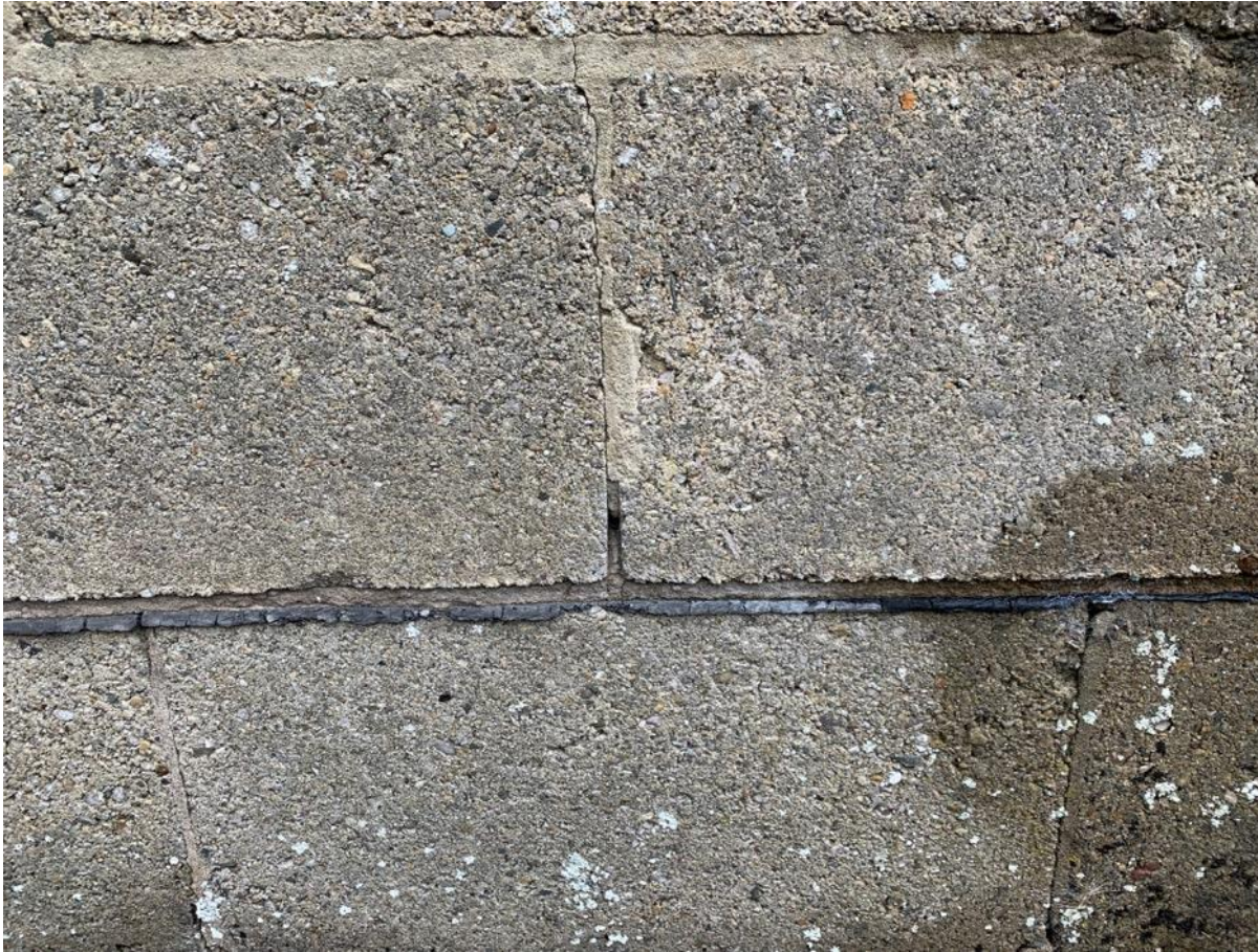
Photo 4 – South Elevation DPC
