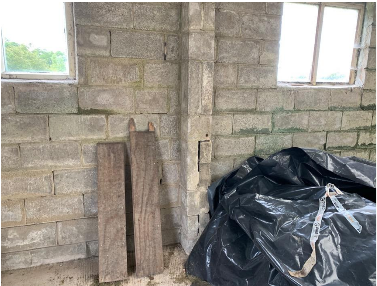
Photo 46 - Internal to newer blockwork building – block pier
