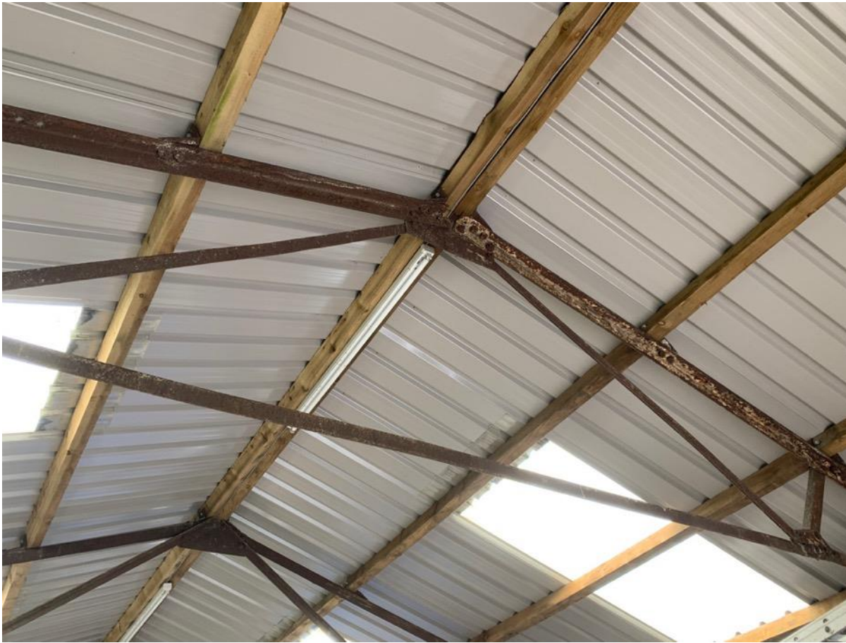
Photo 48 - Internal to newer blockwork building – roof truss and purlins
