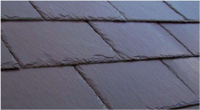
PL14: Example of natural slate roofing.
