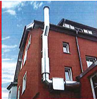
Outdoor installation with wall bracket (accessories).
