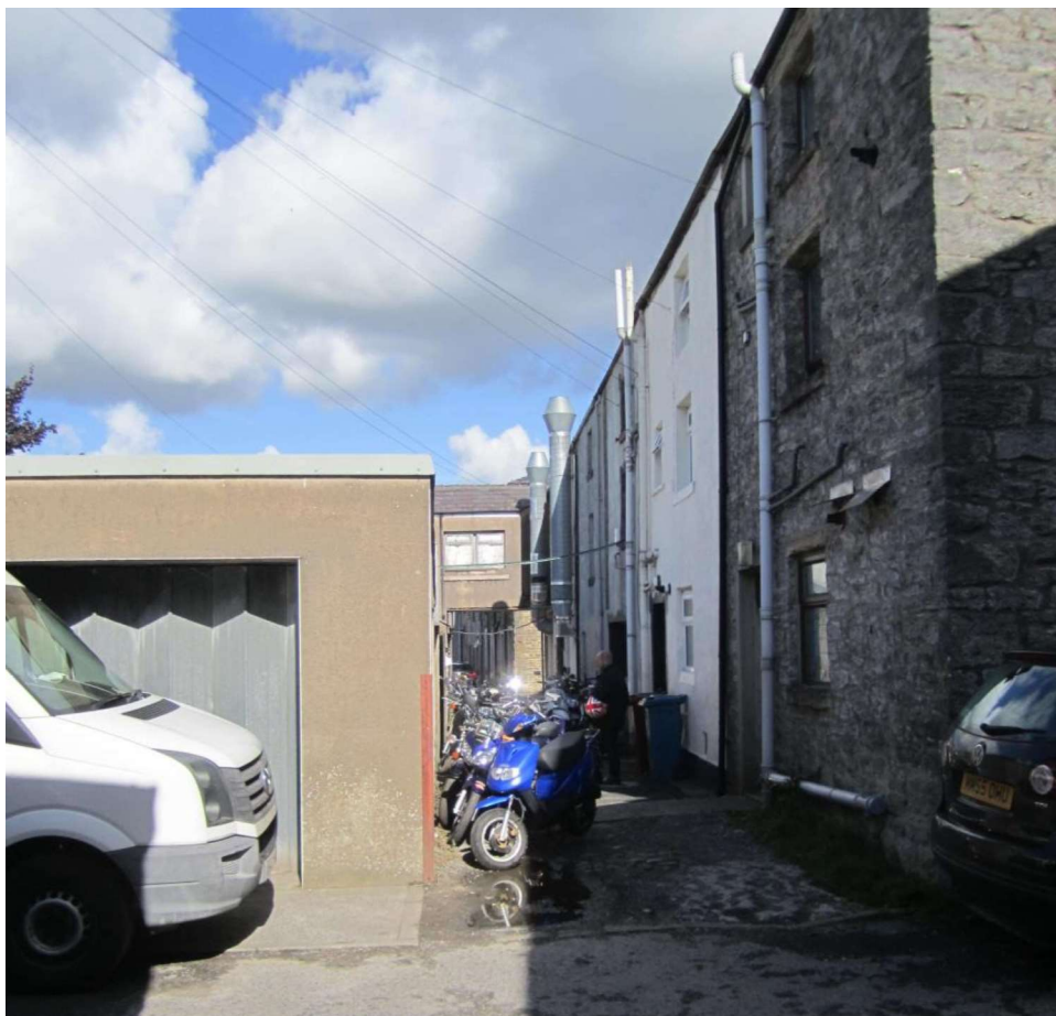
Extraction equipment at the rear of 48 and 50 Whalley Road
