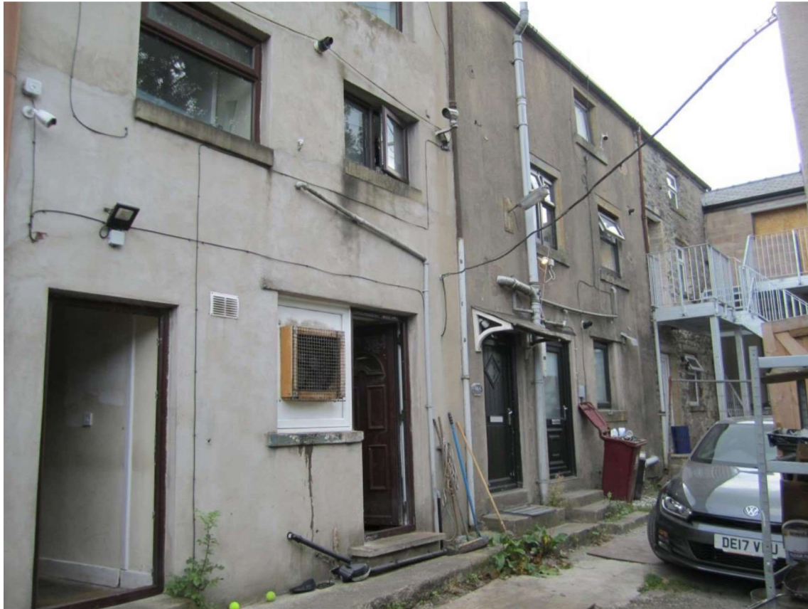
Rear Elevations (66 Whalley Road).
