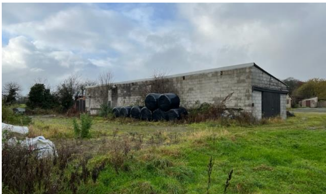
Figure 3: Building subject to appeal.
