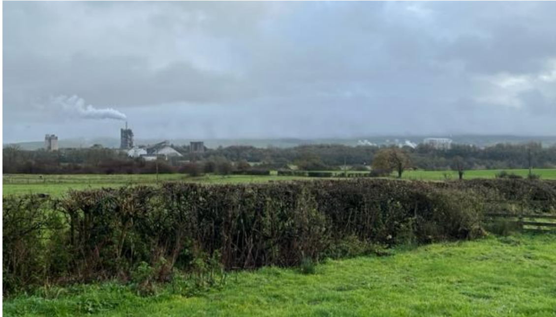
Figure 4: Cement and asphalt works to the south and east of the site.
