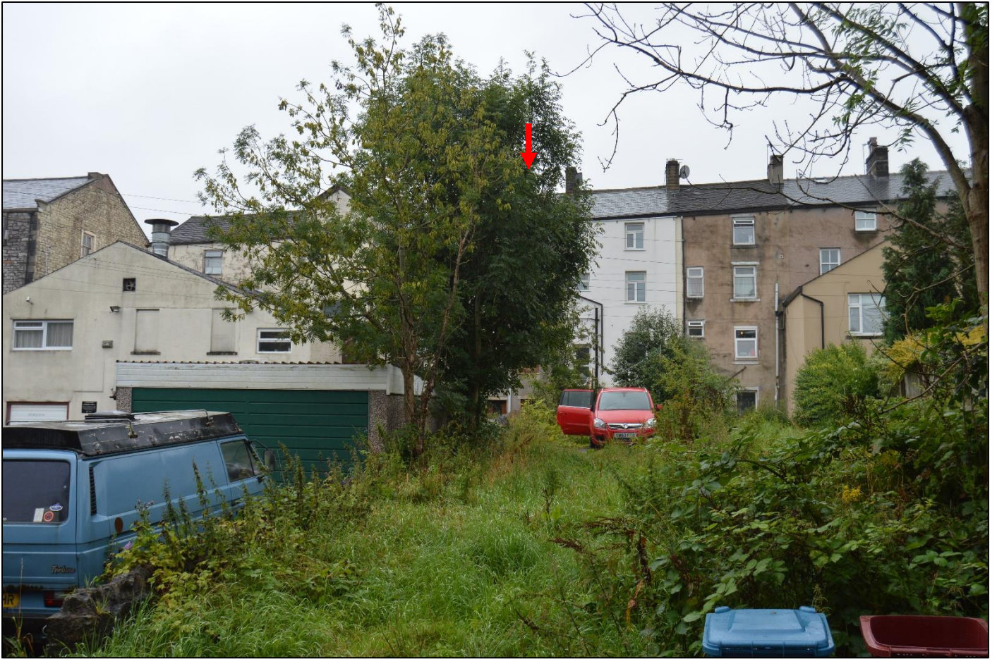
PL03: View of the 84 Whalley Road from the access road to the north west.
