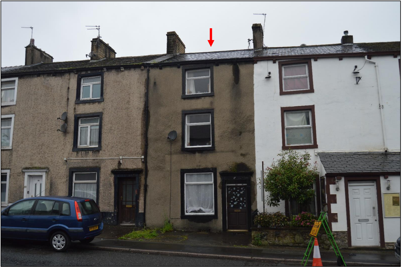
PL01: View of 84 Whalley Road from the south east.
