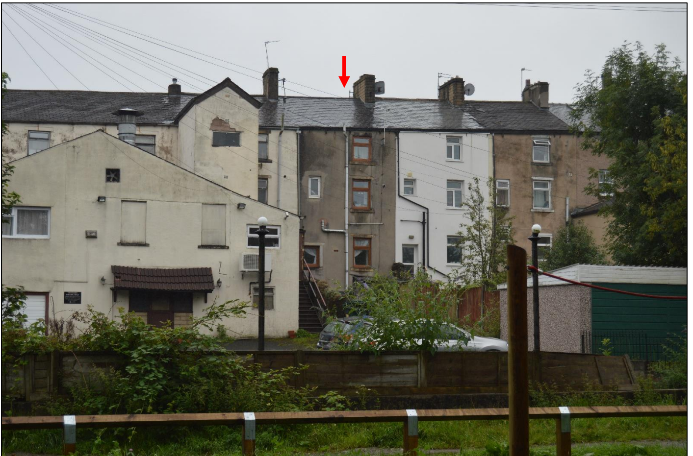
PL02: View of 84 Whalley Road from the north west.
