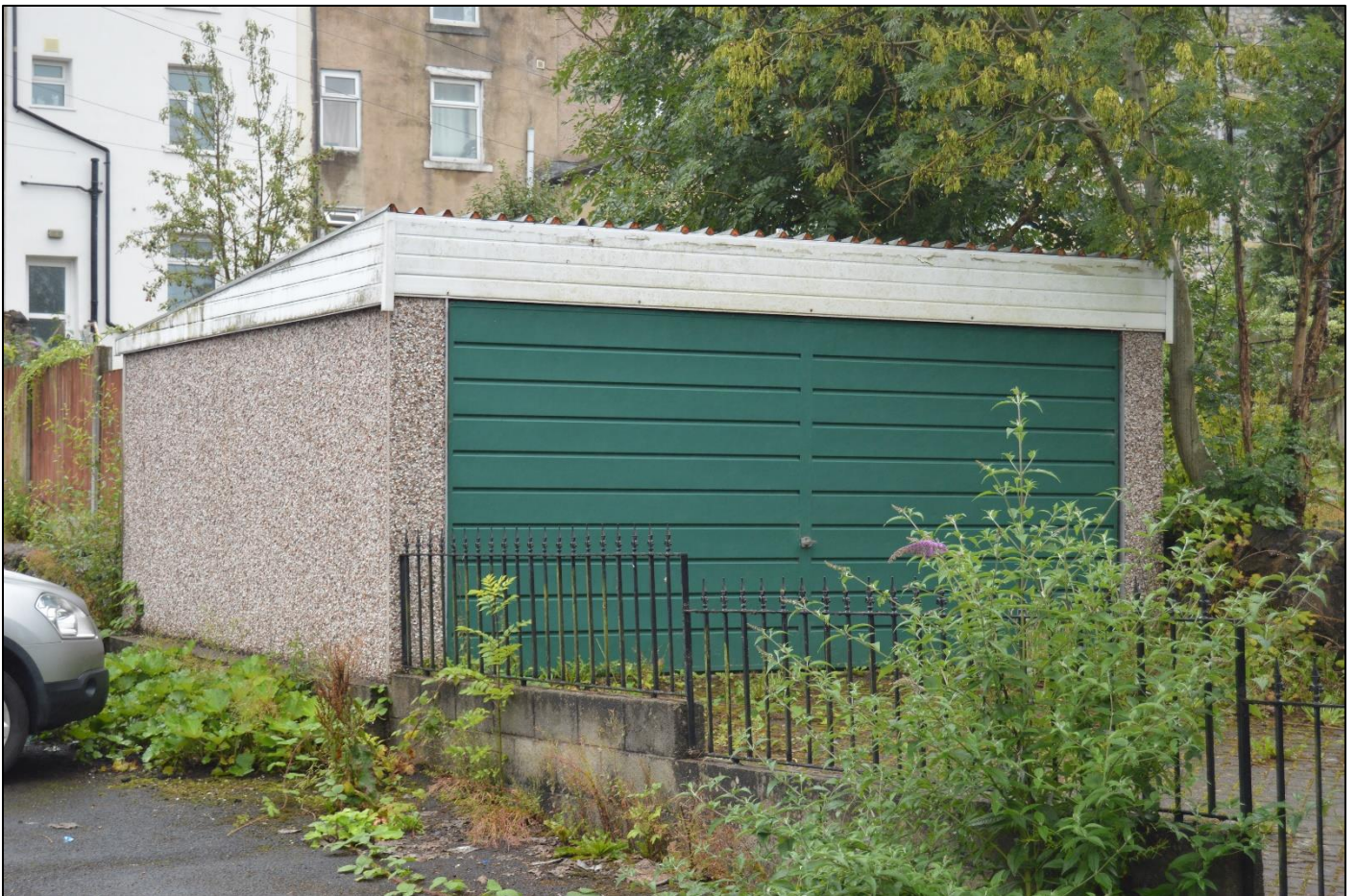
PL04: View of the existing Garage from the north.
