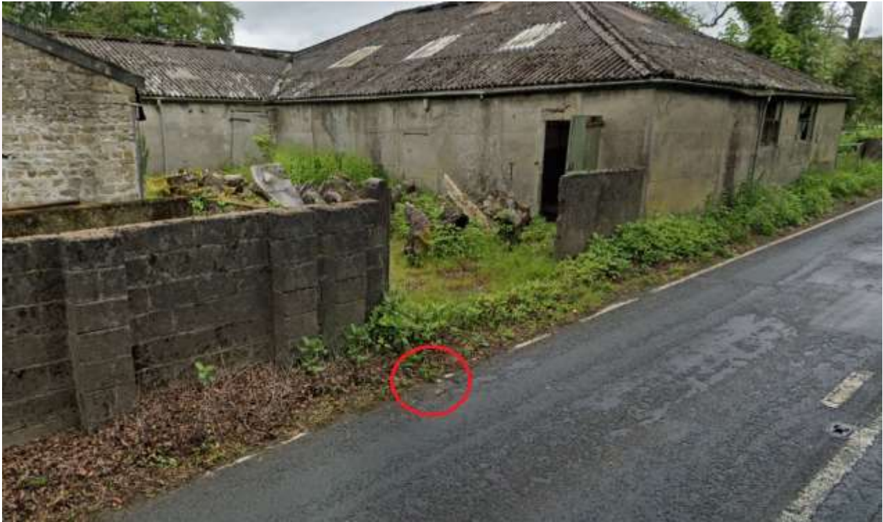
Figure 5: Existing Manhole into culverted watercourse (Google Maps Street View, 2023)
