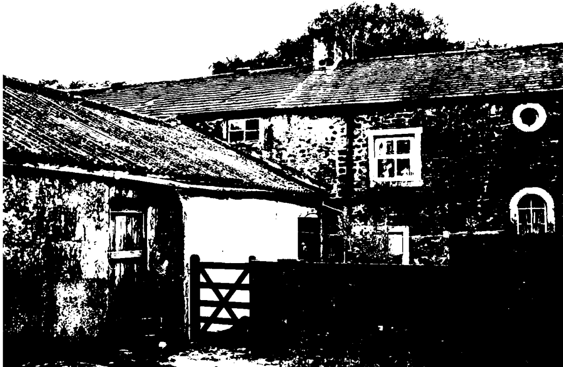
Plate 9. Barn B, north elevation, property boundary with farmhouse is indicated by change in roof covering between Welsh slate over farmhouse and stone slabs over barn.
