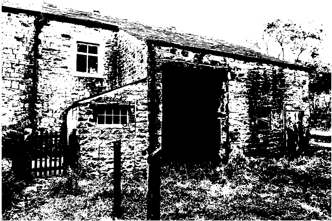
Plate 4. Barn B, south elevation, viewed from south-west.
