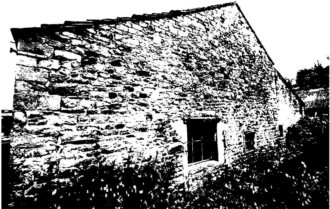
Plate 7. Barn B, east elevation, viewed from south-east.
