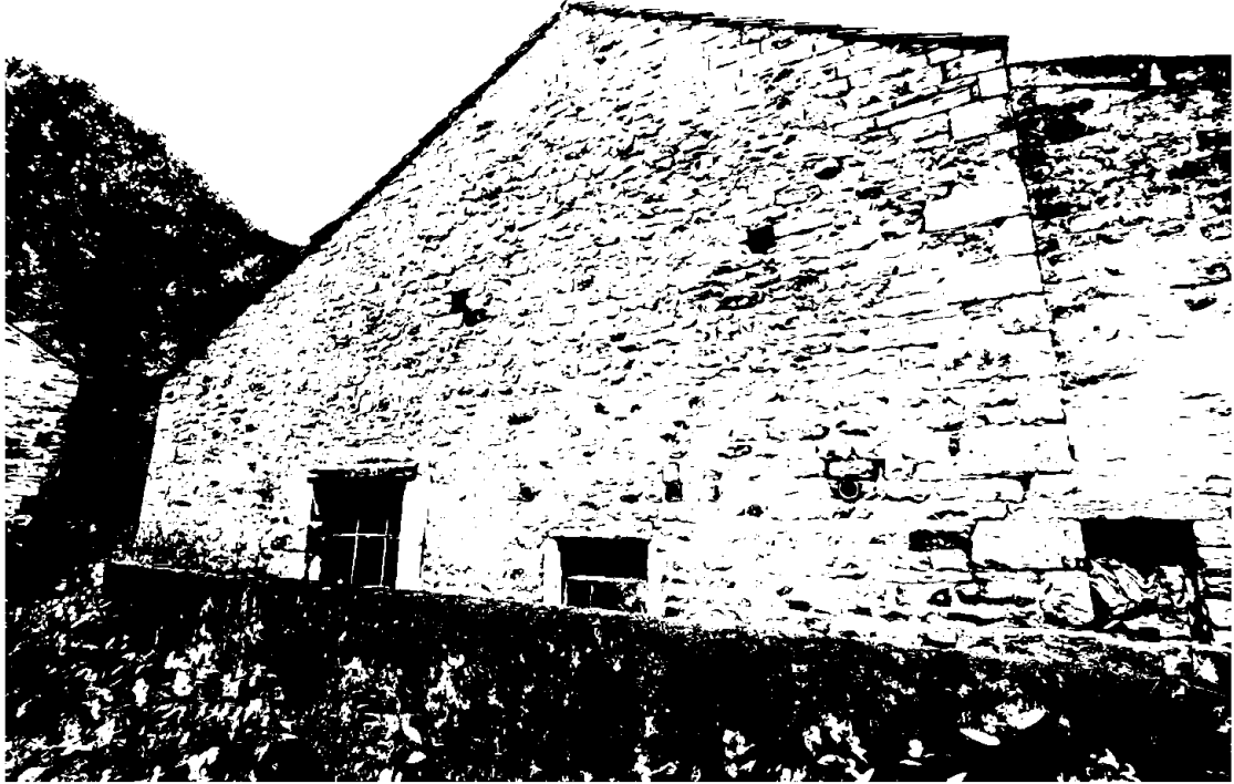
Plate 6. Barn B, east elevation, viewed from north-east.
