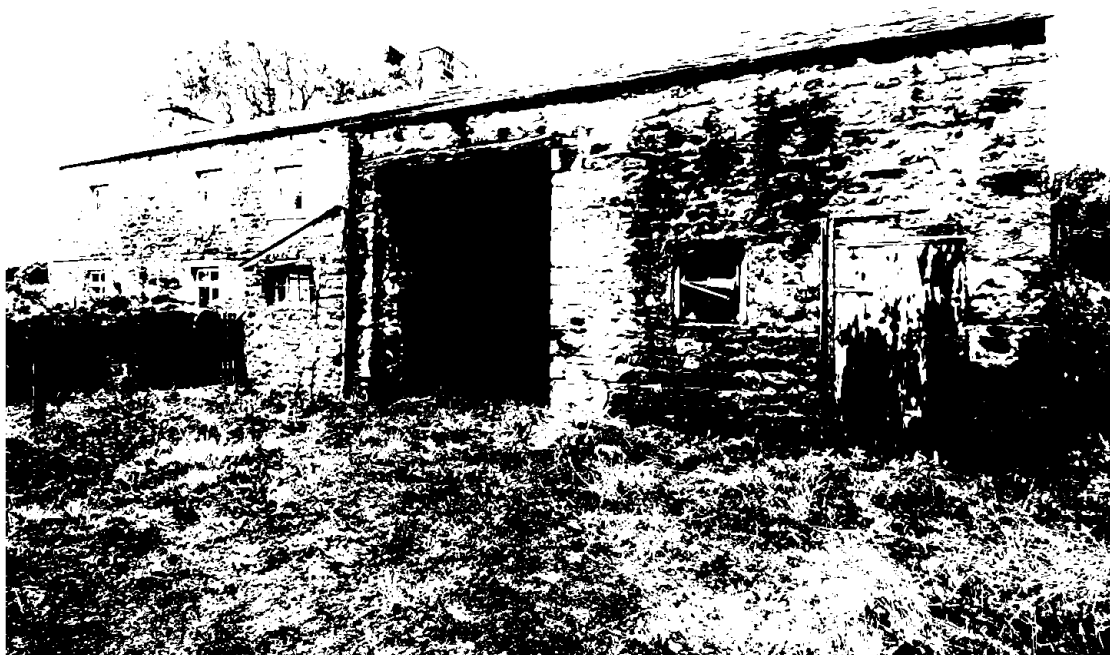
Plate 1. Barn B, south elevation, with farmhouse to left, viewed from south-east.
