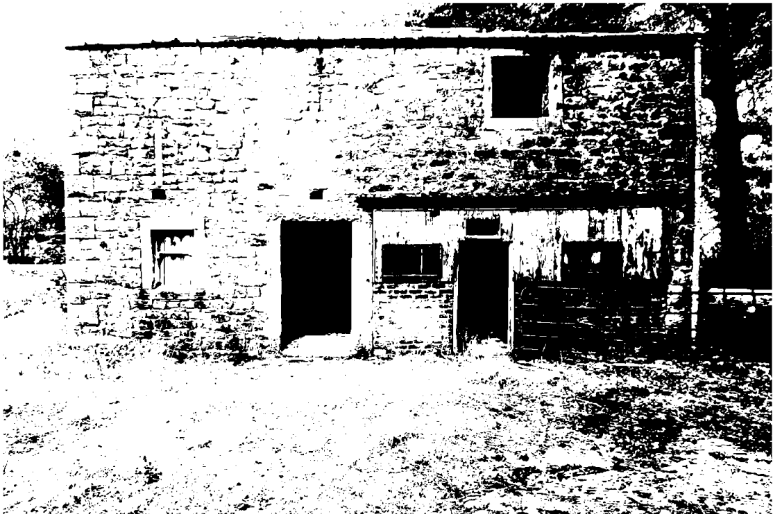
Plate 32. Barn A, west elevation, viewed from west.
