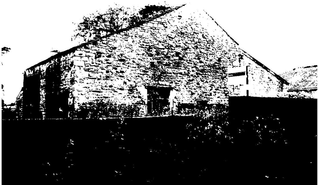
Plate 5. Barn B, east elevation, viewed from Slaidburn Road, from south-east.
