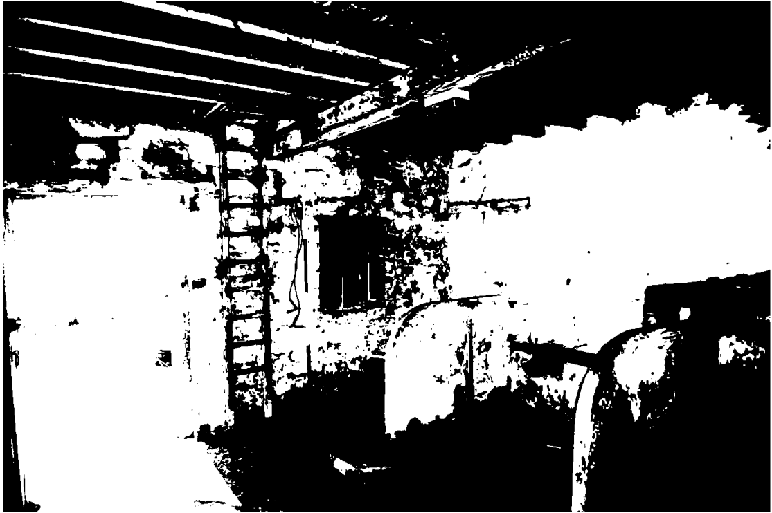
Plate 36. Barn A, bay 2, viewed from south-east, Jacob's Ladder to left of scale.
