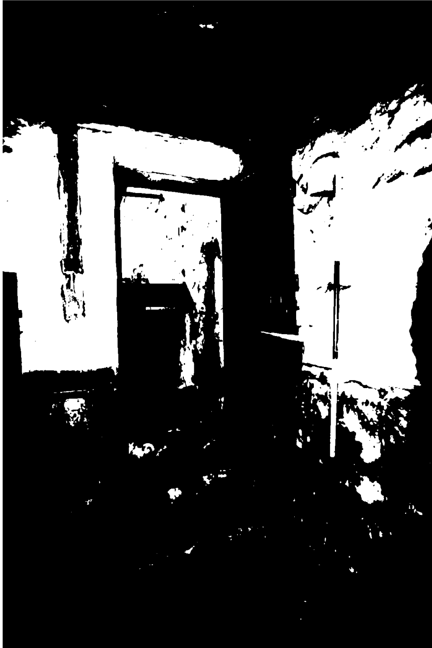
Plate 21. Barn, bay 3, doorway at north end, viewed from south.
