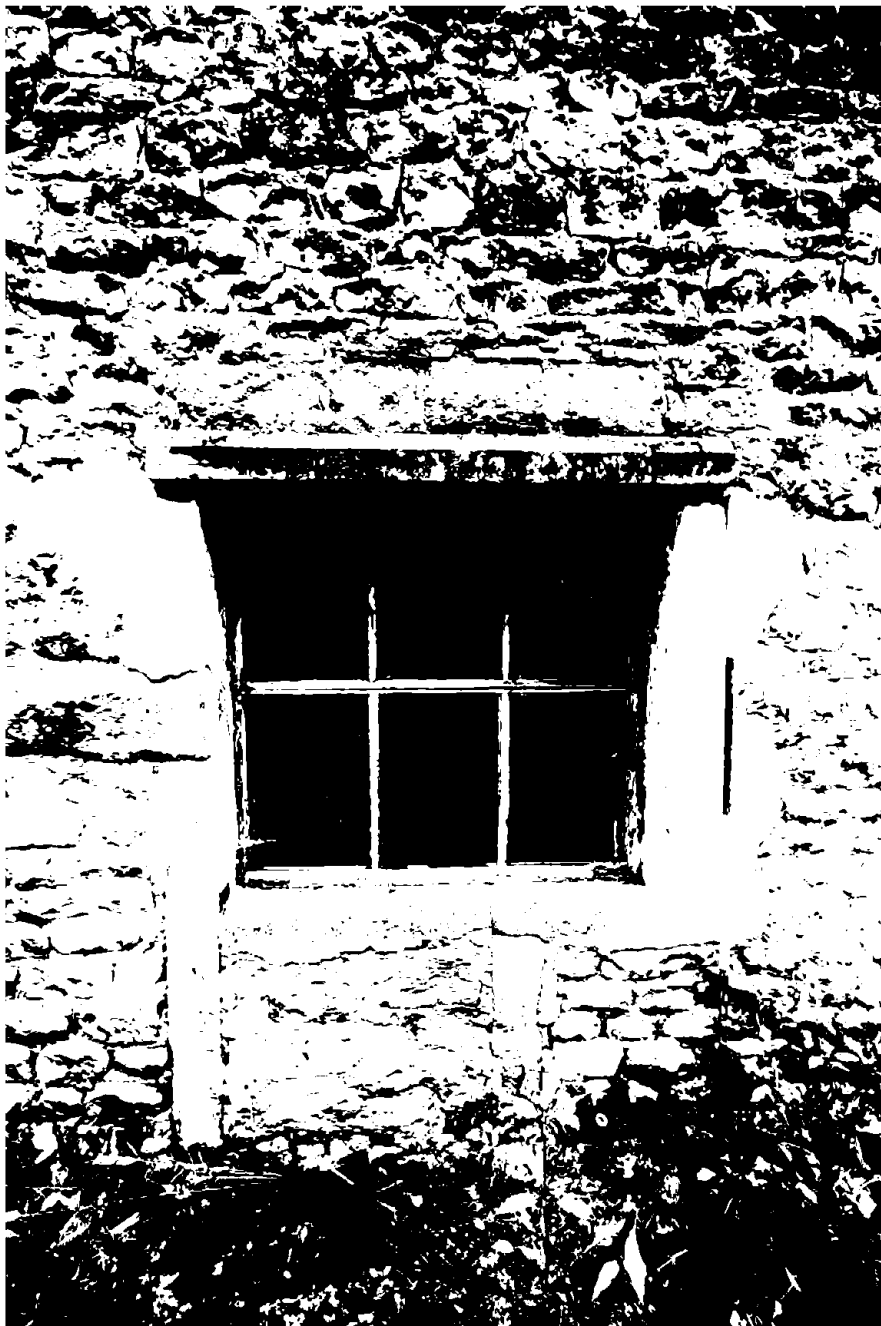
Plate 8. Barn B, east elevation, blocked doorway replaced by window, viewed from east.
