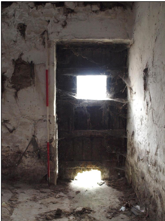
Plate 50: Doorway in south end of east gable
