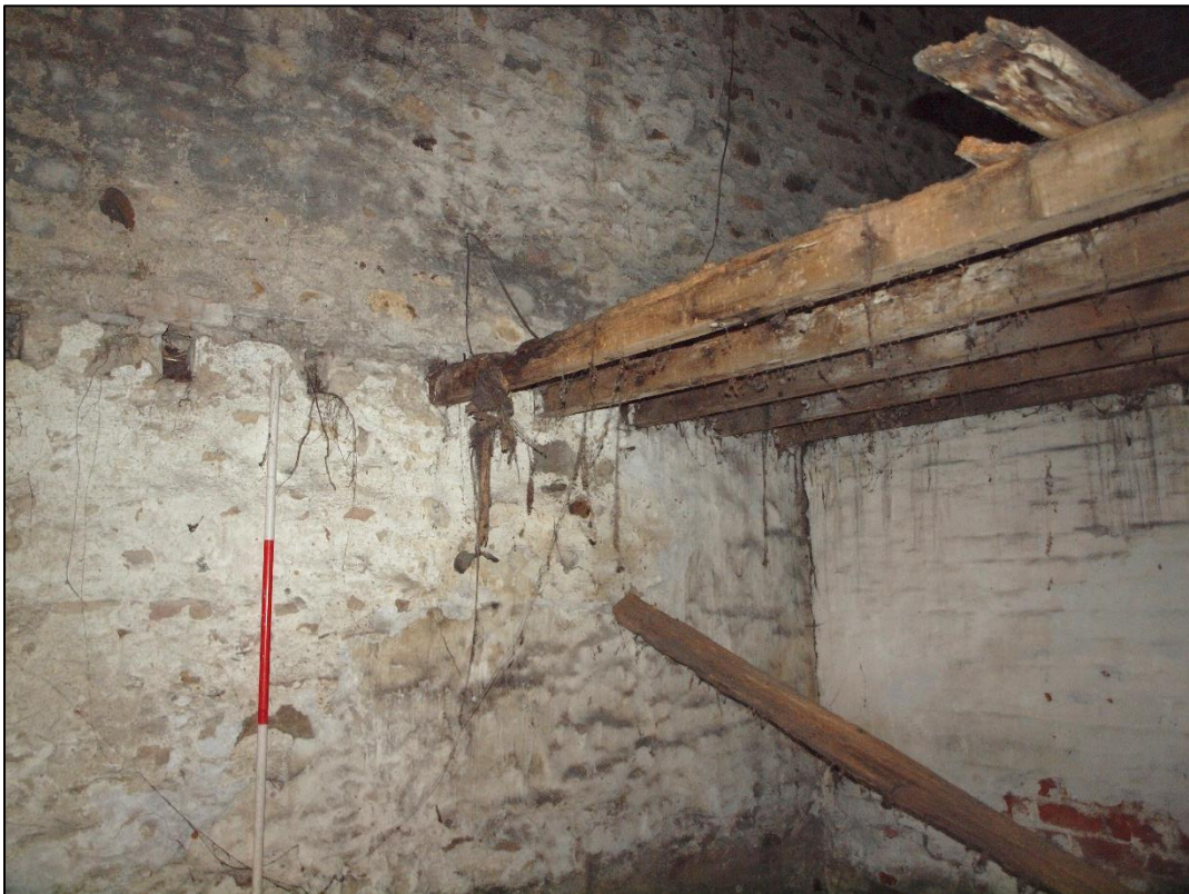
Plate 72: Joist holes and remaining first floor
