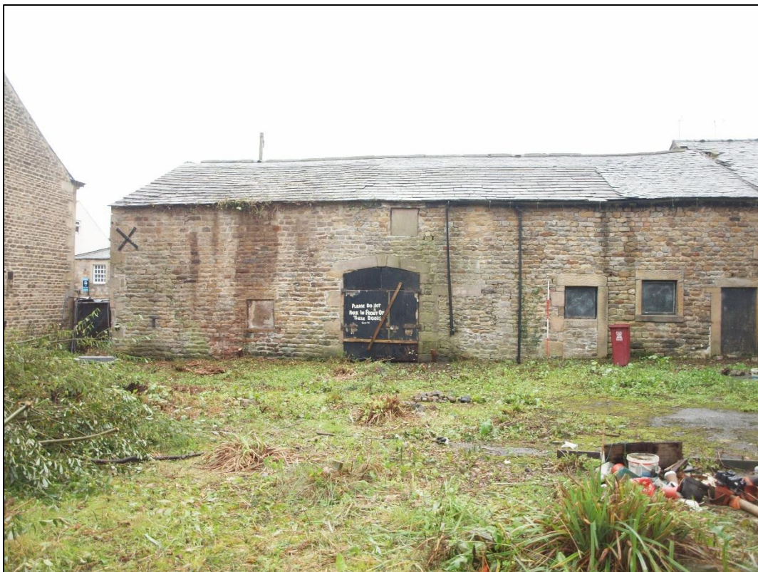
Plate 20: Eastern end of north elevation
