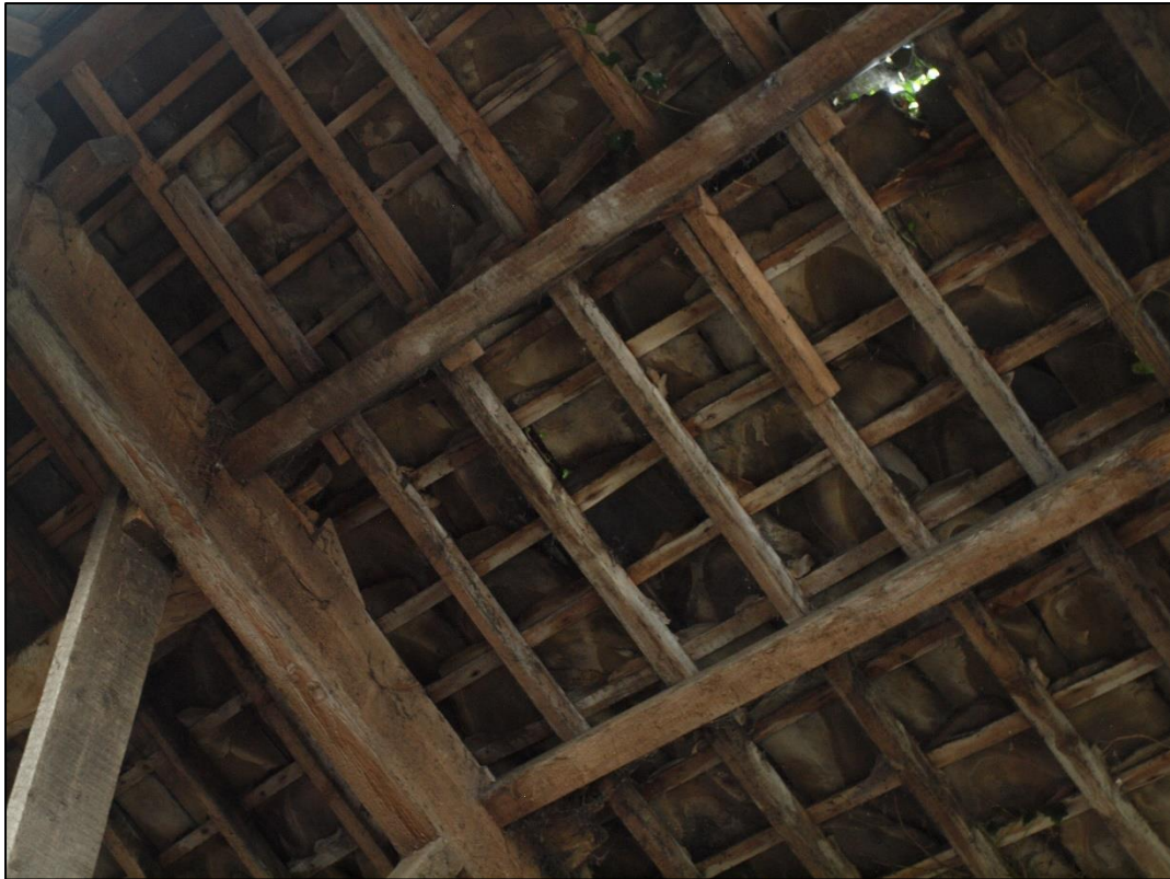
Plate 49: Detail of roof structure
