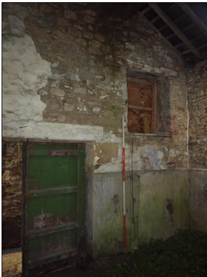
Plate 78: Doorway with pitching eye over in west wall
