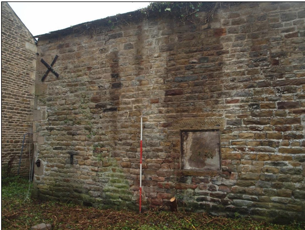
Plate 22: Eastern end of north elevation
