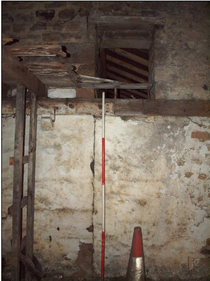
Plate 73: Straight joint of original corner of barn
