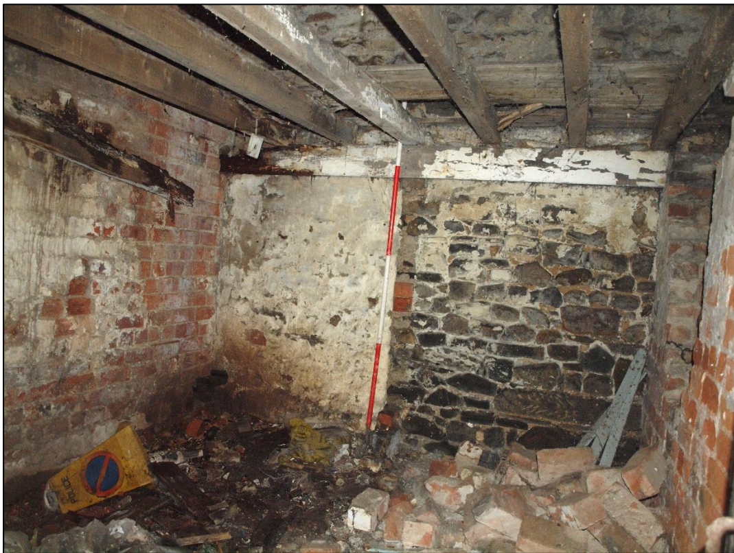
Plate 76: Central room of extension showing scar of removed brick wall
