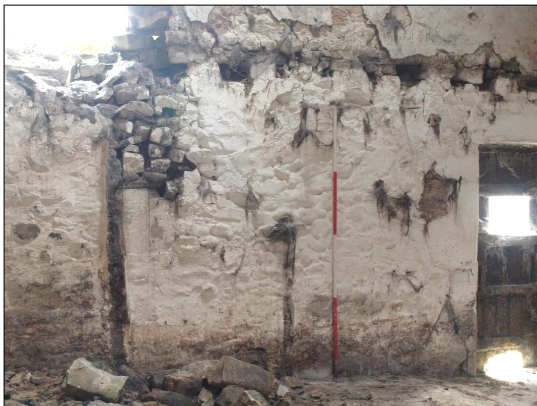
Plate 45: Scars of removed stalls in gable
