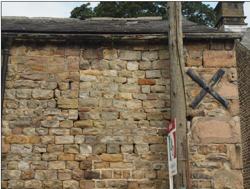
Plate 14: Blocked window at first floor level
