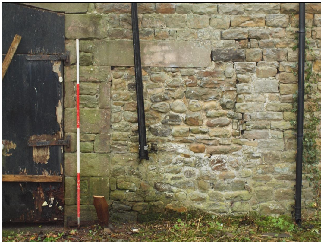
Plate 26: Detail of blocked doorway
