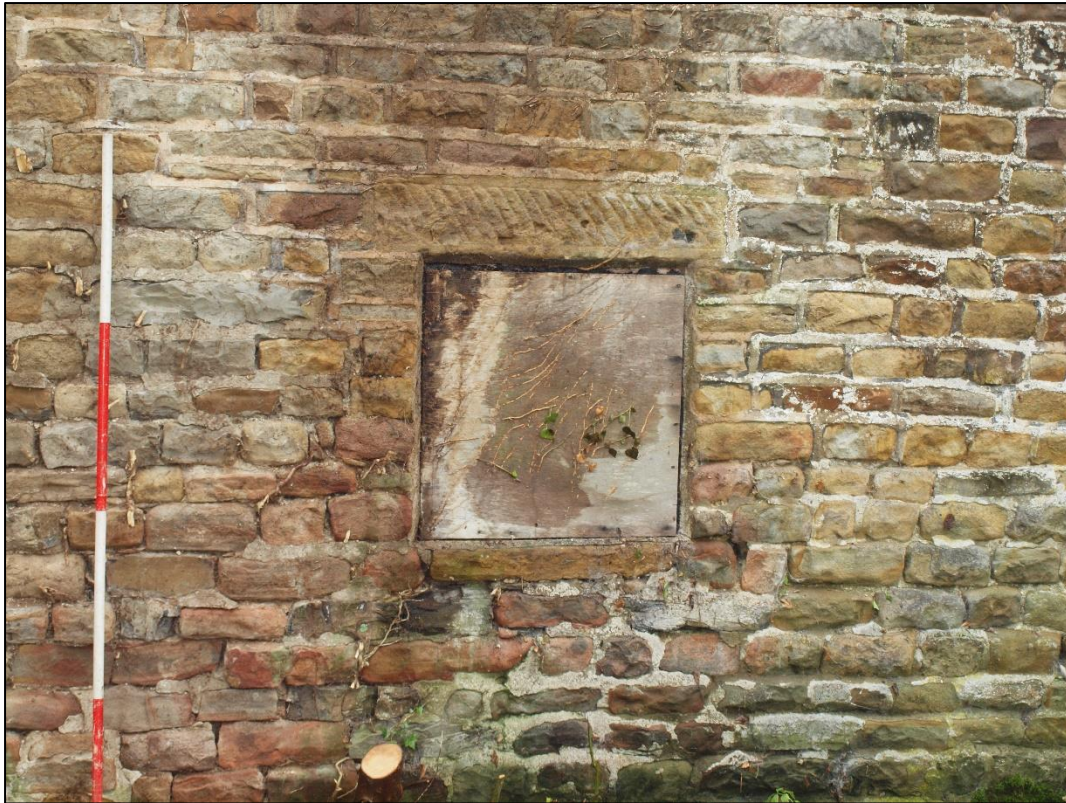
Plate 23: Detail of window shown above
