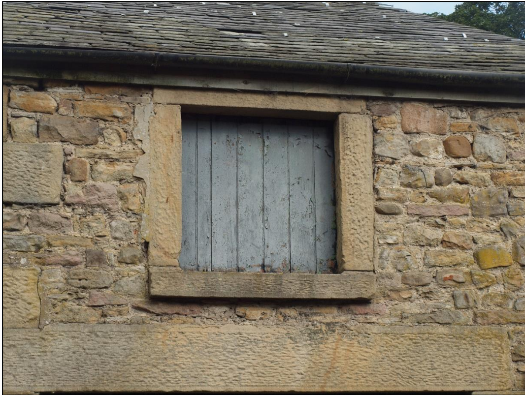
Plate 7: Pitching eye detail
