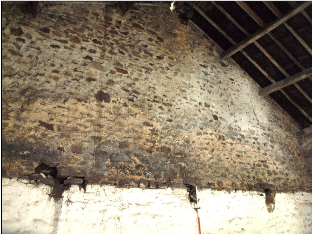
Plate 59: Detail of removed first floor joist holes and first floor of gable
