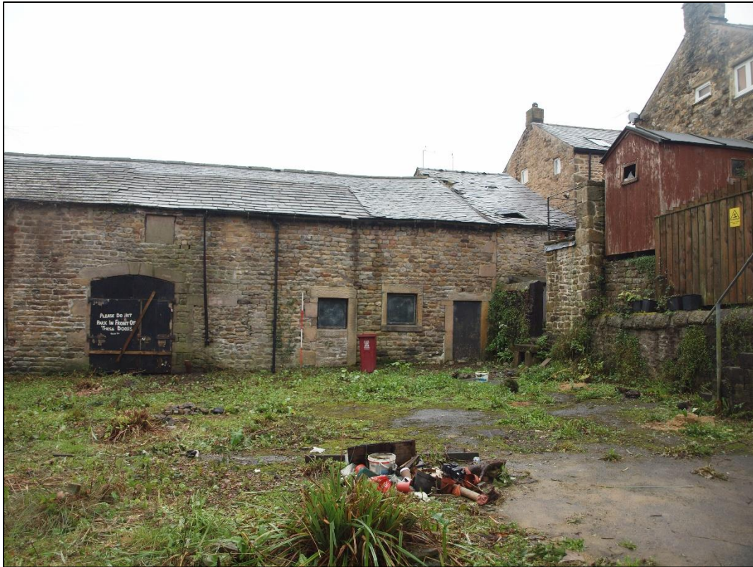
Plate 21: Western end of north elevation
