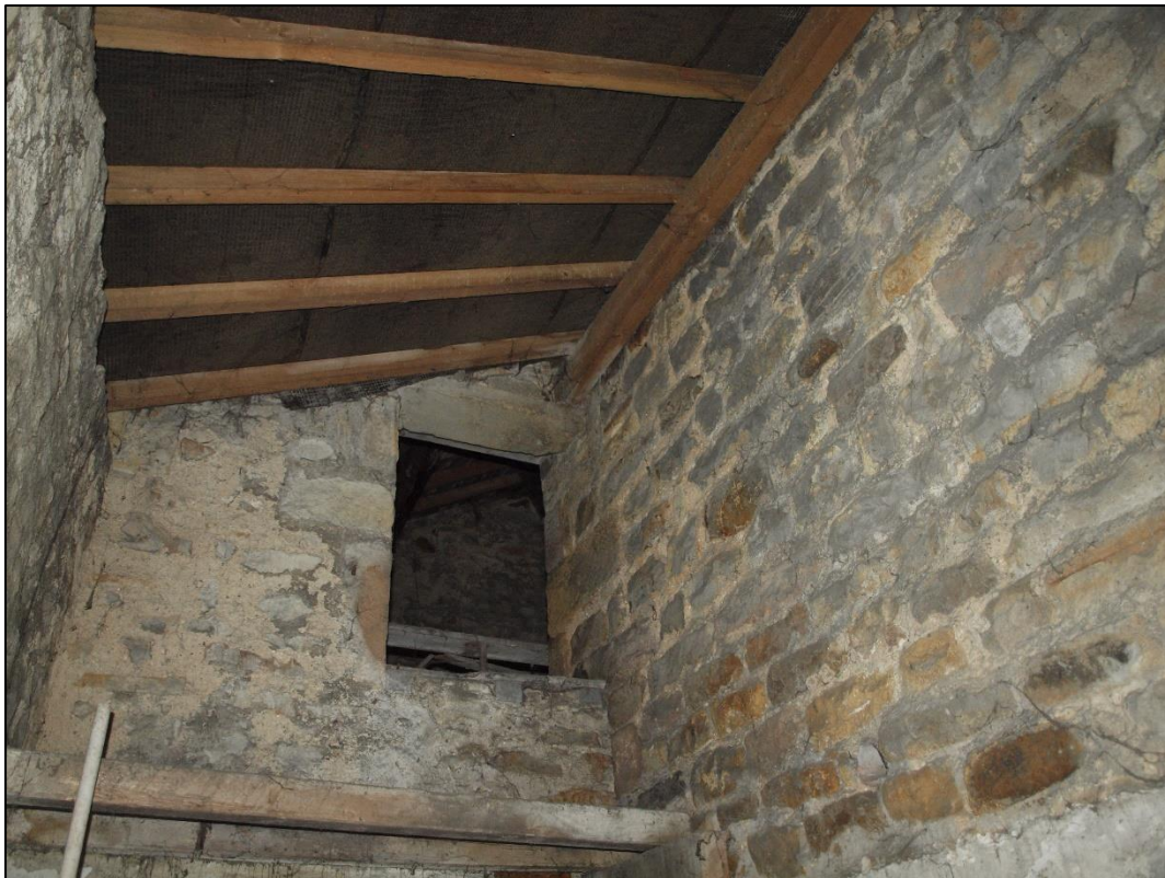
Plate 66: Opening to extension
