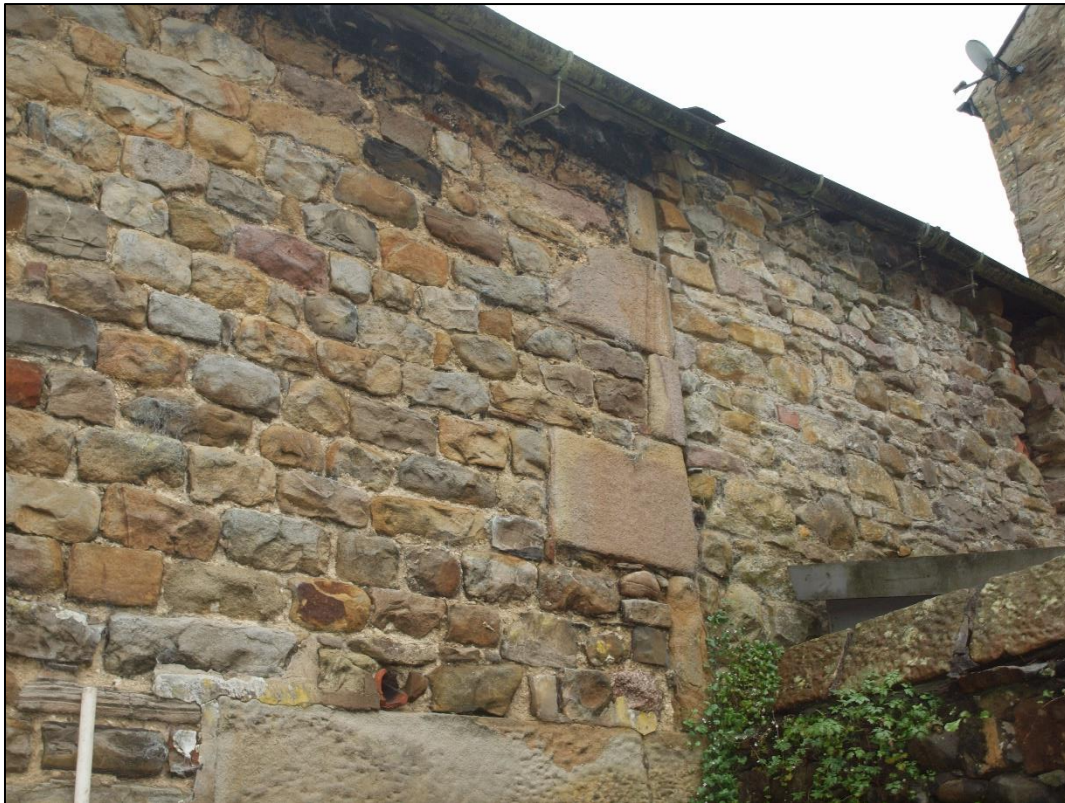
Plate 31: Straight joint with quoins marking end of original barn
