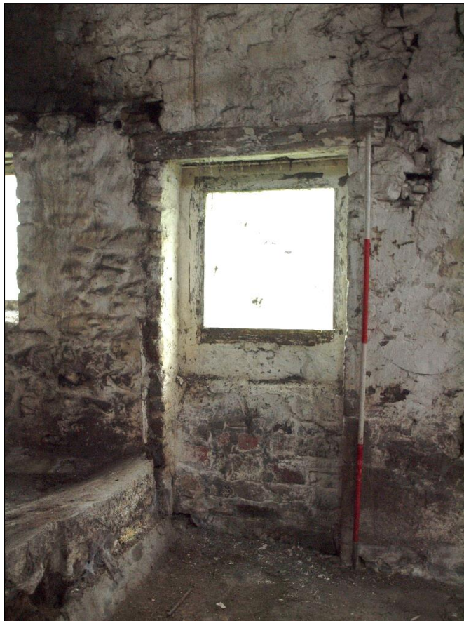
Plate 55: Blocked doorway with window inserted
