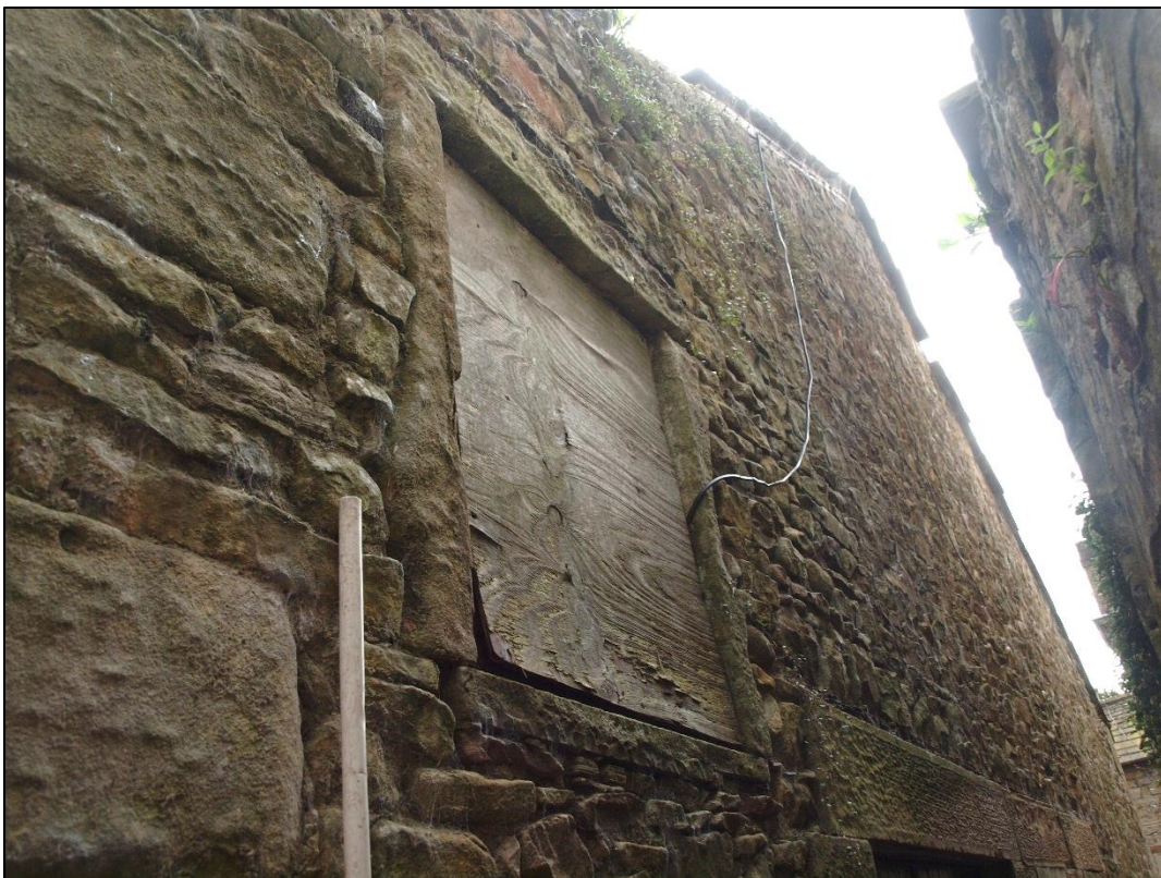
Plate 36: Pitching eye to northern end
