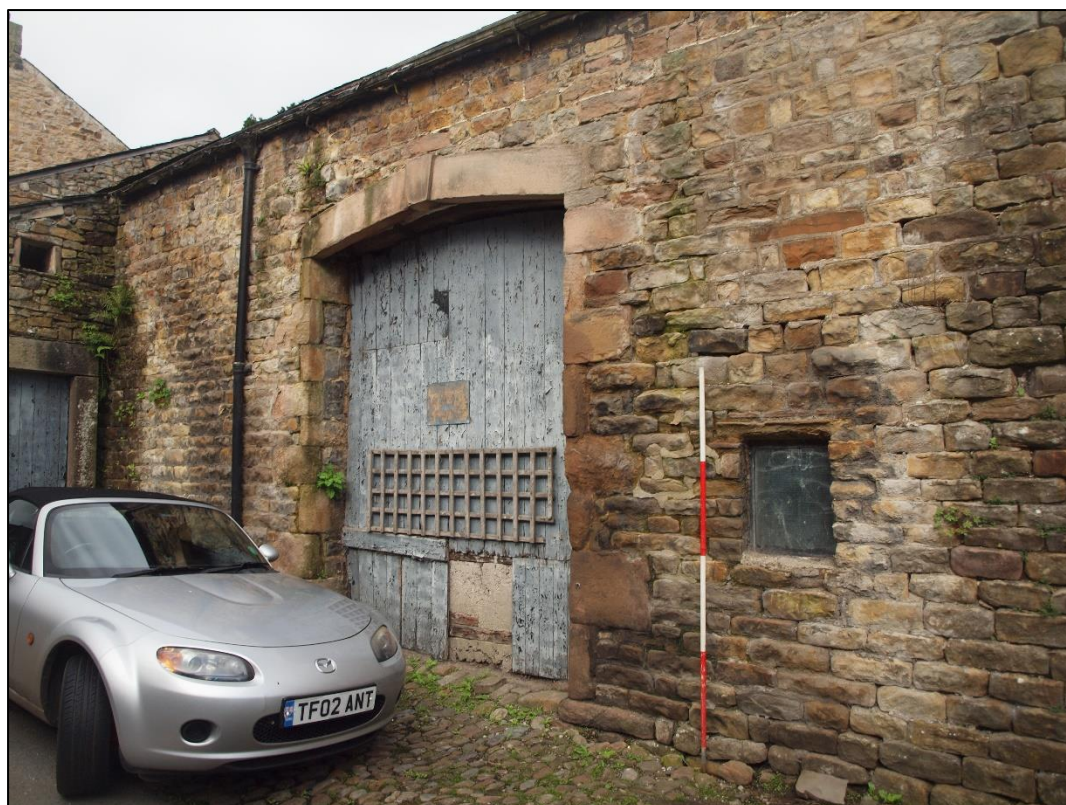
Plate 9: East end of south elevation showing barn door and window
