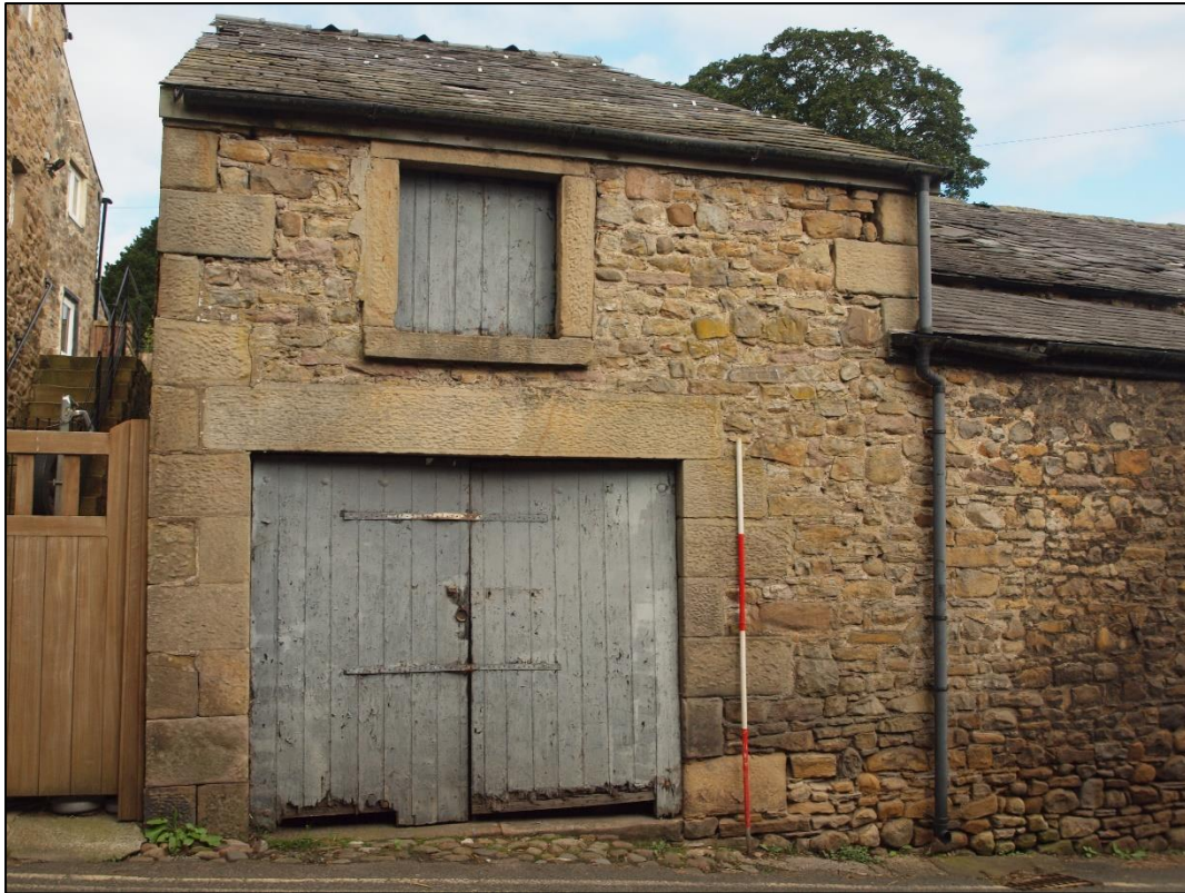
Plate 5: Loading doorway with pitching eye over
