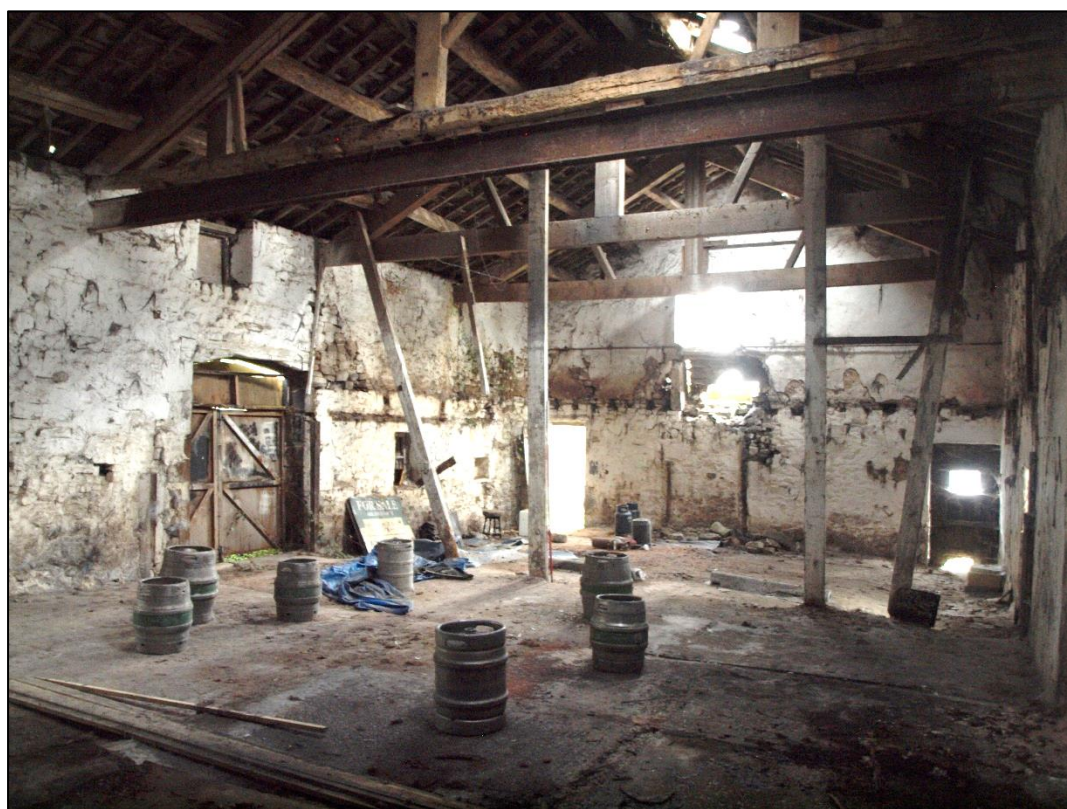
Plate 42: General shot of interior looking east
