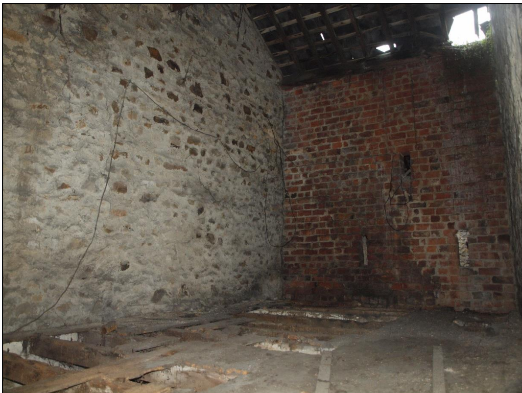
Plate 68: First floor of extension showing brick wall
