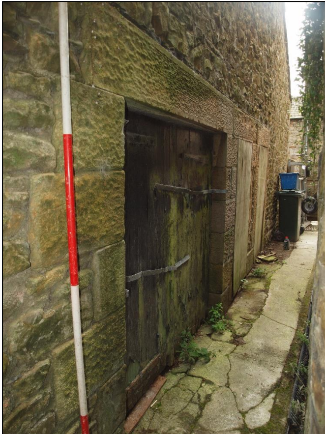
Plate 37: Wide loading doorway at northern end
