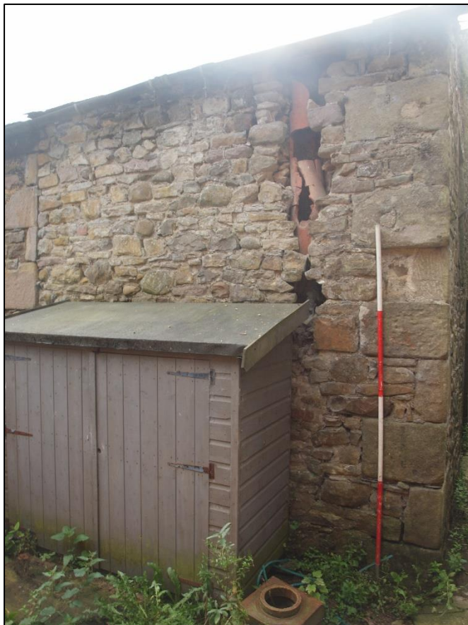
Plate 32: North elevation of extension
