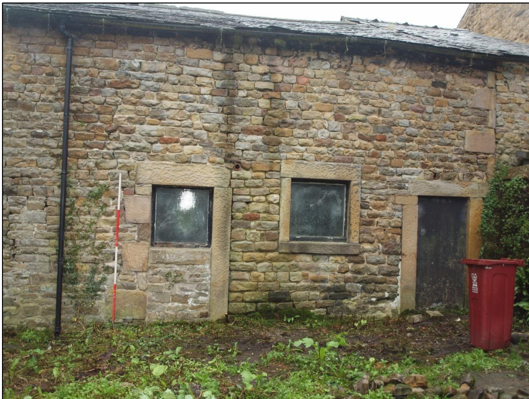
Plate 28: Western end of barn showing three openings
