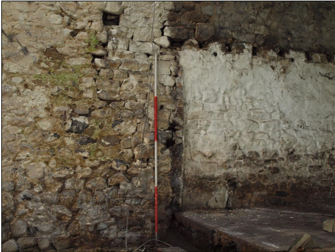
Plate 61: Scar of removed wall to western bay
