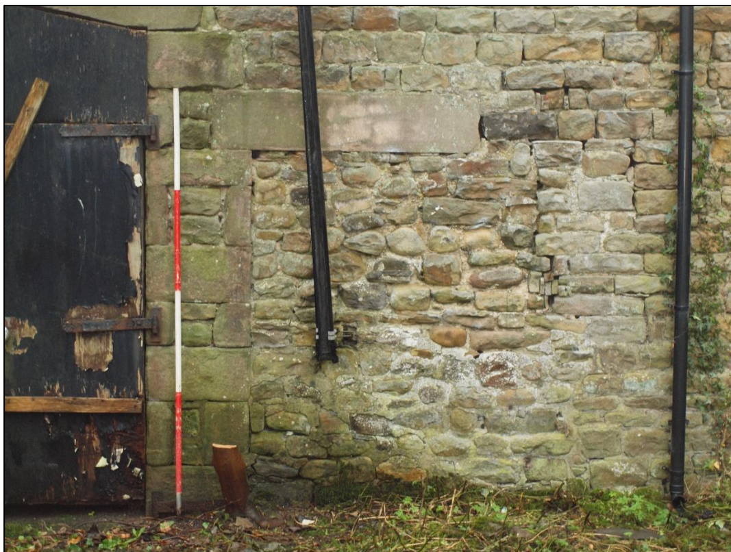
Plate 26: Detail of blocked doorway
