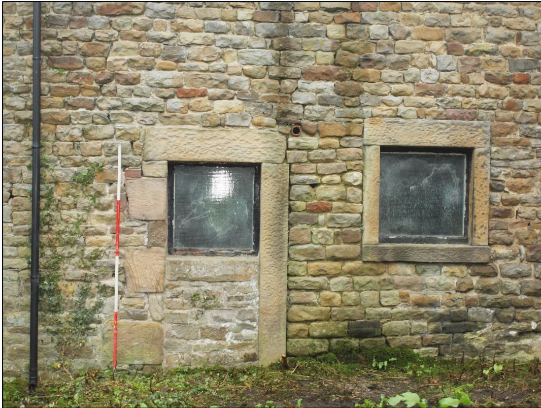
Plate 29: Doorway converted to window and window to the west
