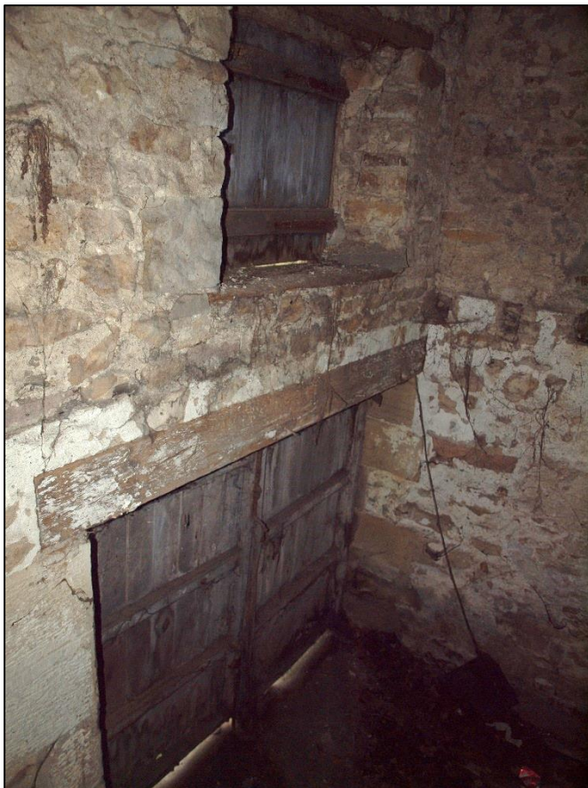
Plate 70: Doorway and pitching eye over in south wall
