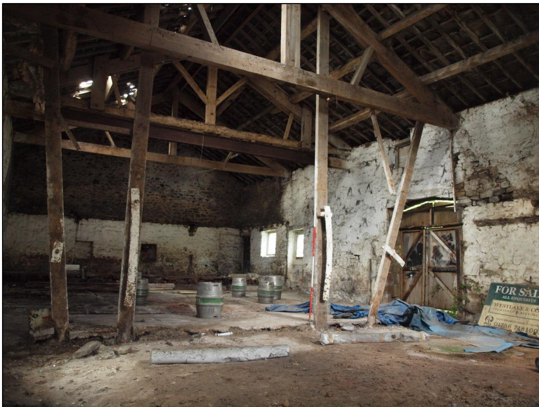
Plate 40: General shot of interior looking west
