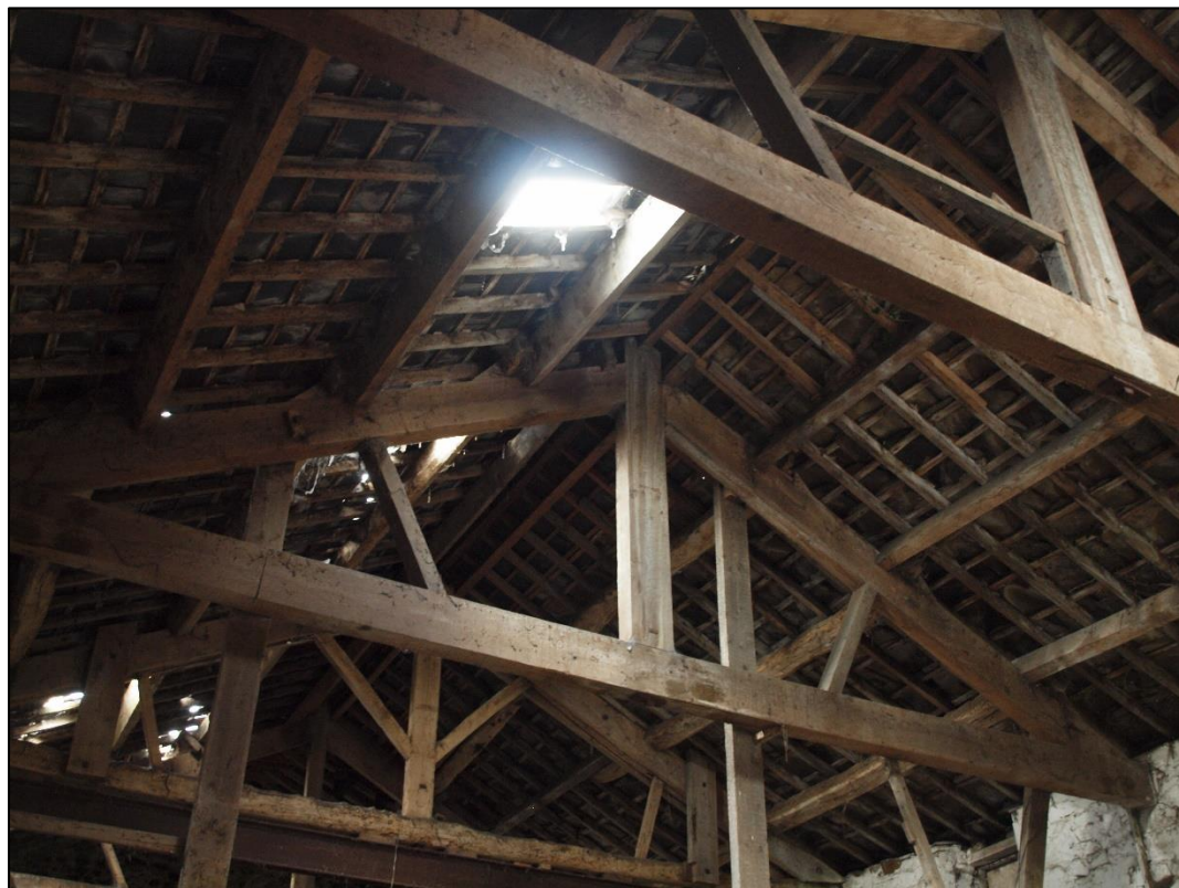
Plate 41: King post trusses
