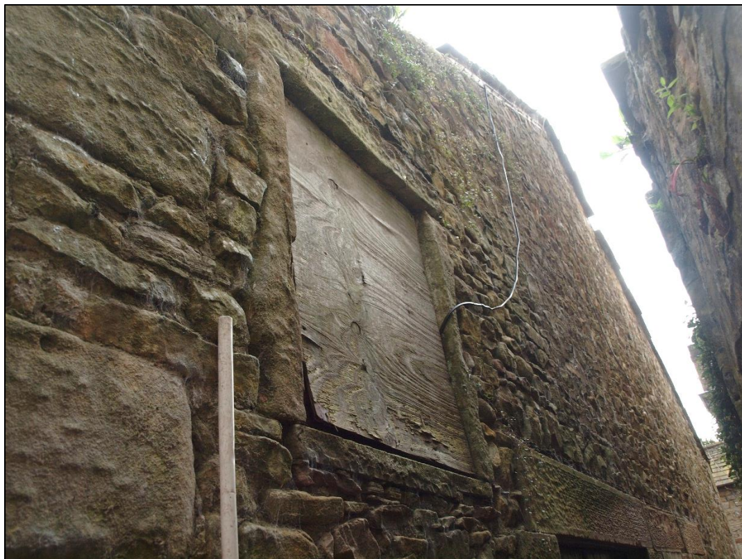
Plate 36: Pitching eye to northern end
