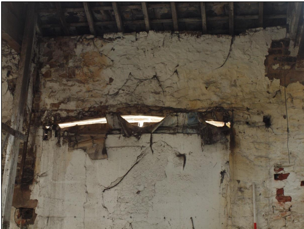
Plate 52: Detail of hand cut timber lintel
