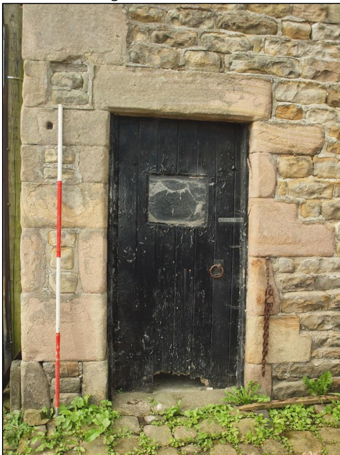
Plate 16: Doorway to southern end of gable
