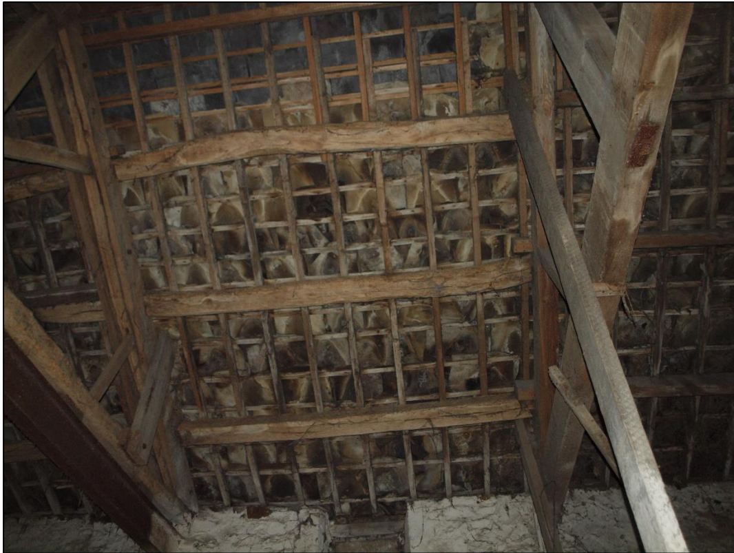
Plate 63: Roof showing remaining hand cut purlins
