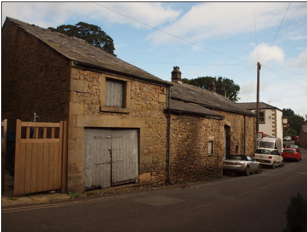
Plate 2: Western end of south elevation
