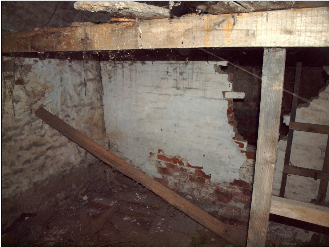
Plate 69: Ground floor looking north
