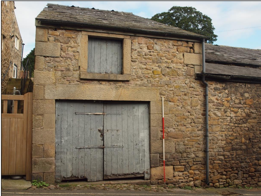
Plate 5: Loading doorway with pitching eye over
