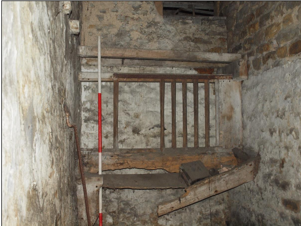
Plate 65: Detail of timber feeding trough
