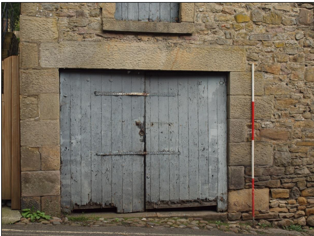
Plate 6: Loading door detail
