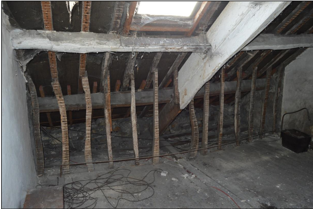
Plate 75: Interior shot c. 2011 prior to strip out (courtesy LCC)
