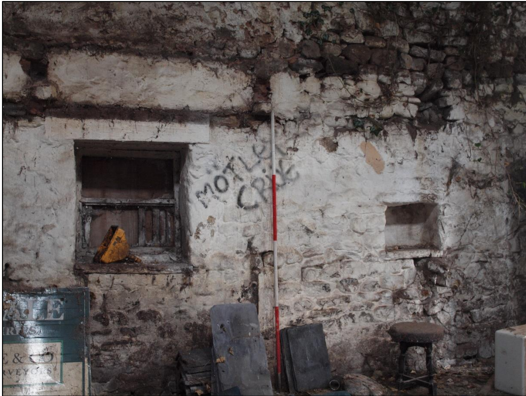
Plate 43: Eastern end of north wall showing window and adjacent niche
