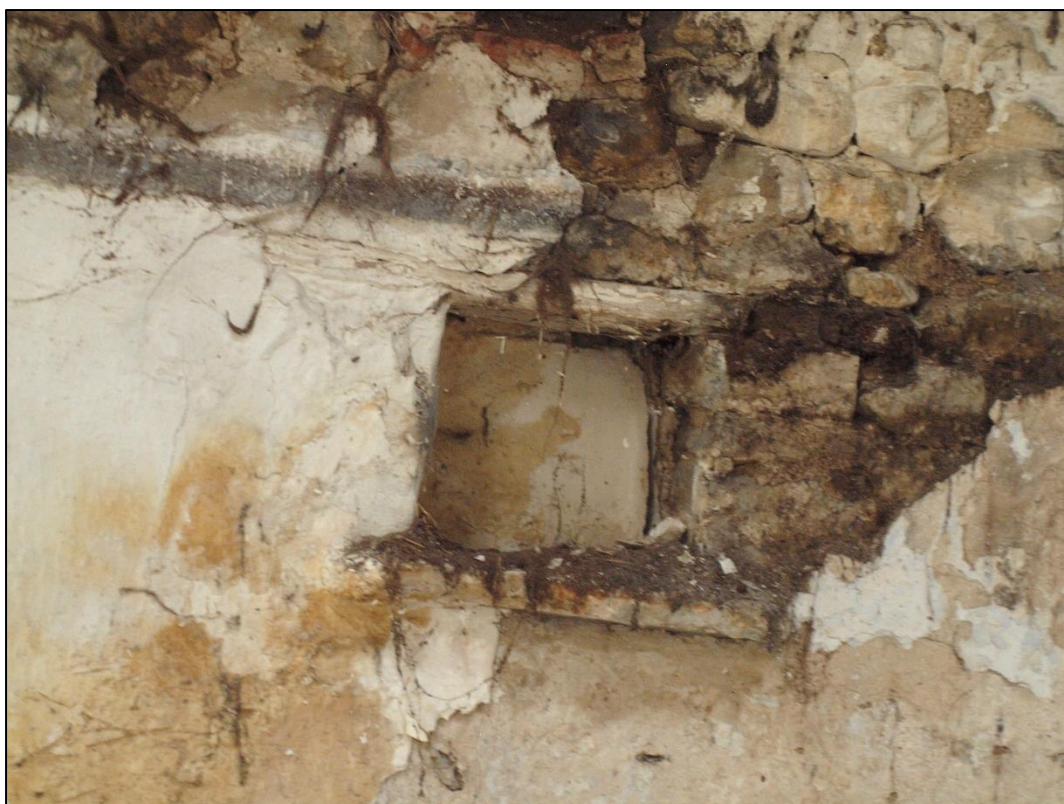
Plate 48: Detail of niche
