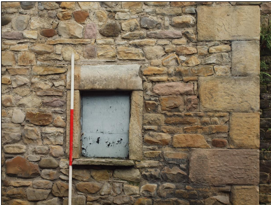
Plate 8: Window to east end detail
