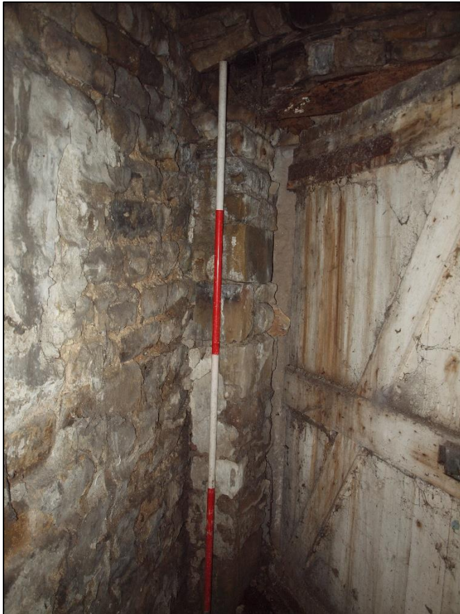
Plate 67: Doorway to outshut
