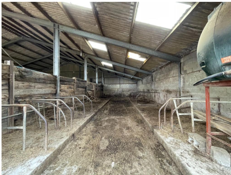
4. Infill between columns longitudinally – timber sleepers and blockwork
