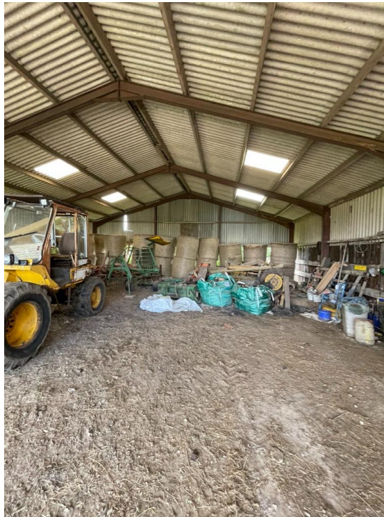
3. Portal frame – unfinished ground
