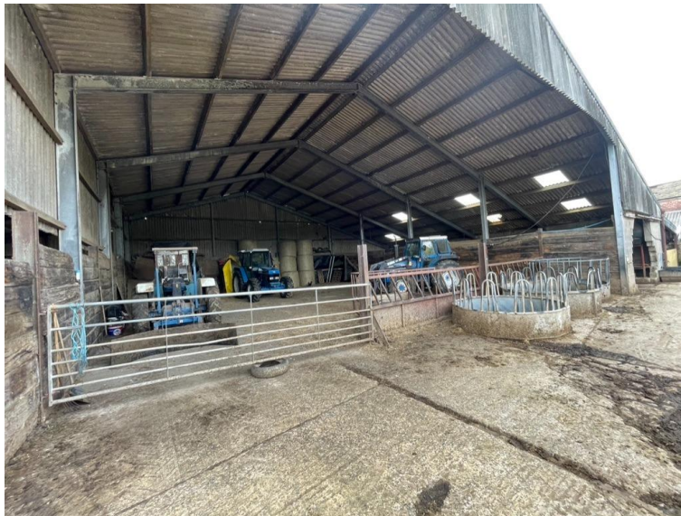
1. Portal frames – concrete hardstanding, timber purlins, 4 bays
