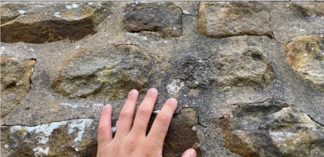
Plate 9: Mortar was generally intact, and no evidence of bat activity was found on the external walls (05/08/2022).
