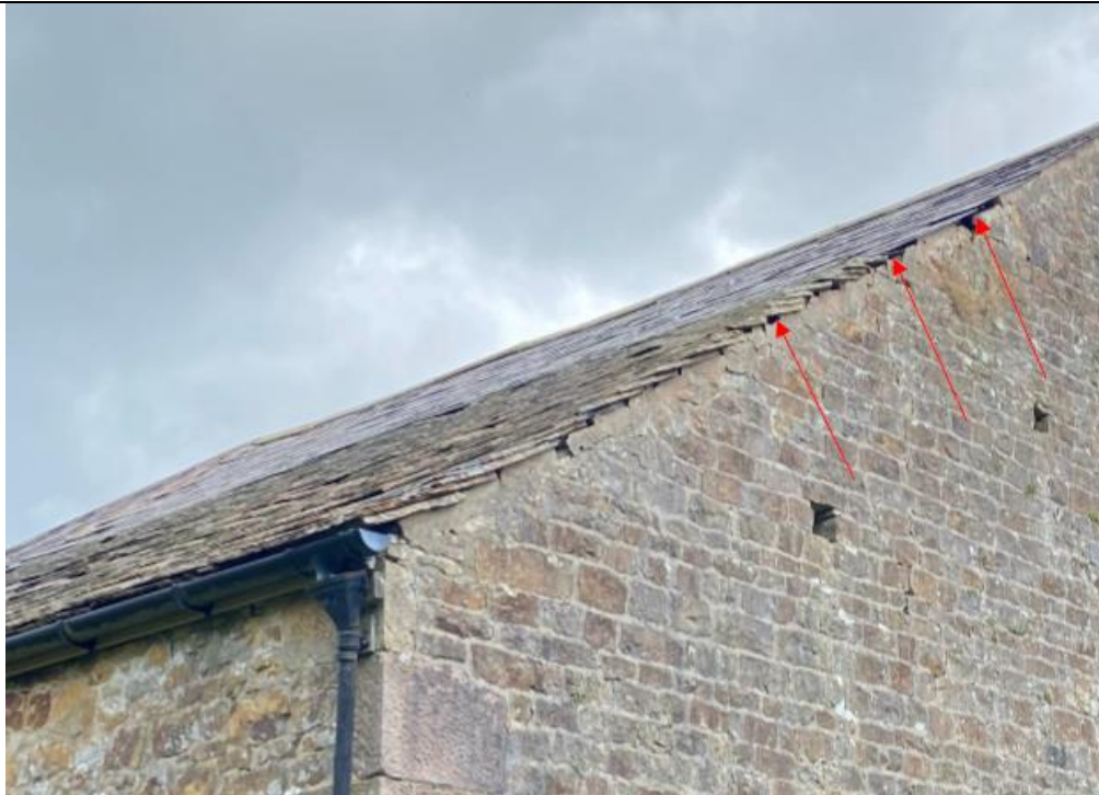
Figure 2: Gaps will be re-incorporated along the verges to replace roosts like-for-like and ensure no loss of roosts.
