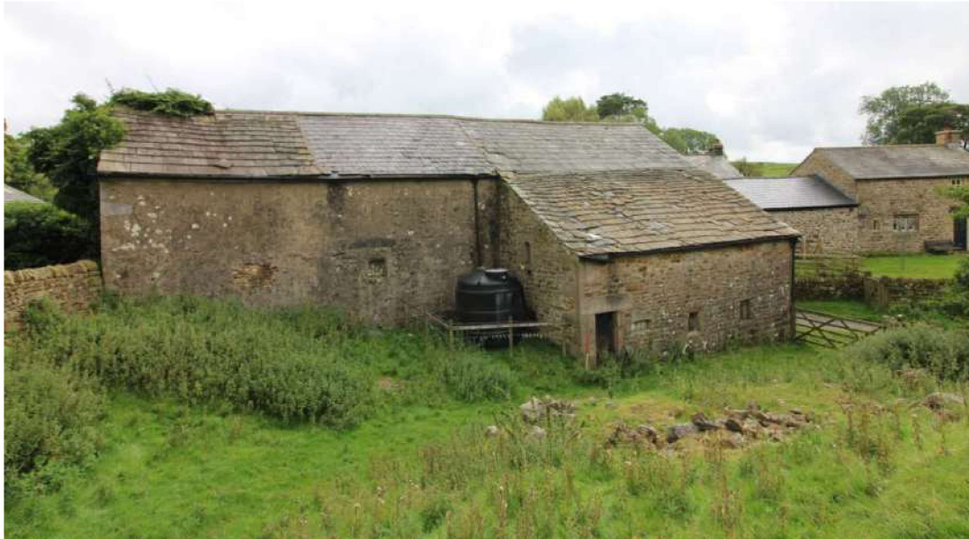
Plate 13: Western elevation (rear). 1m scale
