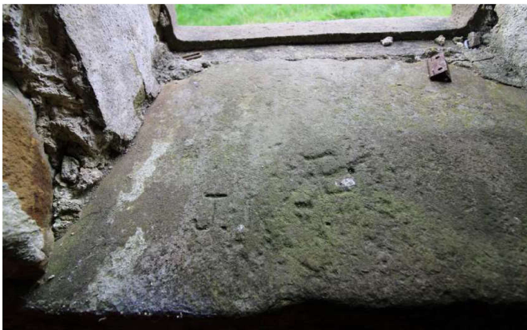
Plate 65: Graffiti on byre window sill (western elevation)
