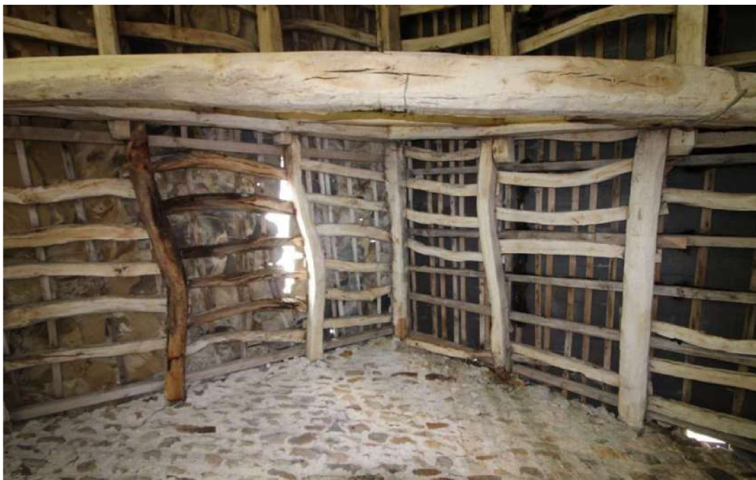
Plate 44: Underside of timber-framed roof showing damage at the southern end of the northern cell
