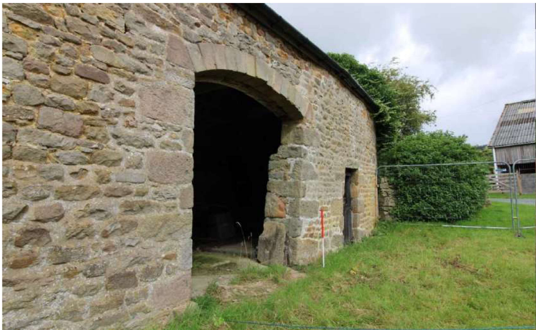
Plate 4: Southern cell butted against the southern gable wall of the northern cell with quoins incorporated into the northern jamb of the southern double width door. 1m scale
