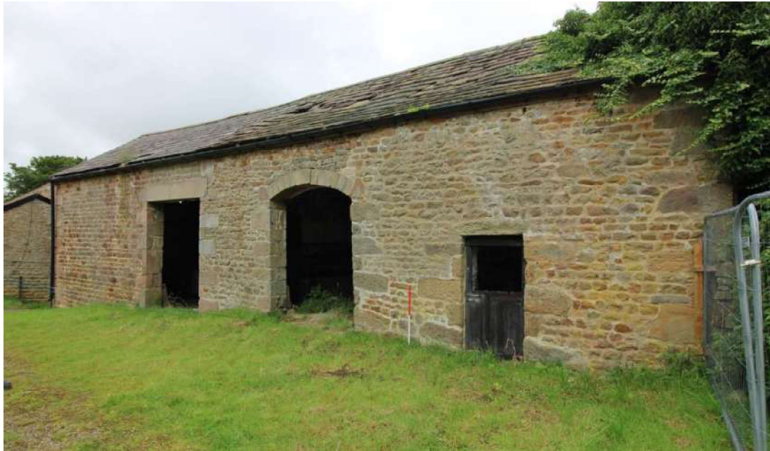
Plate 1: Principal elevation facing south-west. 1m scale
