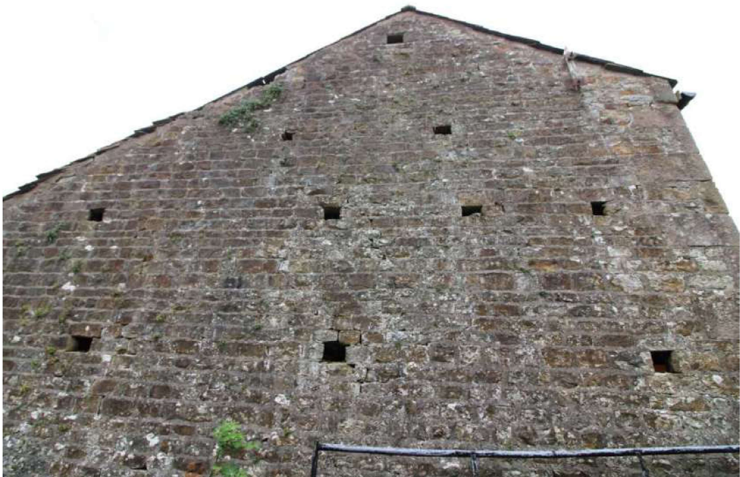
Plate 12: Rectangular apertures and an owl hole on the southern gable wall
