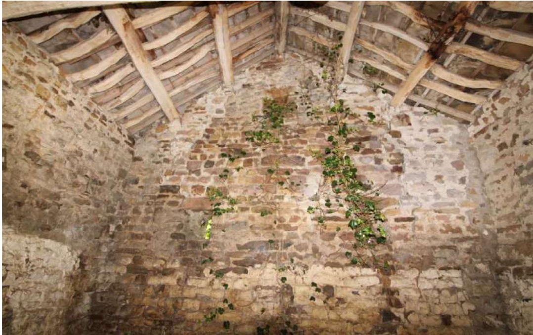
Plate 41: Upper northern gable containing three ventilation loops (northern cell)
