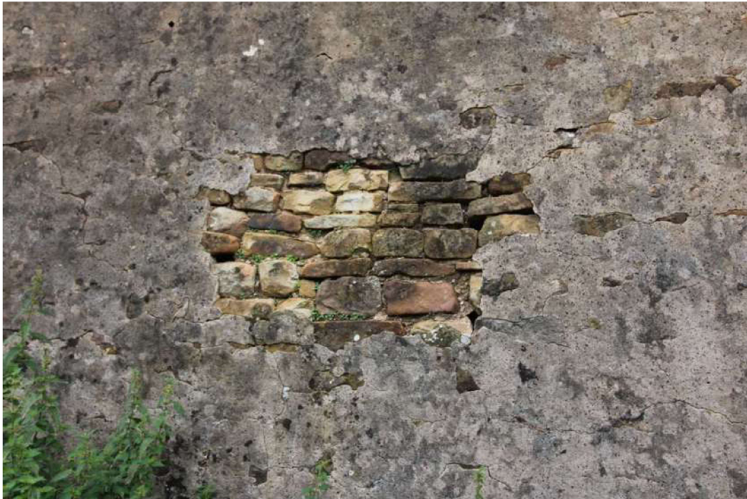
Plate 25: Exposed sandstone rubble at the northern end of the western elevation
