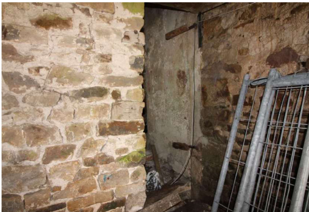
Plate 54: Entrance to western room with remains of door hinges (southern cell)
