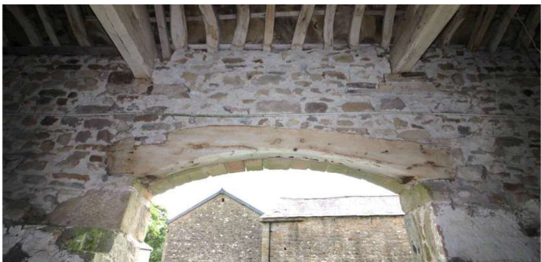
Plate 30: Wooden lintel above double-width door
