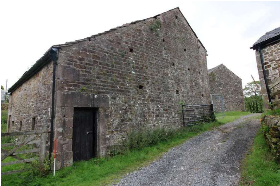
Plate 9: Southern gable end with lean-to lofted byre. 1m scale
