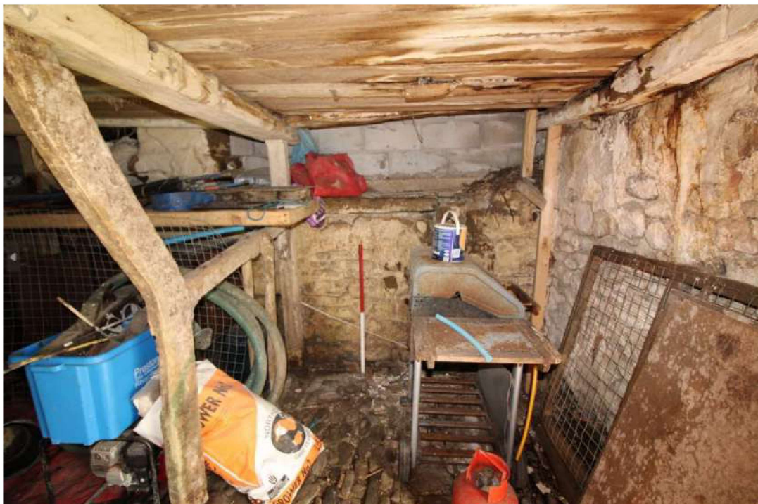
Plate 61: Eastern elevation of a cattle stall with cobbled surface. 1m scale
