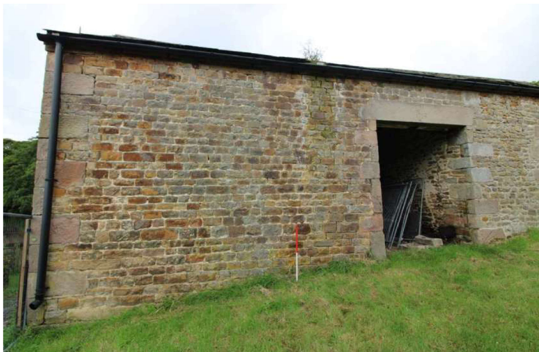
Plate 7: Southern end of southern cell facing west. 1m scale
