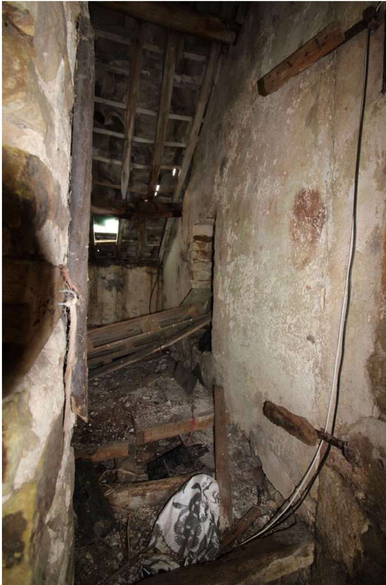
Plate 55: View inside small storage room looking west (southern cell, western side)
