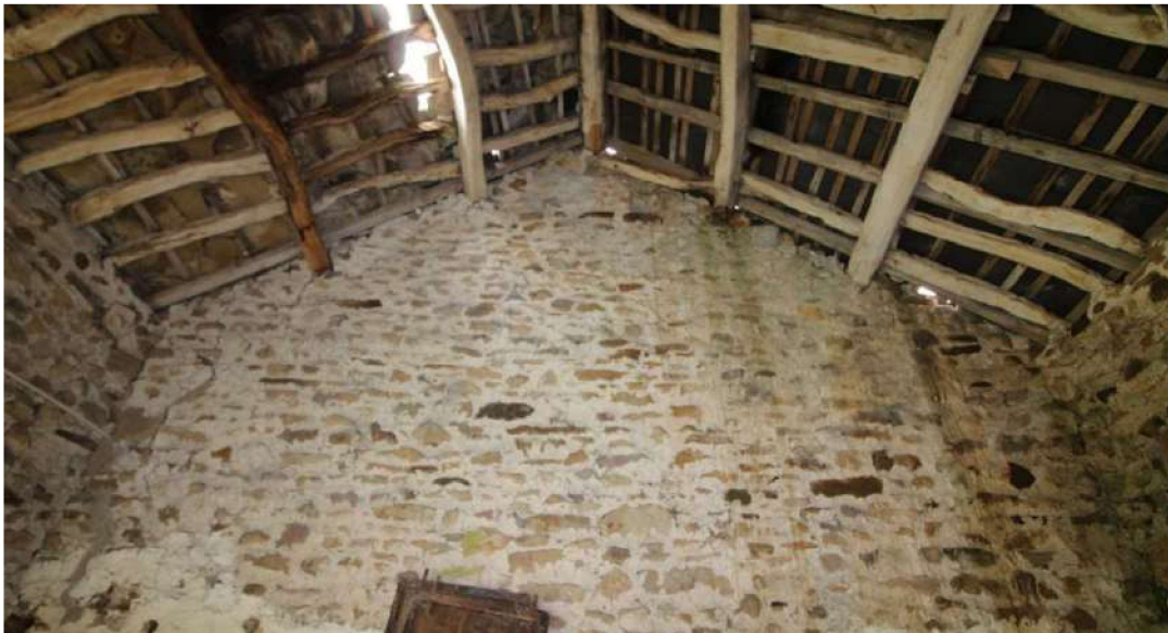
Plate 35: Upper southern gable end (northern cell)
