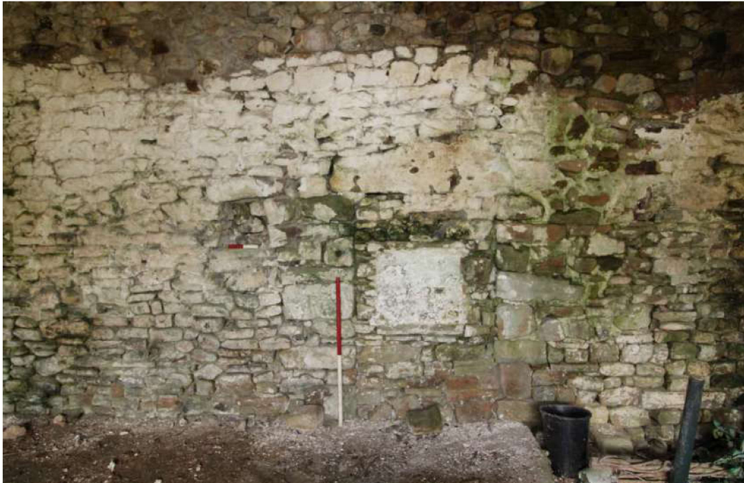
Plate 37: Blocked pedestrian-width door (1m scale) and niche (0.2m scale) (left) in the centre of the western wall (northern cell)
