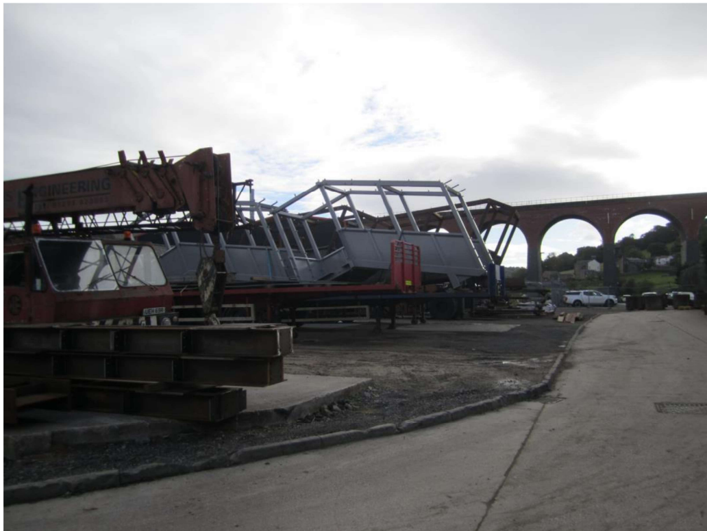
5 Temporary fabrication assembly example.
