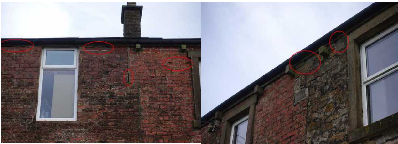
Gaps in pointing and behind fascia board at wall top on frontage.
