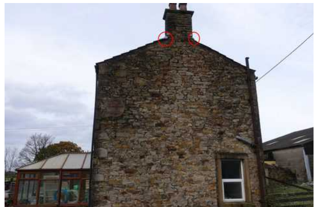
Gaps behind flashing on southern gable
