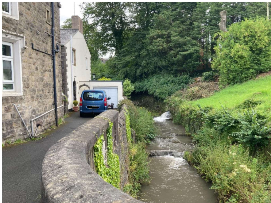
Chatburn (Heys) Brook in deep channel (as seen from the Bridge)
