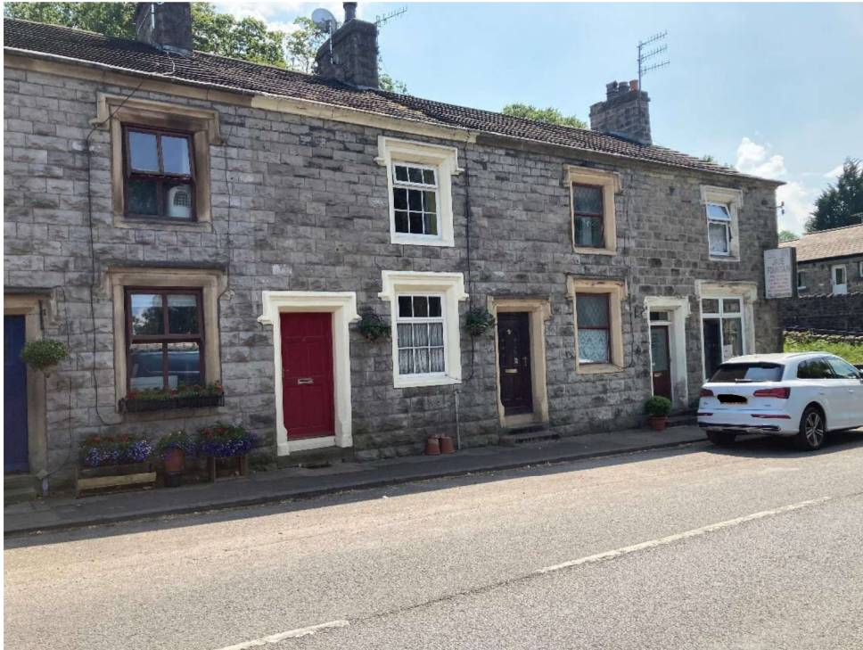
No 10 (second from right) with raised front entrance
