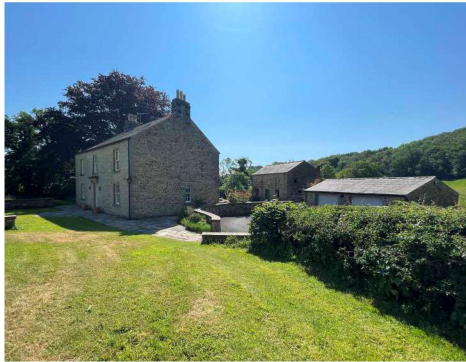
View along original driveway.
