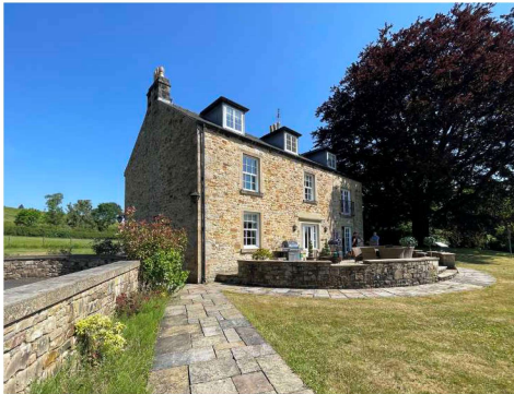
Rear elevation and patio area.
