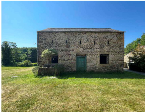
North elevation of barn.
