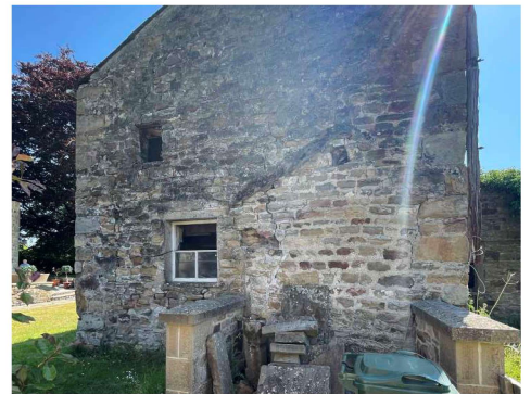
West elevation of barn.
