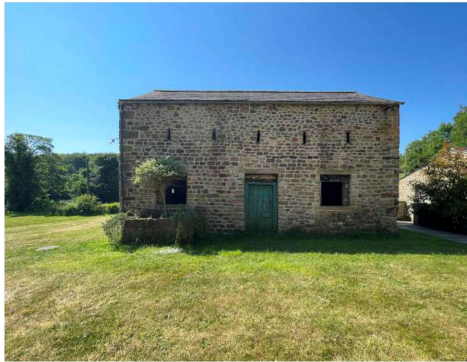
North elevation of barn.
