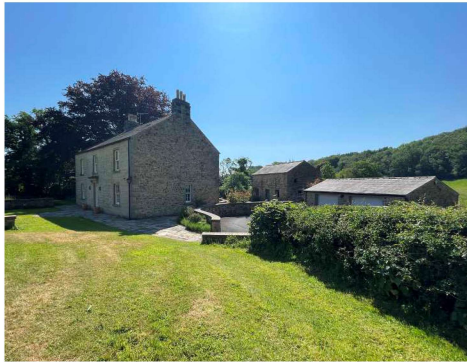
View along original driveway.
