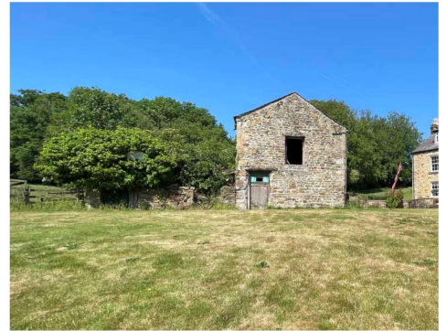
East elevation of barn.
