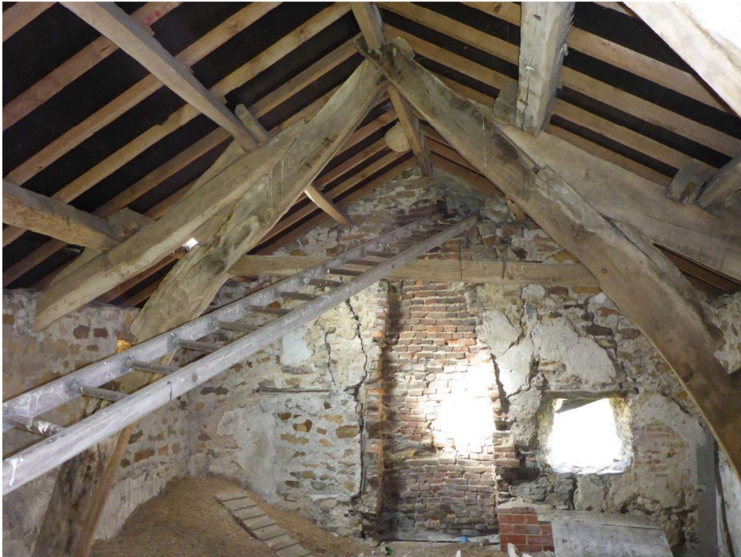
Photo 37 – Original and replacement purlins supported from upper cruck
