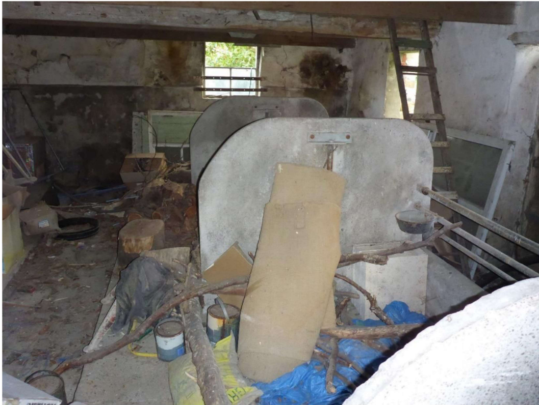
Photo 27 – Internal layout of barn at ground floor level
