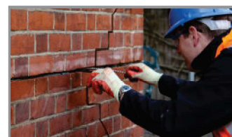
4. Using the HeliBar Insertion Tool push one HeliBar into the grout to obtain good coverage
