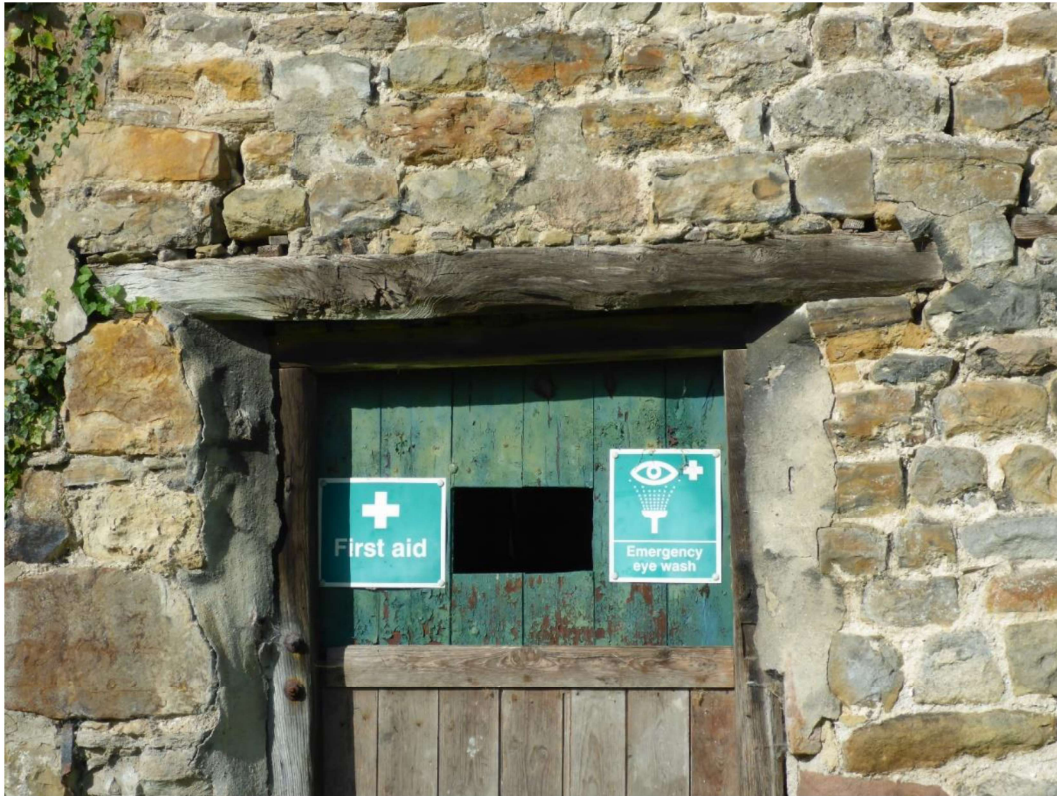
Photo 10 – Timber lintel over doorway
