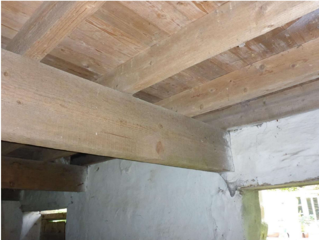
Photo 29 – Sawn timber structure for first floor
