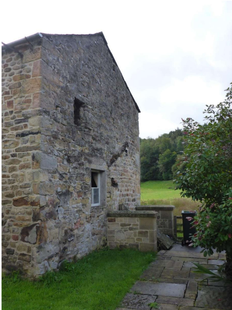
Photo 11 – Western elevation of barn
