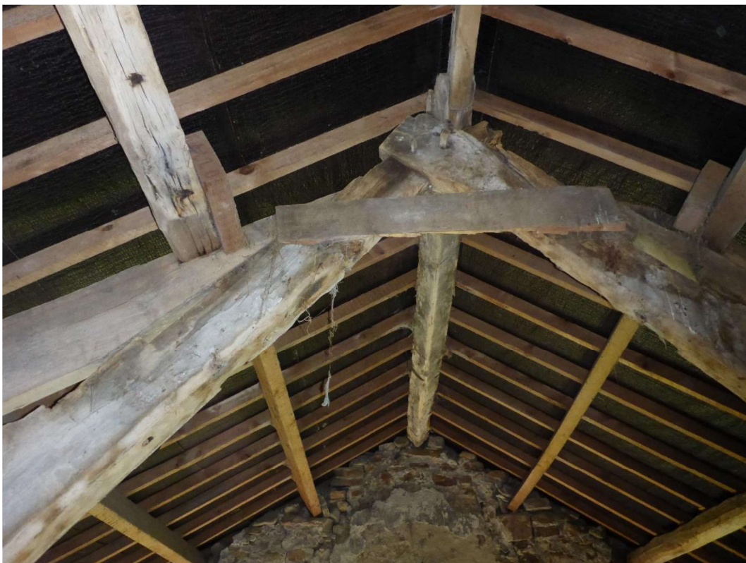
Photo 36 – Replacement tie on upper cruck
