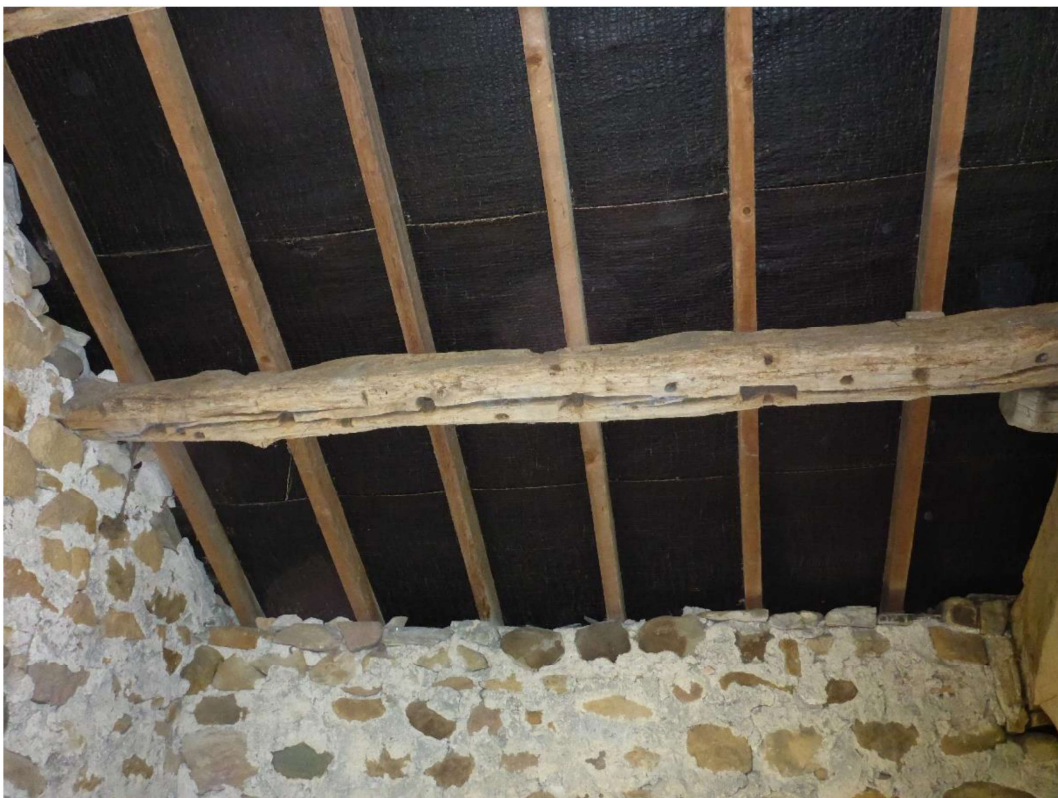
Photo 38 – Condition of original purlins
