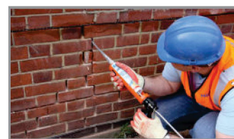
6. Inject CrackBond TE3 into the crack leaving enough space for making it good. Re-point the bed joints with matching mortar and make good the crack.
