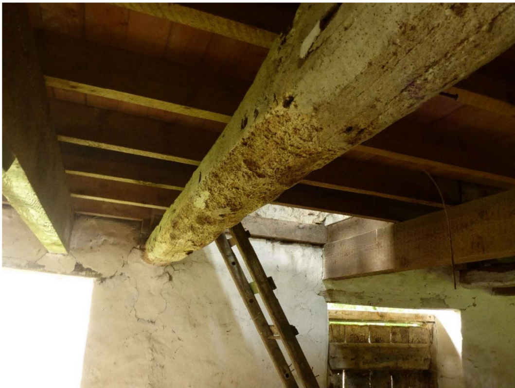
Photo 31 – Sawn timber structure alongside original ceiling ties of upper cruck
