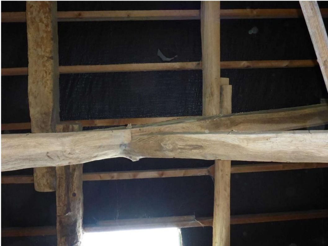
Photo 35 – Possible twist in upper cruck
