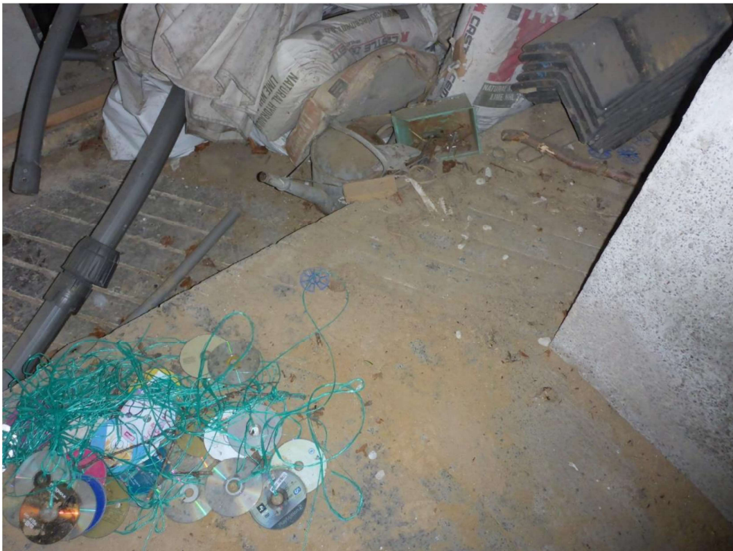
Photo 26 – Concrete floor internally
