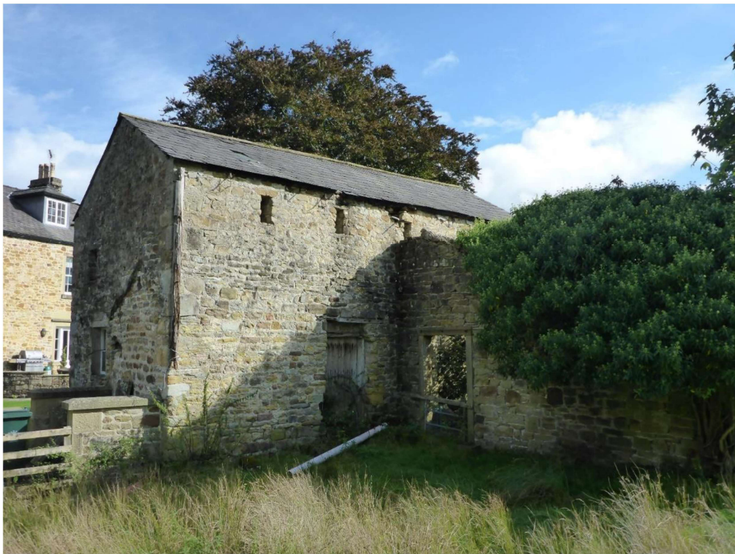
Photo 19 – Rear elevation of barn
