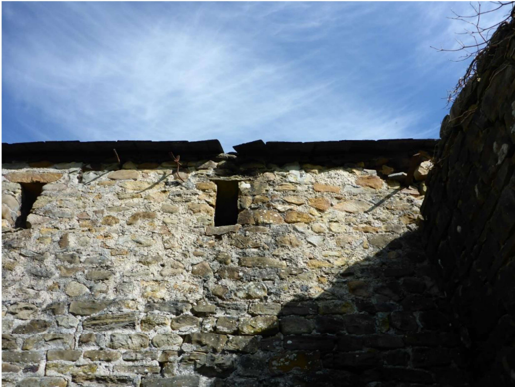
Photo 25 – Slipped roof slate to rear
