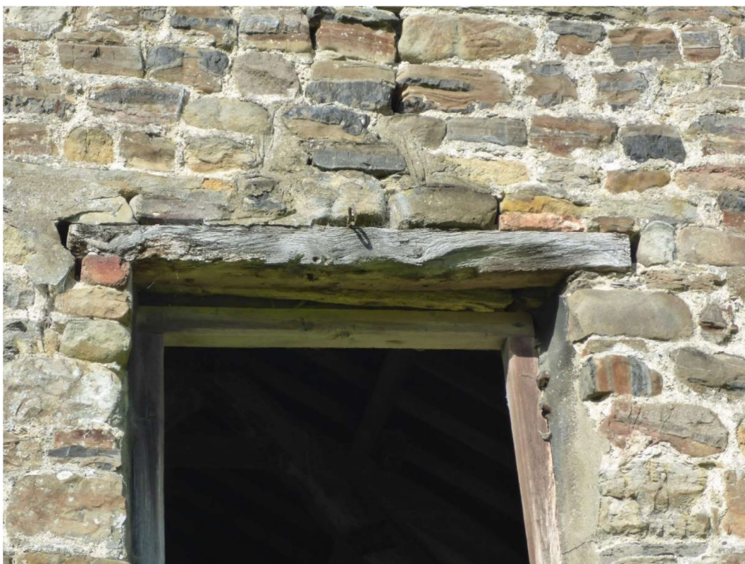
Photo 9 – Timber lintel over hay loft opening
