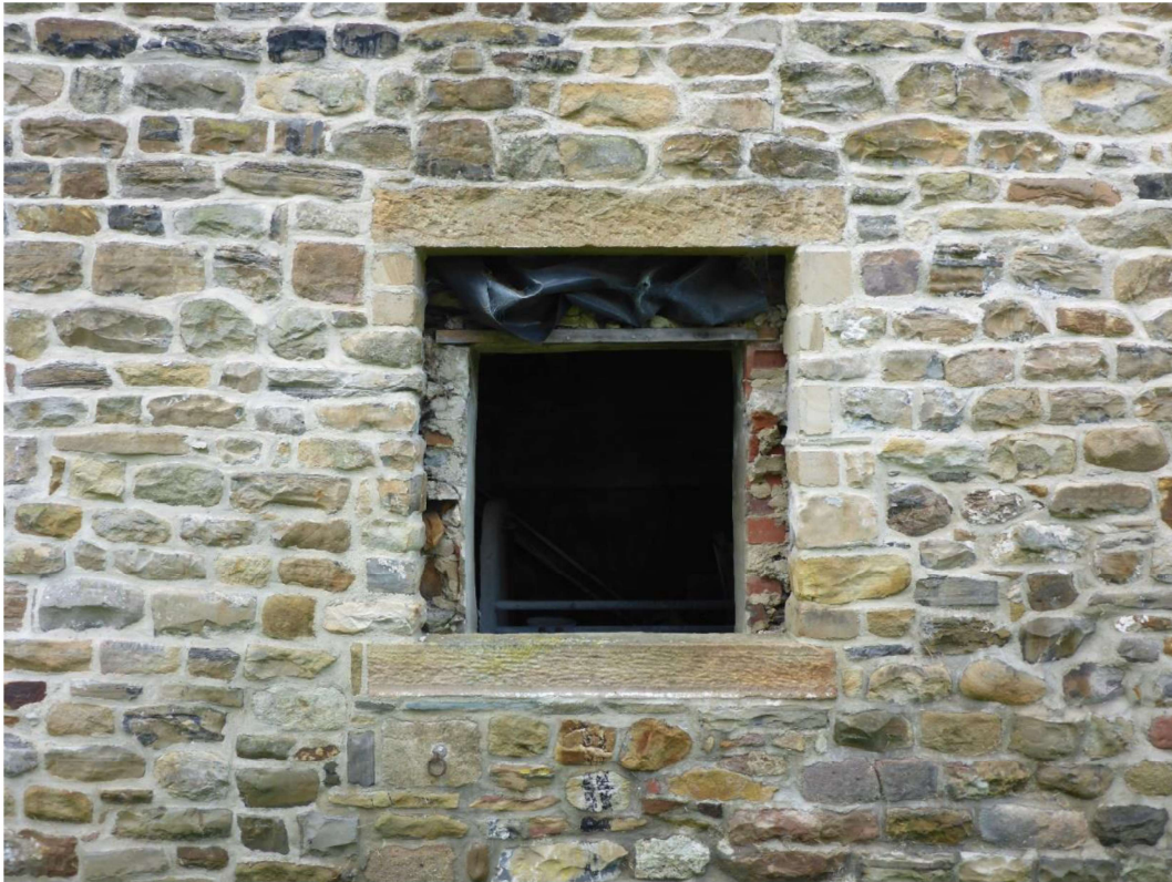
Photo 4 – Stone lintel on front elevation
