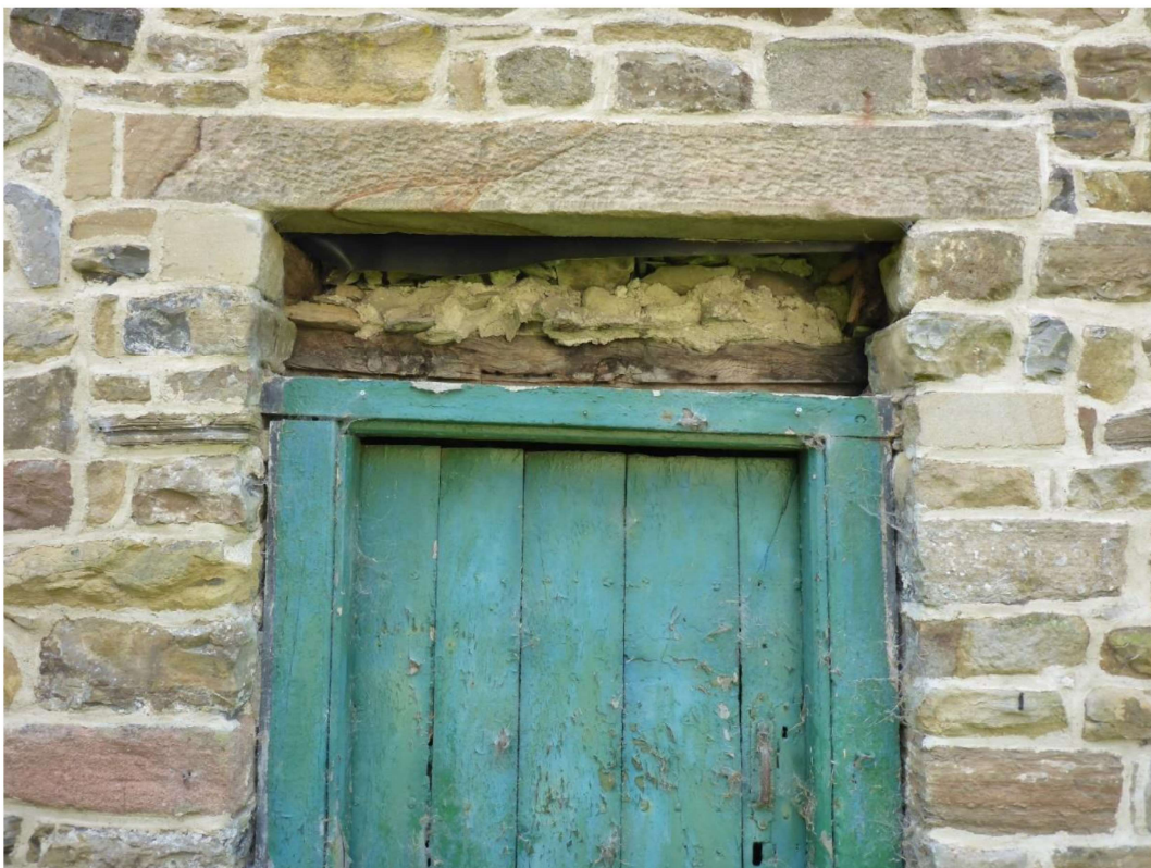
Photo 5 – Stone lintel over door on front elevation
