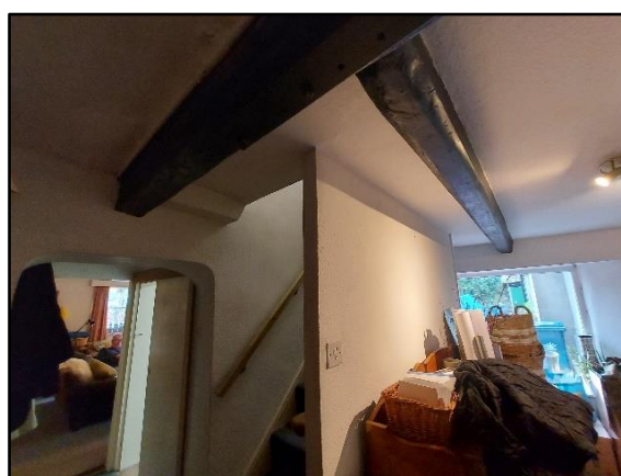
Figure 20 – Timber beams in the (dining) room overlooking the rear garden at 10 Shawbridge Street
