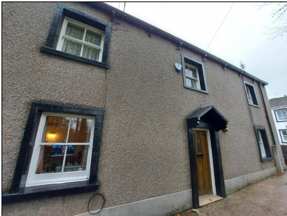
Figure 9 – Eastern elevation (entrance to 10 Shawbridge Street)
