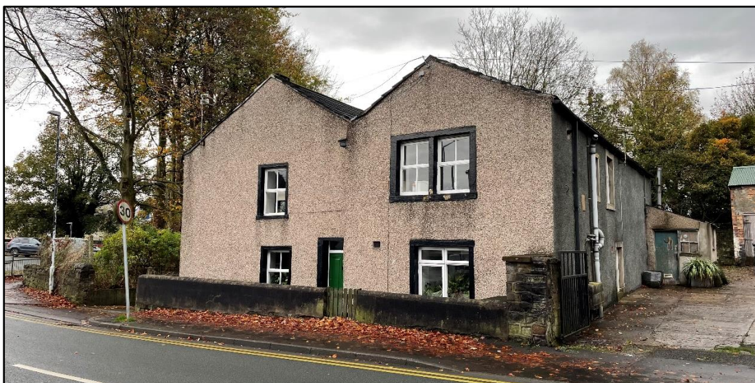
Figure 7 – The building seen from Shawbridge Street
