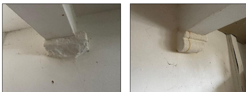
Figure 19 – Stone pads on the ground floor of 8 Shawbridge Street
