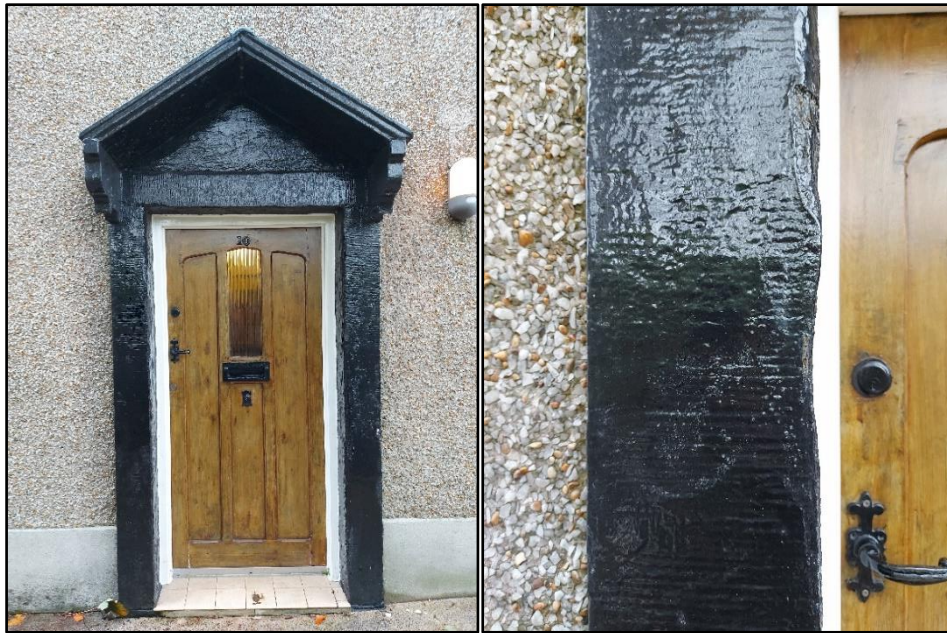
Figure 10 – Doorway with hood (left), detail of tool finish on stone surround (right)
