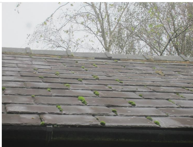
Photo 8: Slate roof over utility area with sections of missing bedding mortar beneath the ridge copings
