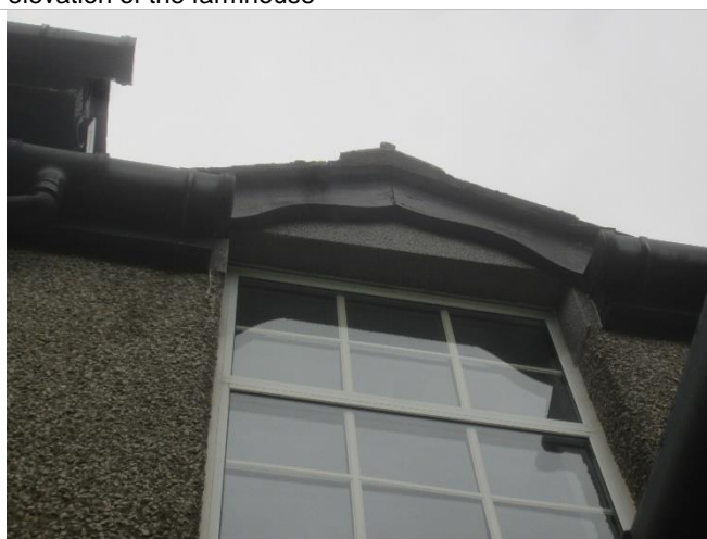
Photo 12: Gaps behind timber fascia at eastern section of farmhouse
