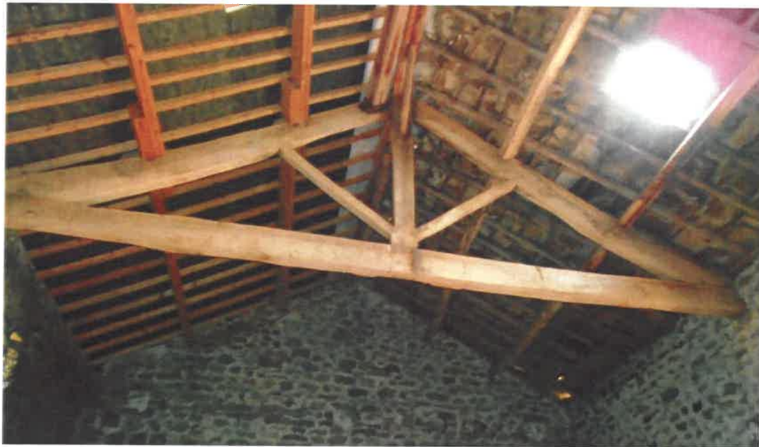
Photograph (– Showing the roof structure to the main barn.
