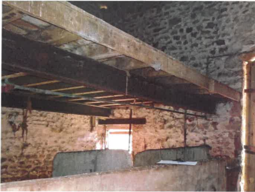
Photograph– Illustrating the condition of the internal front wall.
