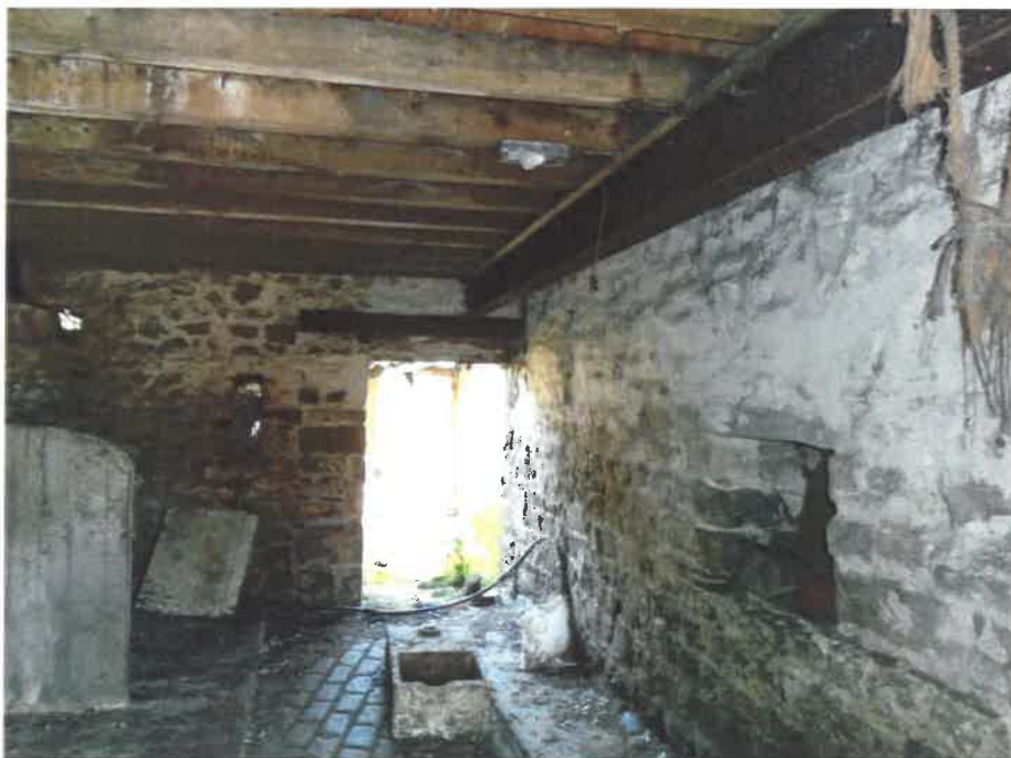
Photograph– Illustrating the condition of the internal rear wall.
