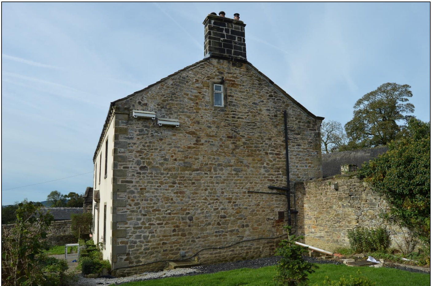
PL07: View of the east gable end of Eaves House Farmhouse.
