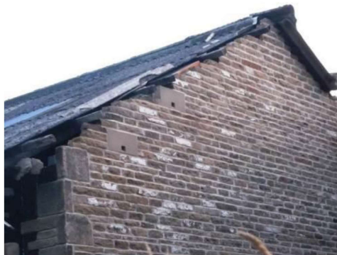
Example of Forticrete boxes in situ
