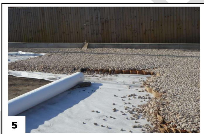
Photo 5: A closer view of the GeoWeb™ surface showing the cells filled with road stone and the geotextile membrane base layer.
