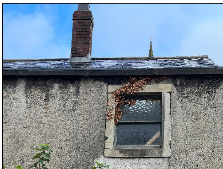
Photo 4: Southeast facing gable end with dense ivy coverage, recently mortared ridge tiles and lead work to chimney.
