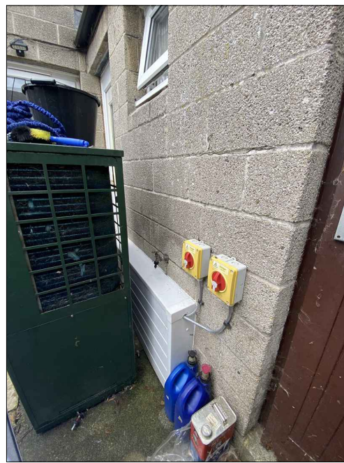
Photos of ASHP as Existing Note: Timber enclosure around air source heat pump present at some properties. To be removed prior to EWI works.
