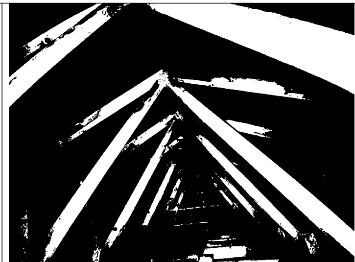
Figure 23 Loft space of B7
