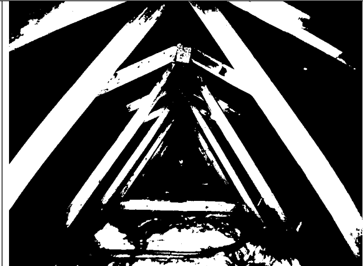
Figure 11 Loft space of B1
