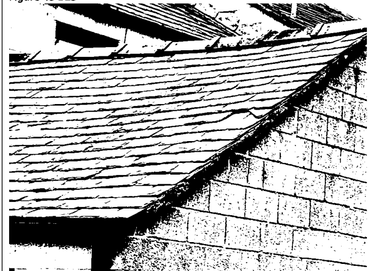
Figure 44 Broken on rear extension of B15
