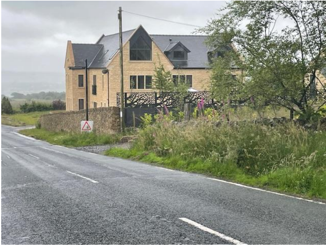
Image 3 Stylised fencing forms the boundary fence of the neighbouring property
