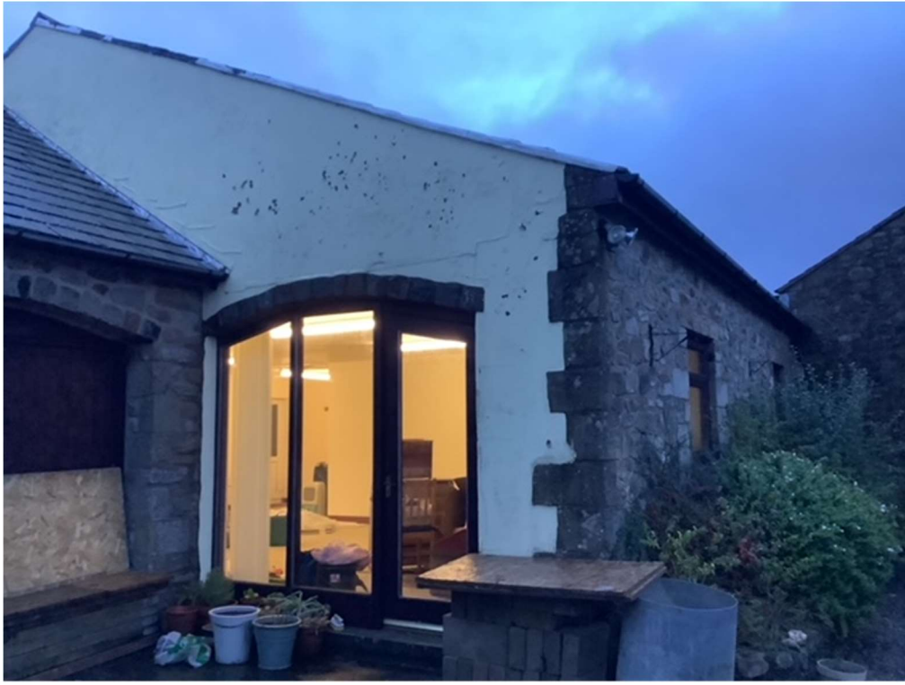
Main entrance to Annex
