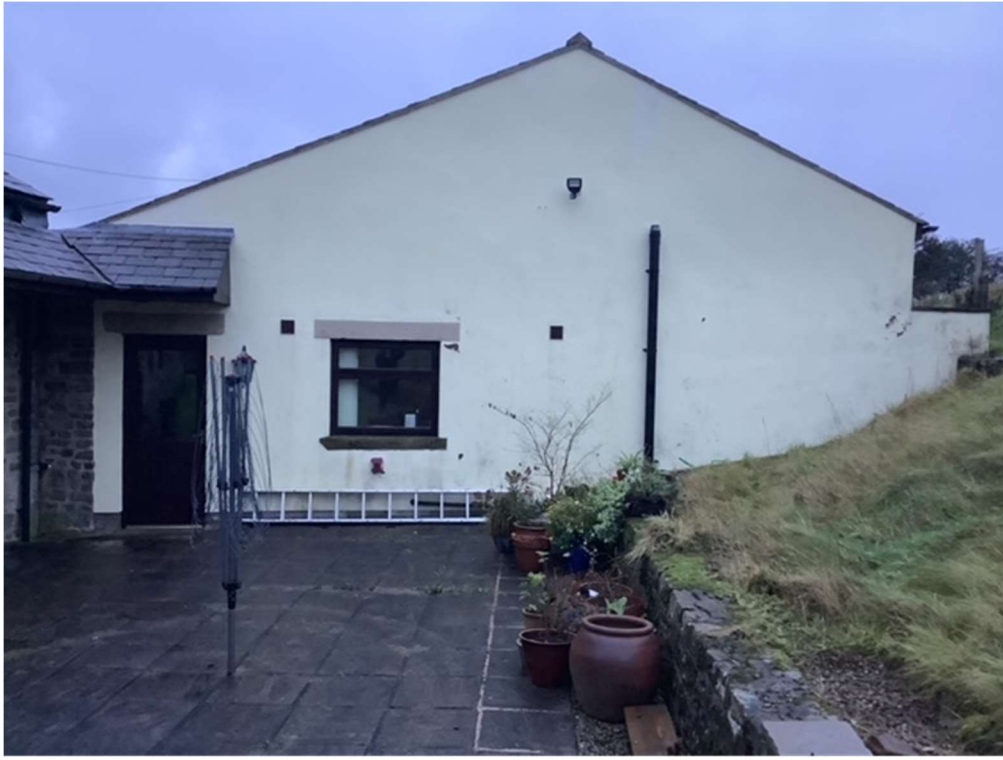
Rear Side of Annex
