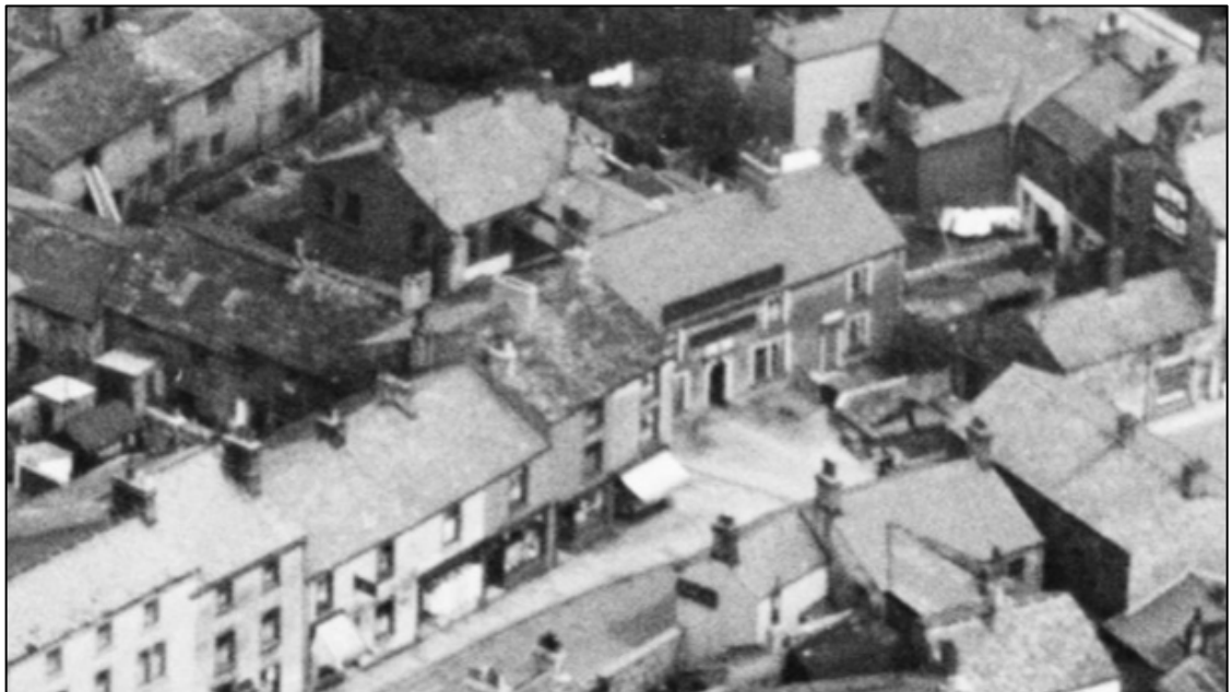
Figure 7 - 1938 aerial showing the front elevation of the Dog and Partridge and No 3 set back from the road, with the 20 th century additions to the rear (Source: Britain from Above).
