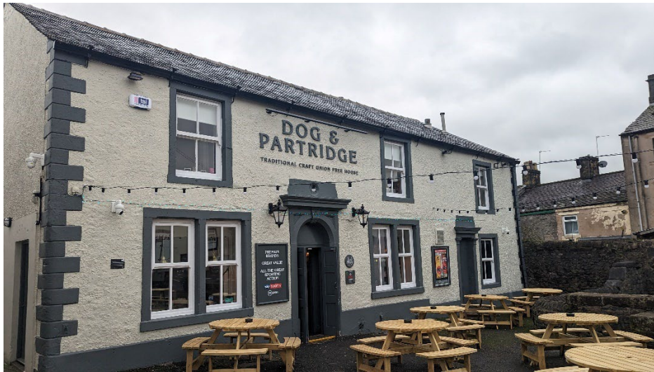
Figure 9 - Front elevation showing pebble-dashed exterior and lack of chimney stacks.
