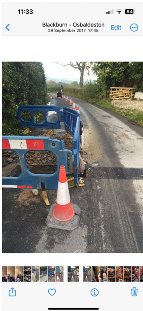
Photo: 29/09/17 to show installation of gas supply to former garage
