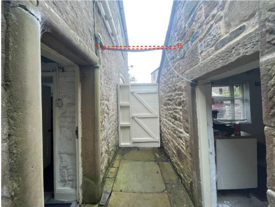
The passage way between the wash-house and the dwelling.
