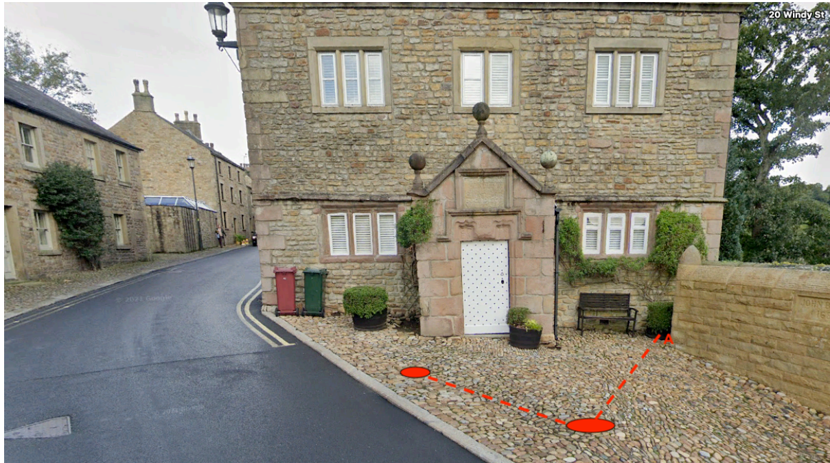
Front curtilage, with an illustration of where the boreholes may be drilled and the underground connecting pipework will enter the building
