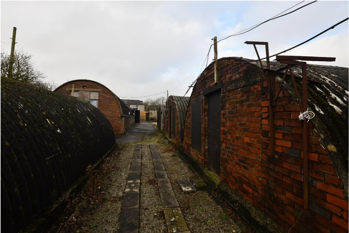
Image 5 Looking north through the various buildings
