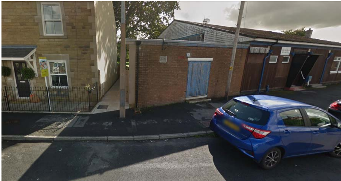
Figure 2.4: Figure 2.5: Front of Existing Building (North-West Face)
