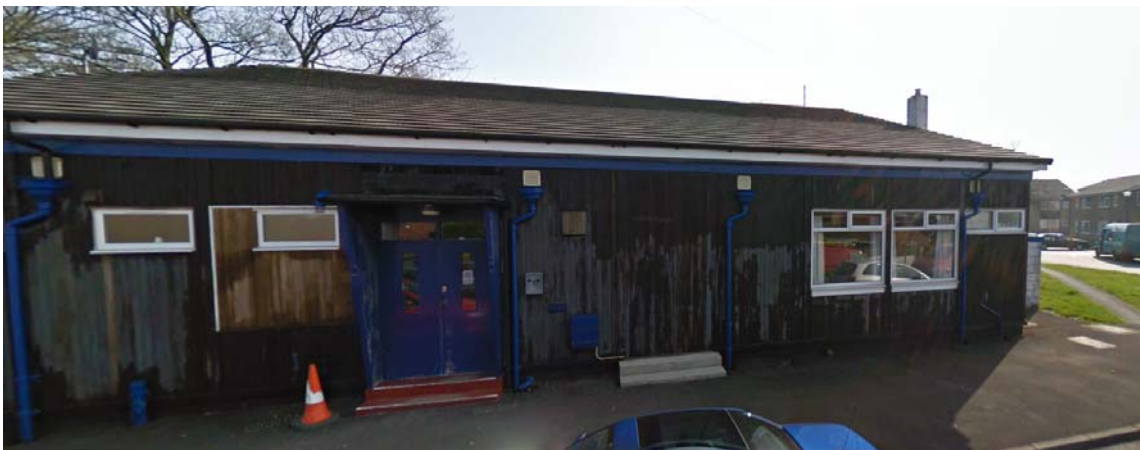
Figure 2.2: Figure 2.3: Front of Existing Building (South-West Face)
