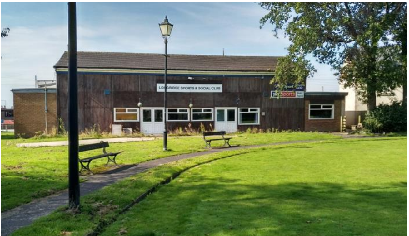
Figure 9) The Club fronting the former bowling green
