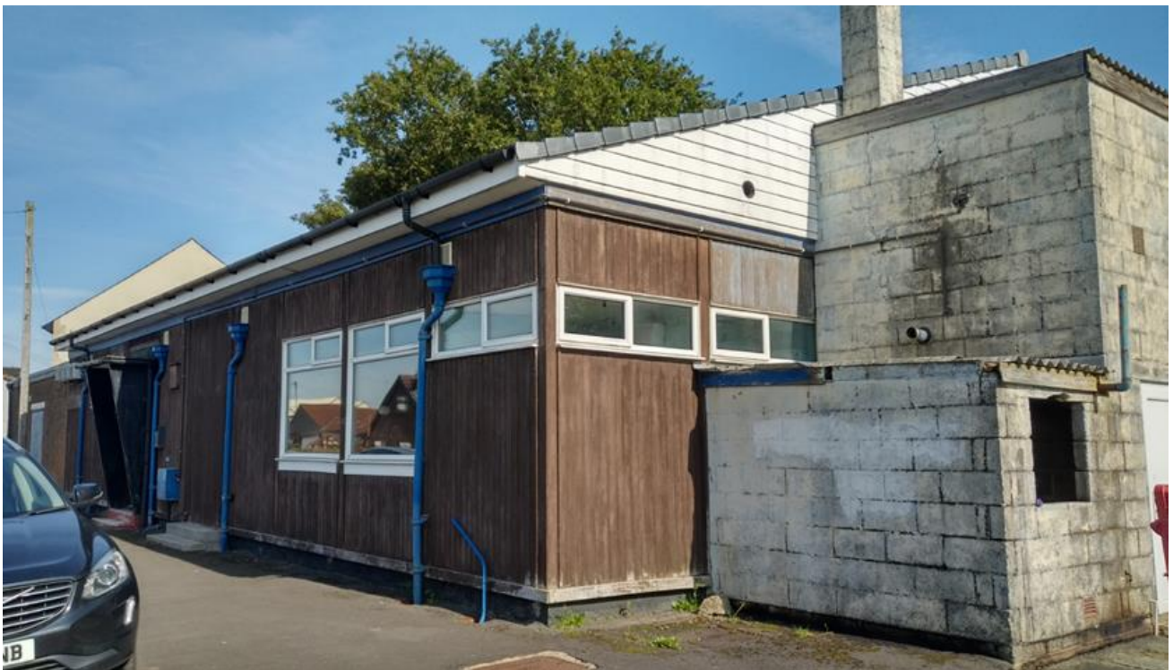
Figure 5) The Club fronting Towneley Road
